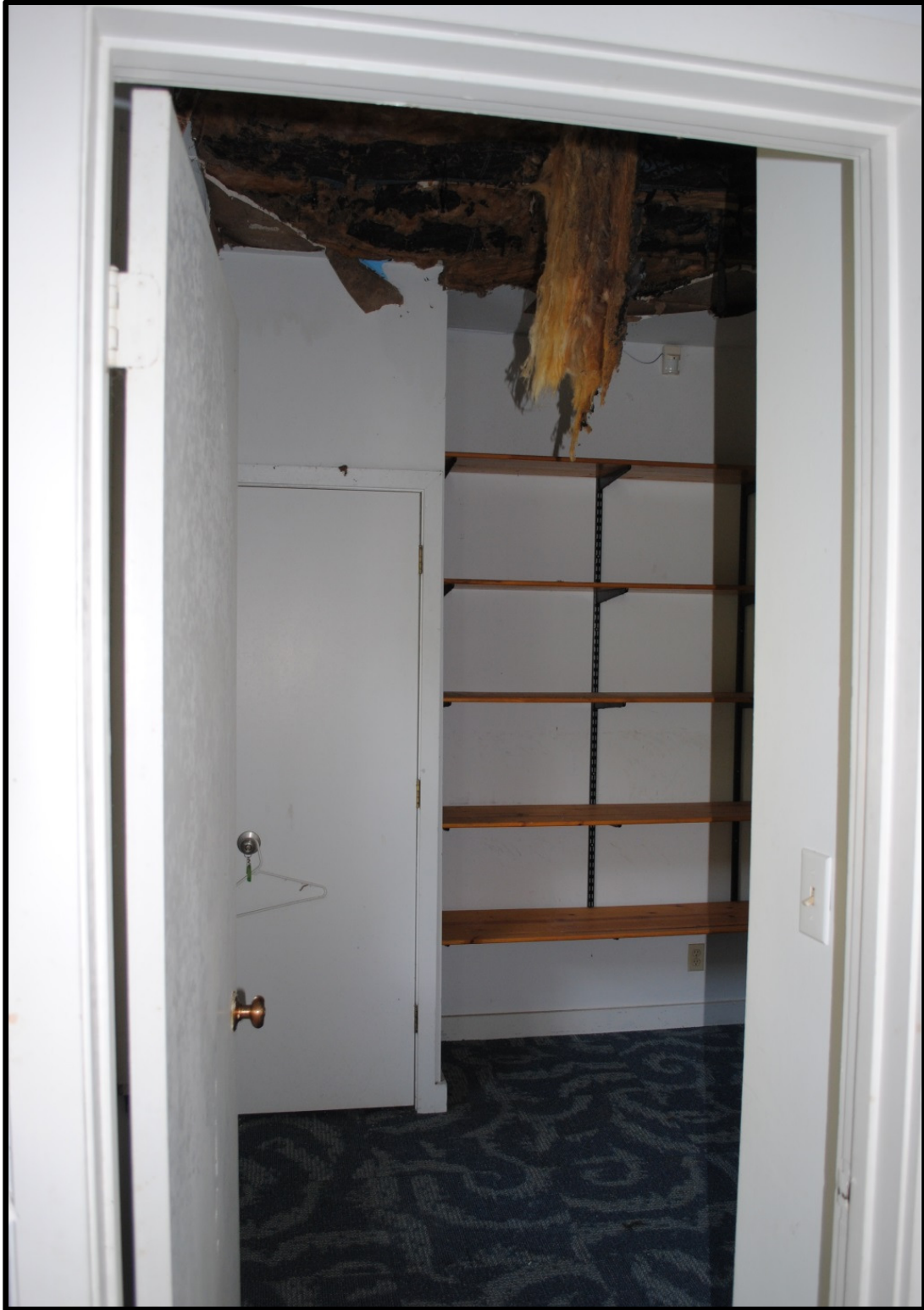
Figure 12 CGMH, auxiliary structure – second floor, looking west (before), 2014
