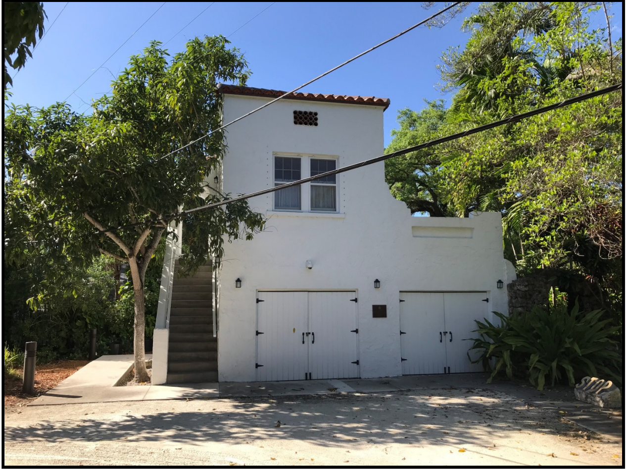
Figure 11 CGMH, auxiliary structure – east / front façade (after), 2019
