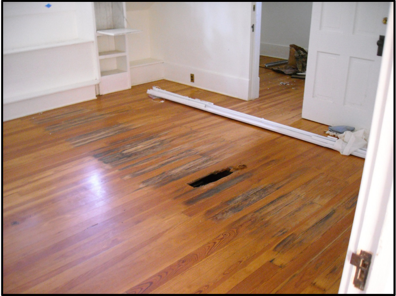
Figure 20 CGMH, second floor west bedroom, looking north (before), 2017
