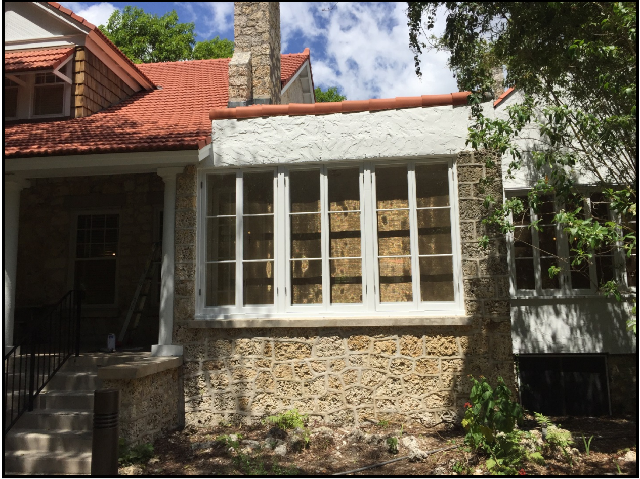
Figure 9 CGMH, east façade at sunroom (after), 2019
