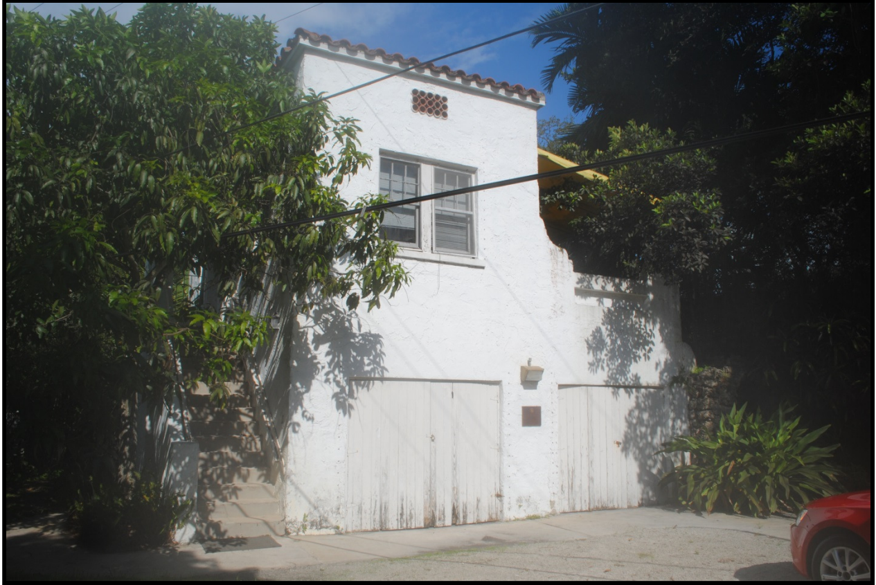
Figure 10 CGMH, auxiliary structure – east / front façade (before), 2014
