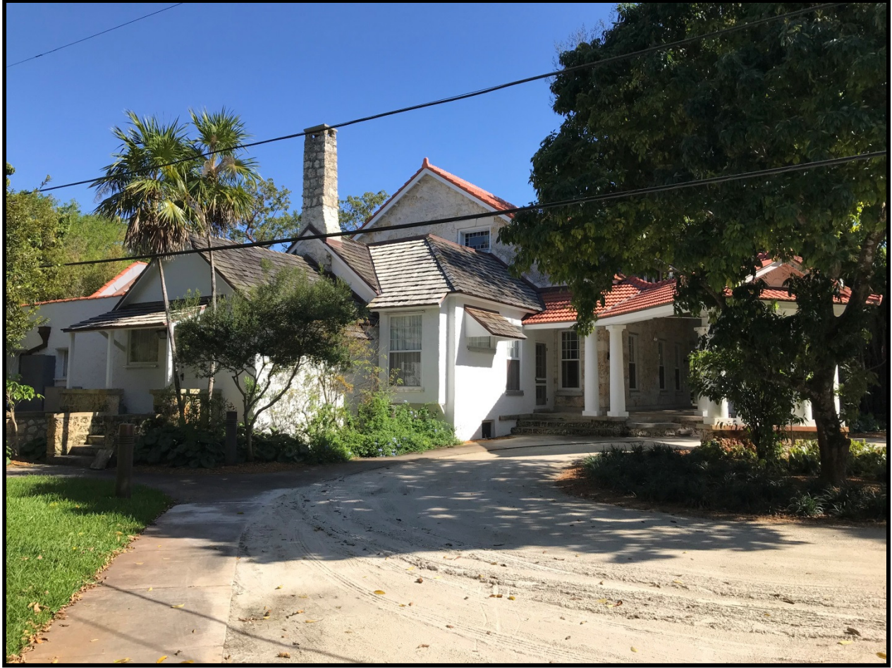
Figure 5 CGMH, northwest corner (after), 2019
