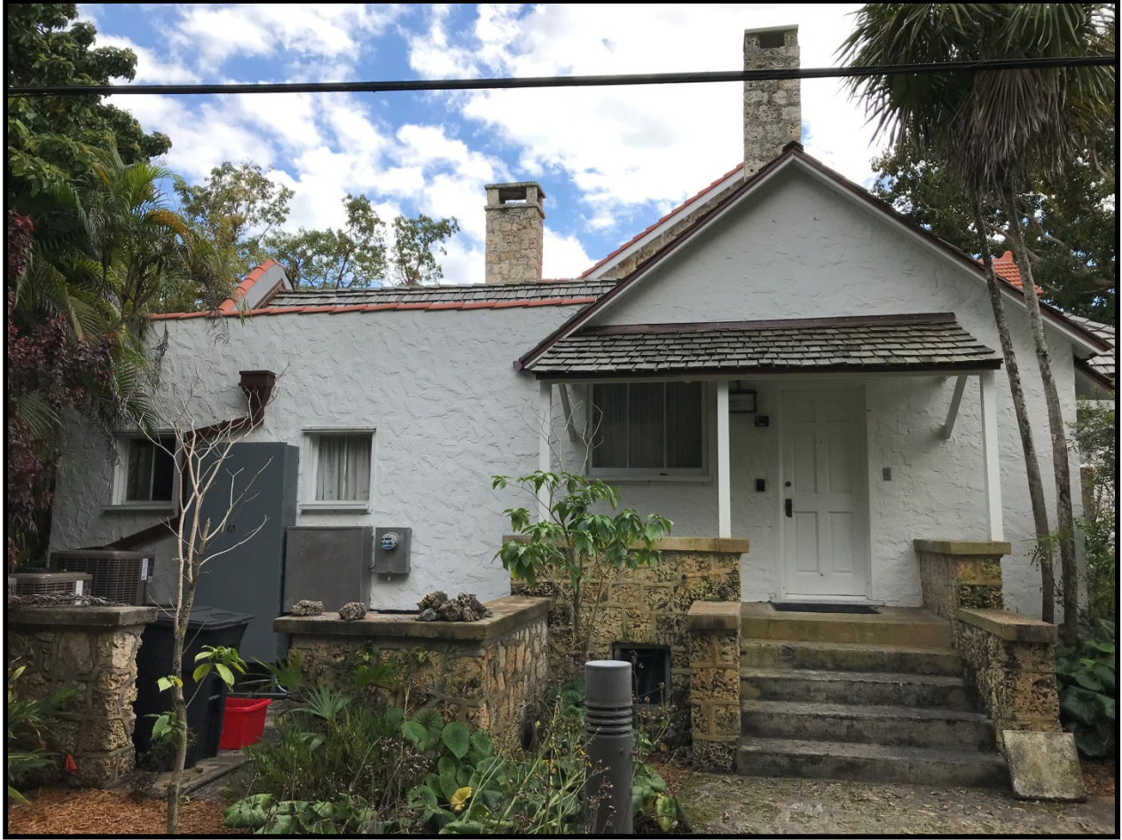
Figure 7 CGMH, north / rear façade (after), 2018
