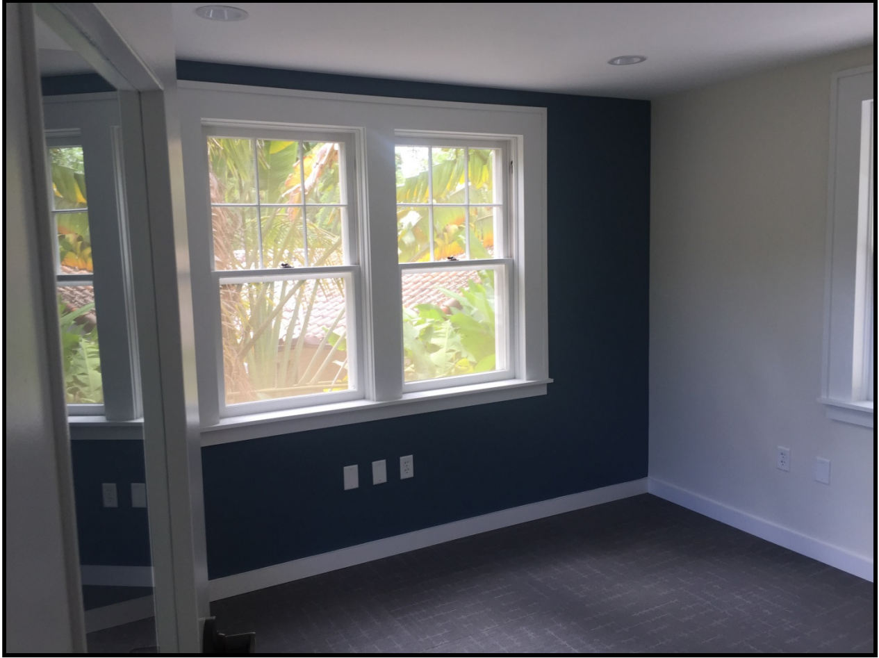
Figure 13 CGMH, auxiliary structure – second floor, looking west (after), 2019
