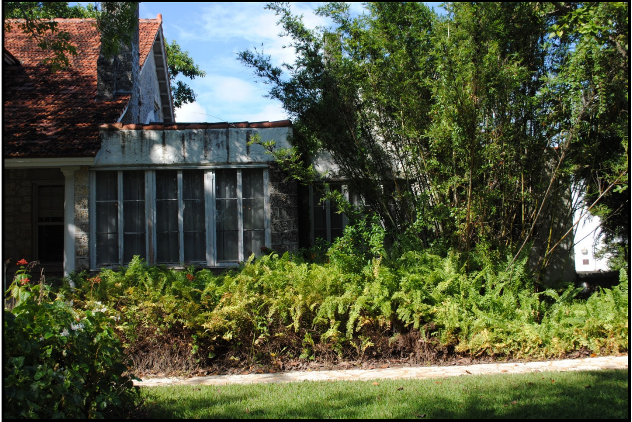
Figure 8 CGMH, east façade at sunroom (before), 2014
