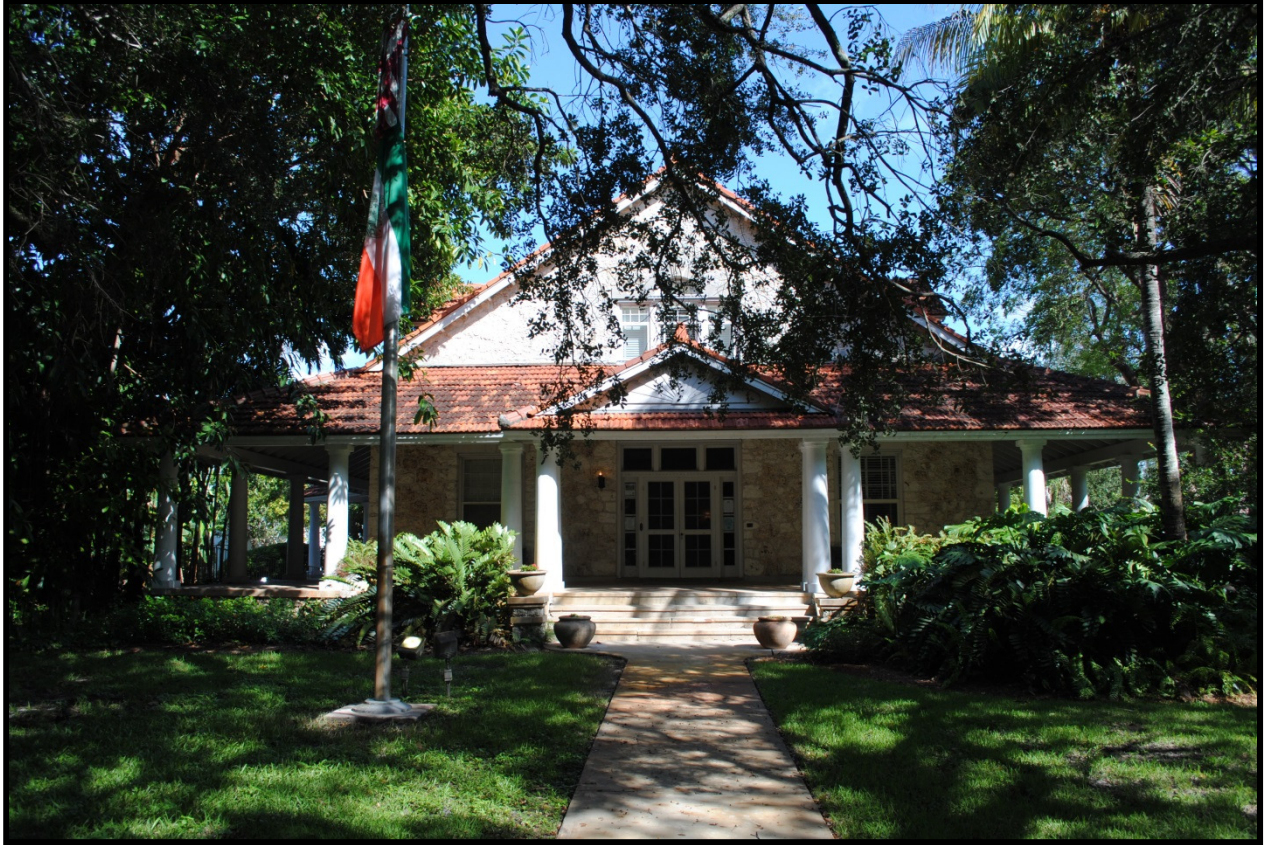
Figure 2 CGMH, south / front façade (before) 2014
