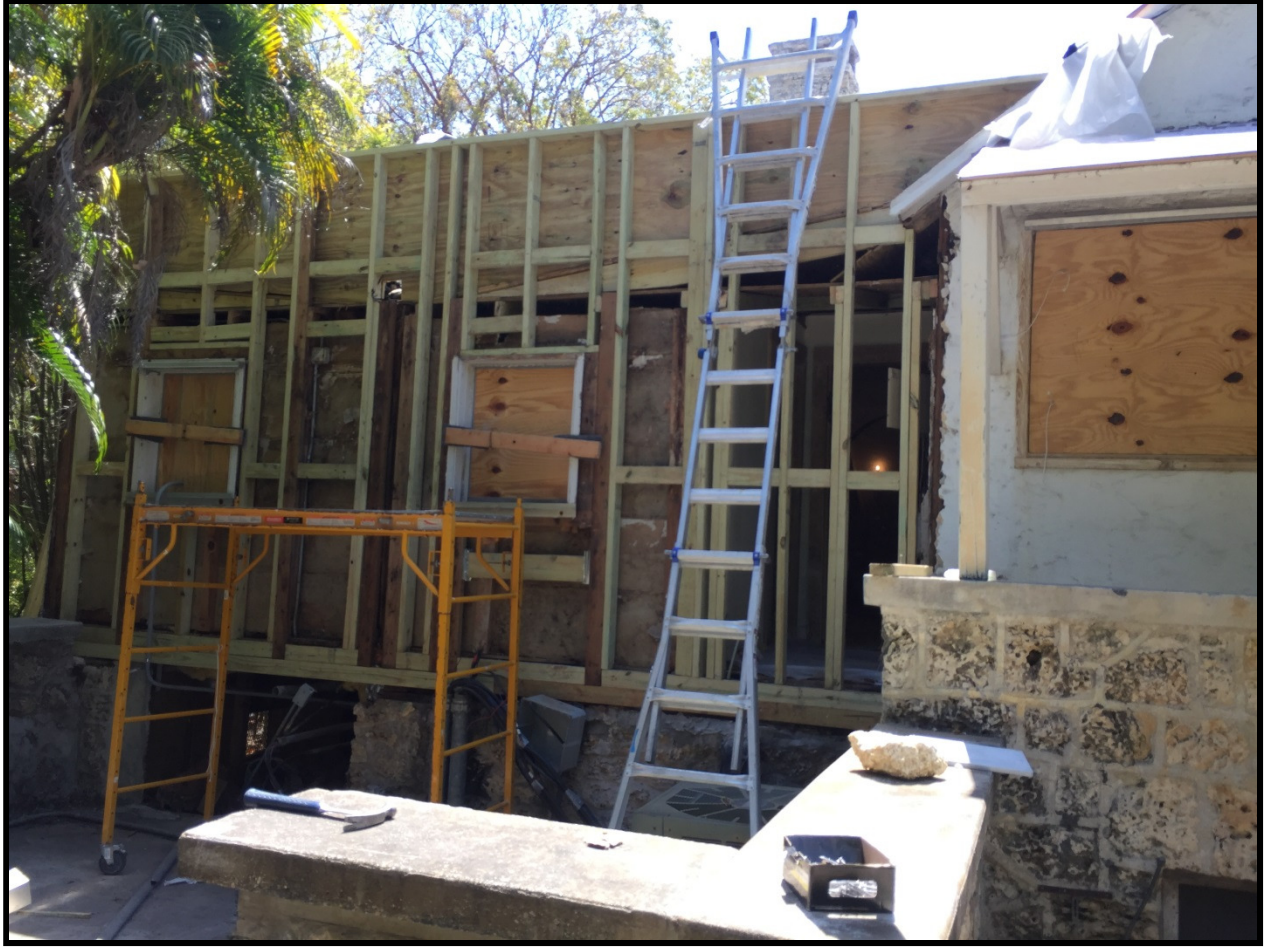
Figure 6a CGMH, north / rear façade (during), 2017
