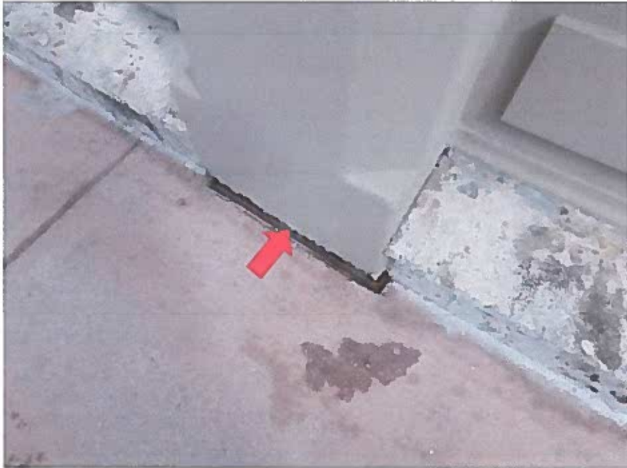
Expansion joint at sidewalk
