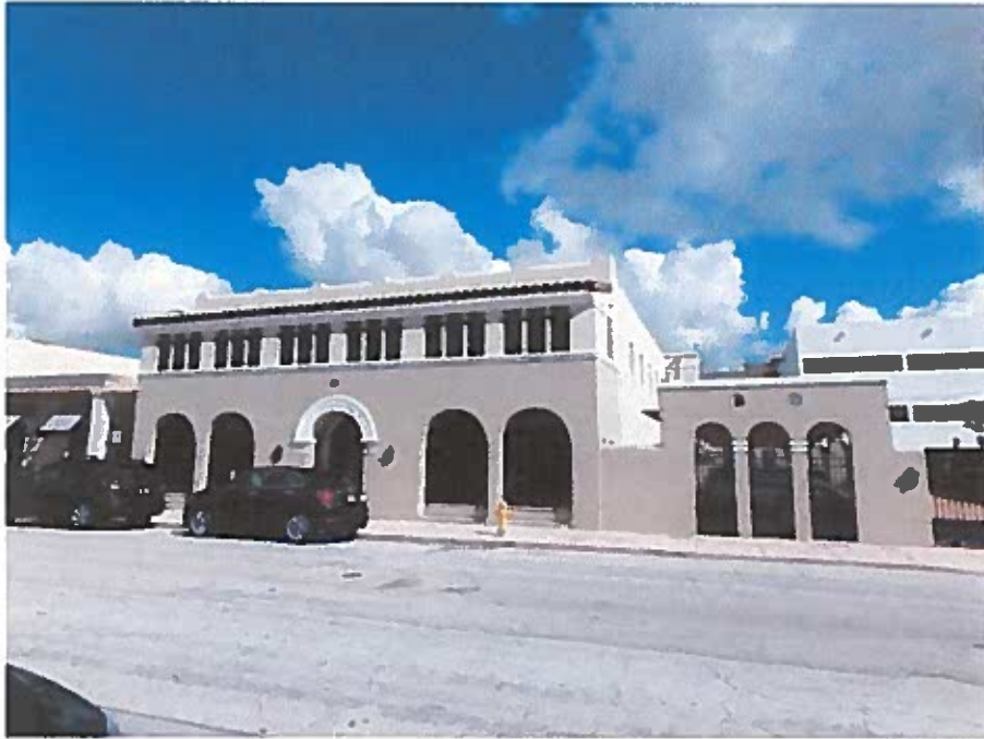
Front of building
