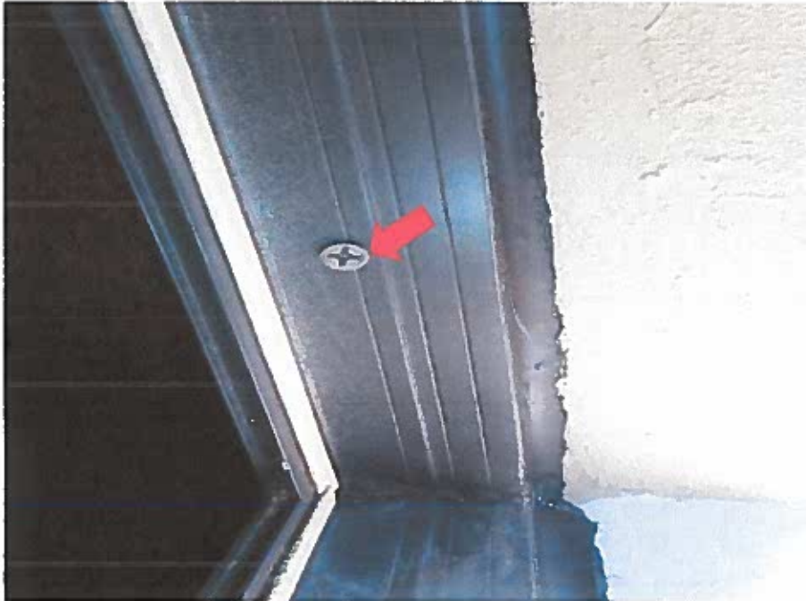
Screw fasteners at window jamb
