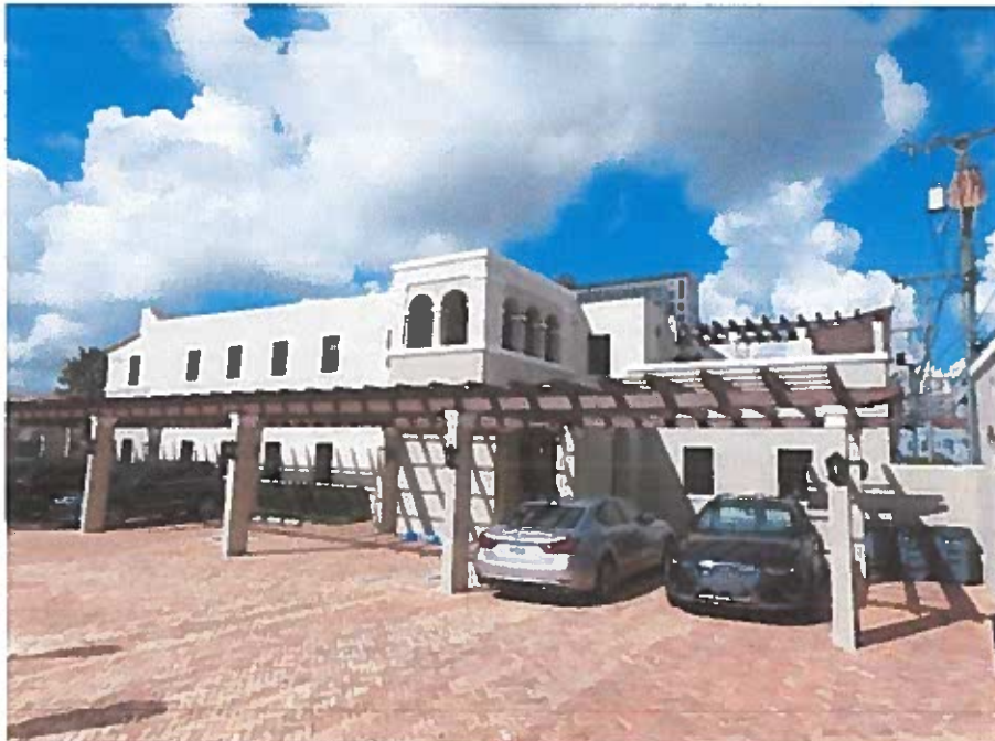
Right side of building
