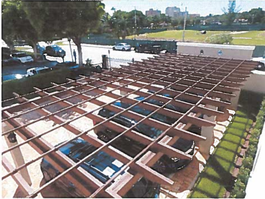
Overview of trellis at parking lot
