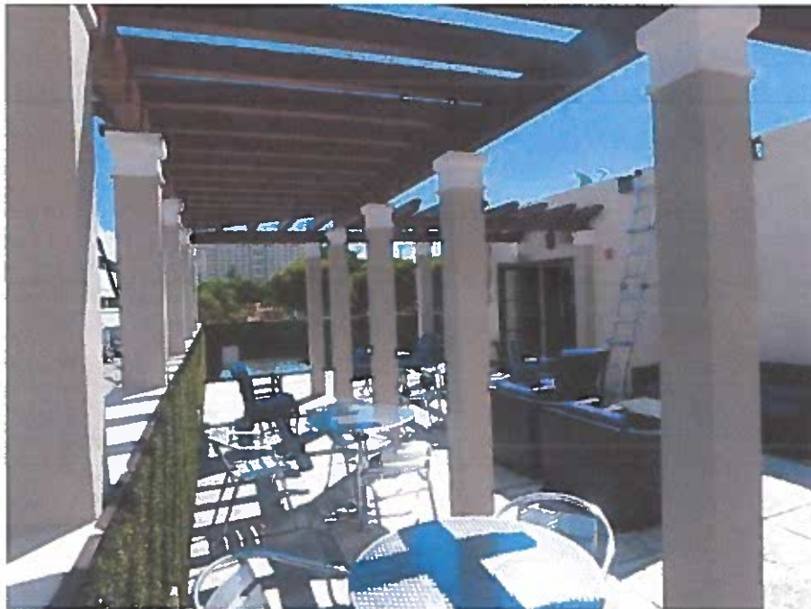
Overview of trellis at patio
