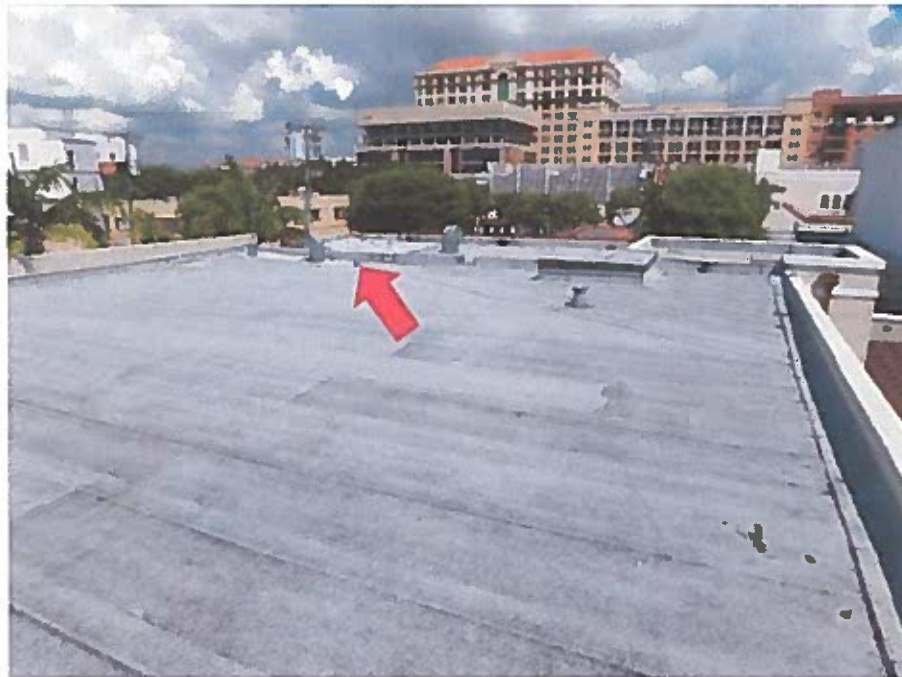
Overview of rooftop with single roof drain
