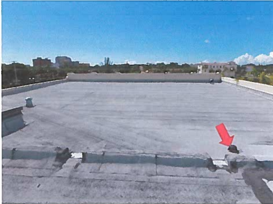
Overview of rooftop with single roof drain
