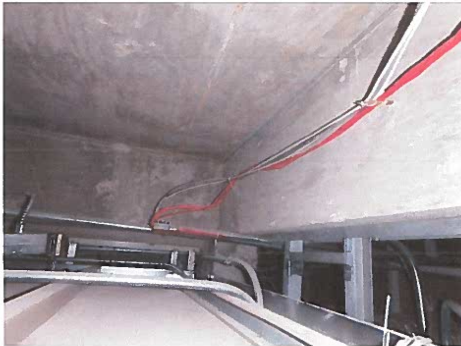
Overview of concrete slab area
