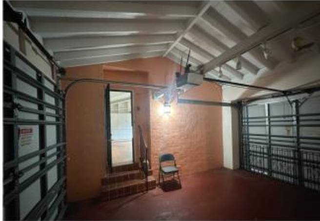
Side entry to home visible, originally accessible from exterior.
