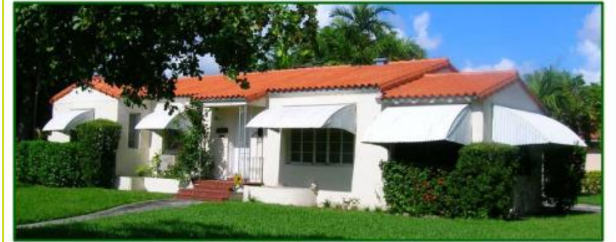
1700 Cortez Street, 1940 Architect: H. George Fink Designated: 2008
