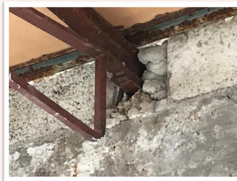
Roof and reinforcement deficiencies at 427 Biltmore Way
