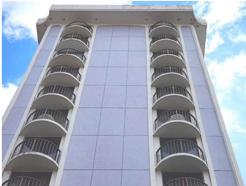
NONE WAS OBSERVED. EAST ELEVATION
