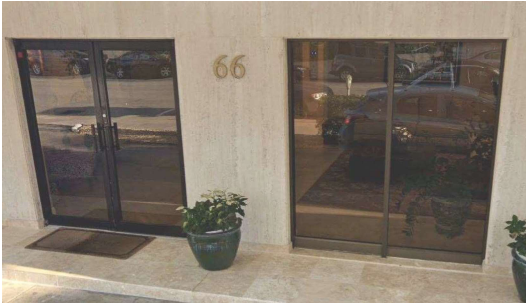
EXTERIOR GLASS DOORS. GOOD CONDITION.
