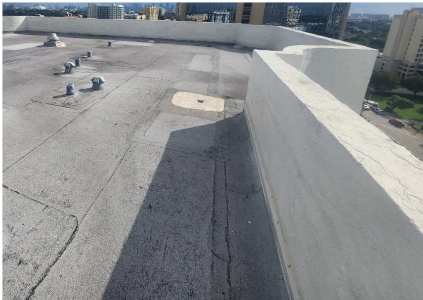
CMU PARAPET. NORTH WEST VIEW FROM ROOF
