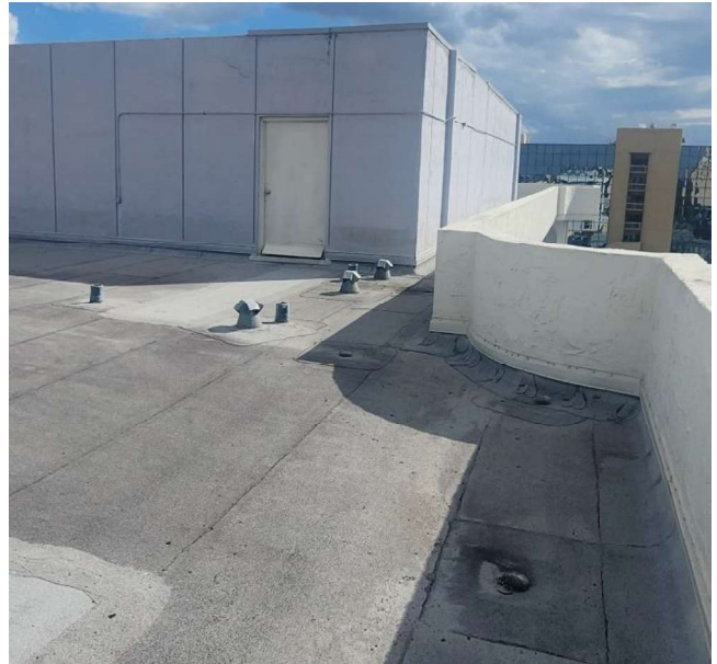
SCUPPERS. GOOD CONDITION. NORTH AND SOUTH VIEW FROM ROOF
