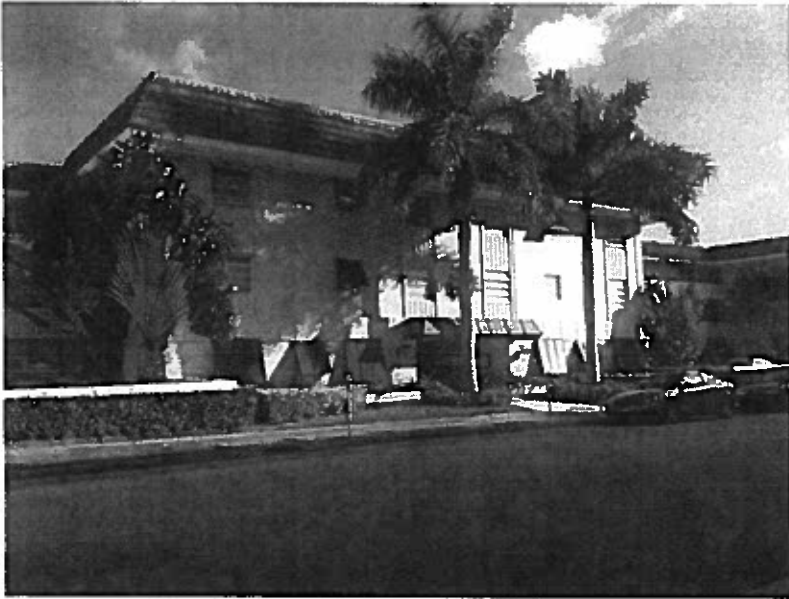
Photograph No. 2 (general building elevation)
