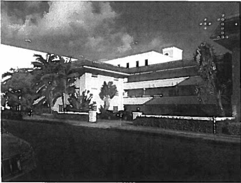
Photograph No. 1 (general building elevation)
