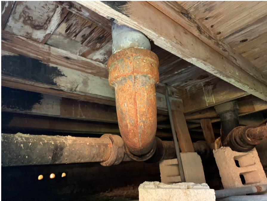
Picture 4 Previously damaged wood floor by water intrusion, not properly repaired. Wood joists supported by unstable blocks and wood posts
