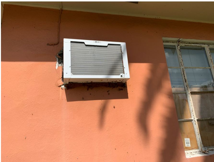
Picture #6 A/C unit not properly encased into the wall.
