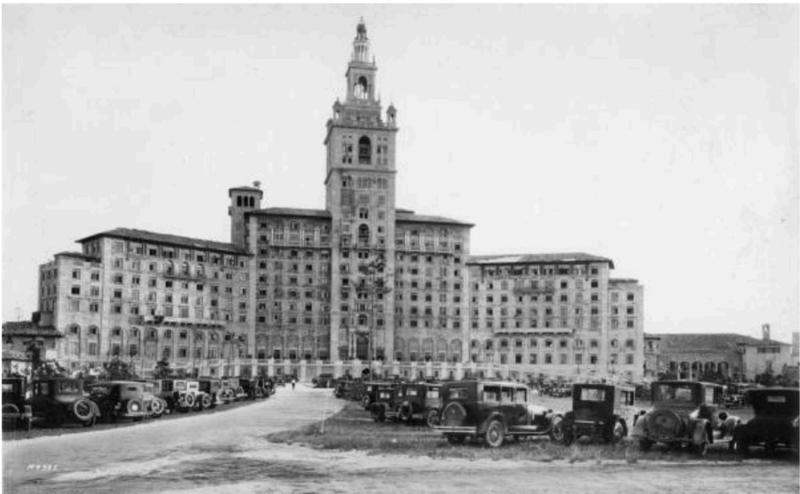
Biltmore Hotel After 1926 Hurricane. Image from Florida Memory.
