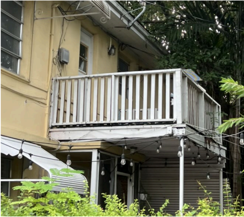
1414 Galiano Street. Photo from Site Visit. Porch Alteration
