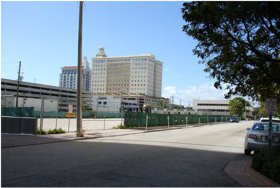
LOOKING SOUTHWESTERLY AT SUBJECT FROM MINORCA AVENUE
