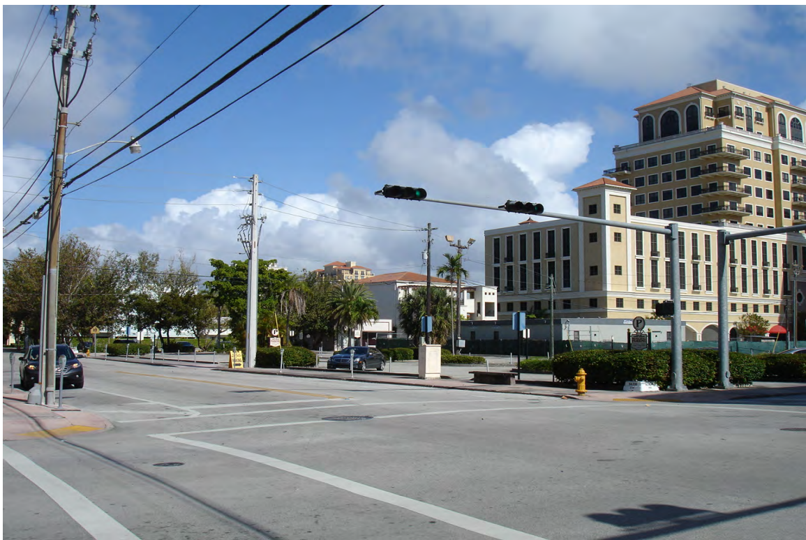
LOOKING NORTHEASTERLY AT PARKING LOT NO. 6 FROM SALZEDO STREET
