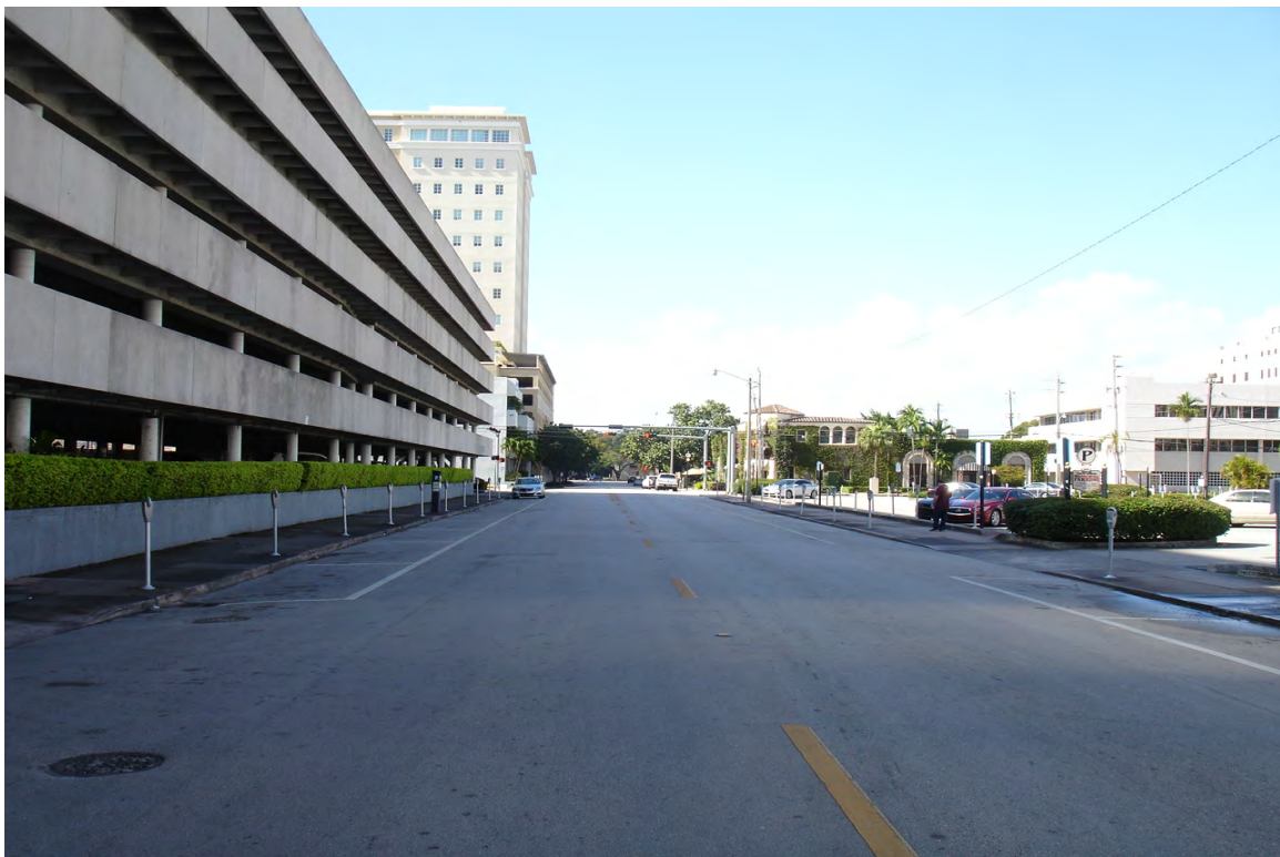
LOOKING WESTERLY ON ALCAZAR AVENUE – PARKING LOT NO. 6 TO RIGHT
