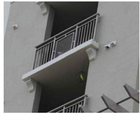
6 42" HIGH A.F.F. SAFEGUARD W/ BALCONIES GABLES PONCE
