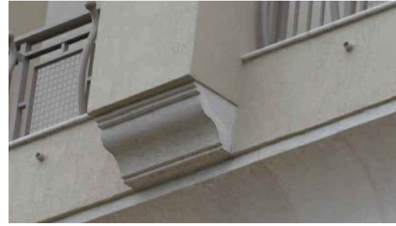
8 PRECAST CONCRETE BRACKETS GABLES PONCE
