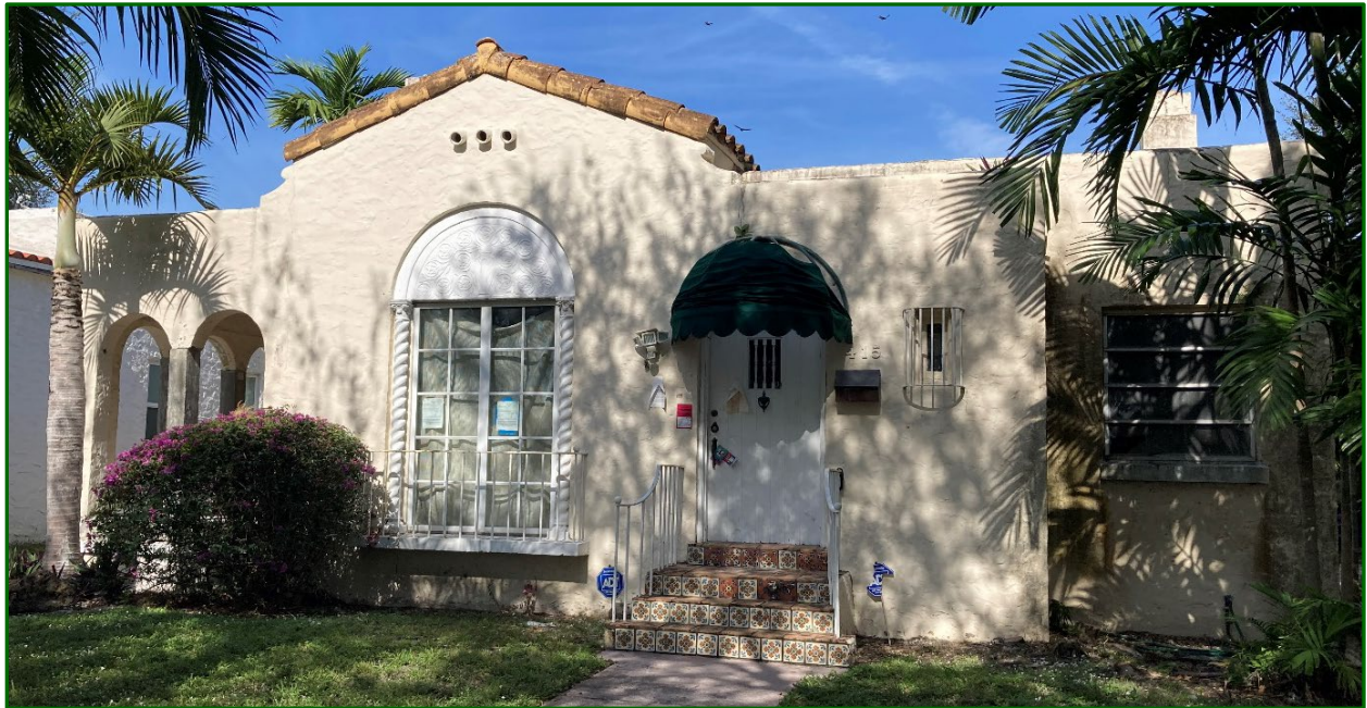
Figure 13: Front (South) Façade, 2023
