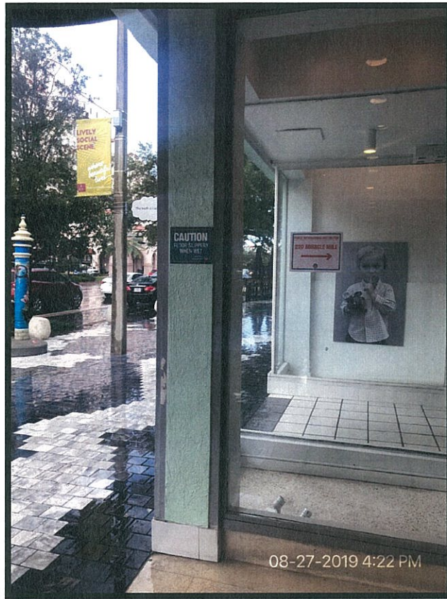
Sign located on NE wall of breezeway
