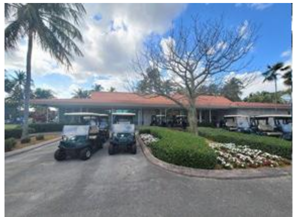
Subject front, view of the golfcart parking
