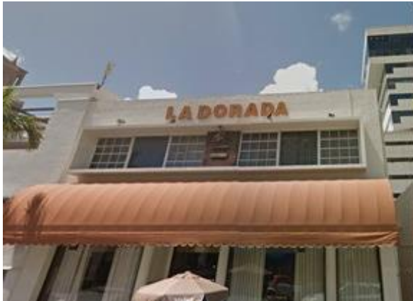
Lease 1 Giralda Plaza Pedestrian Mall Retail
