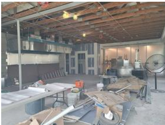
Subject view of the kitchen area
