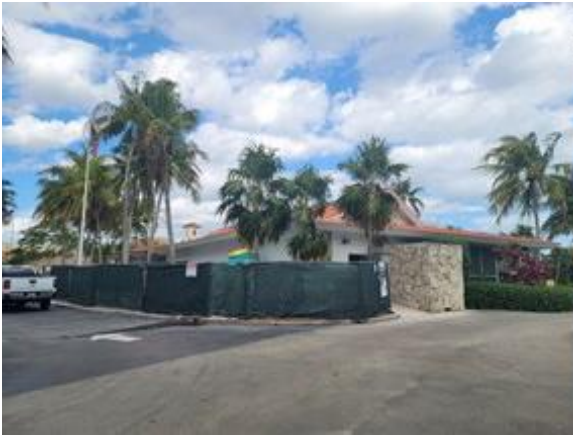
Subject, view of the work area, rear door
