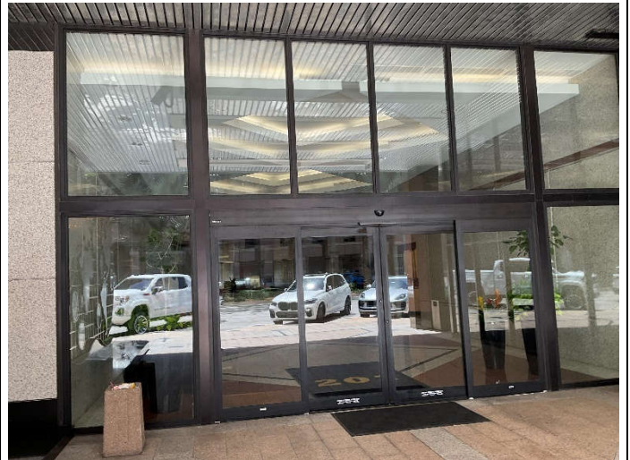
Photo # 48. Close-up view of storefronts at lobby of the building.
