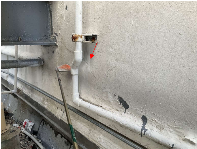
Photo # 23. Delaminated/de-bonded stucco at roof.
