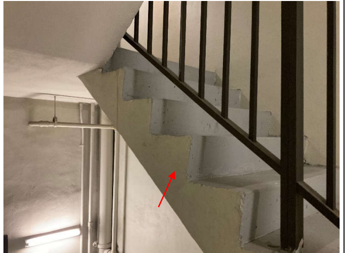
Photo # 42. Reinforced concrete stairs.
