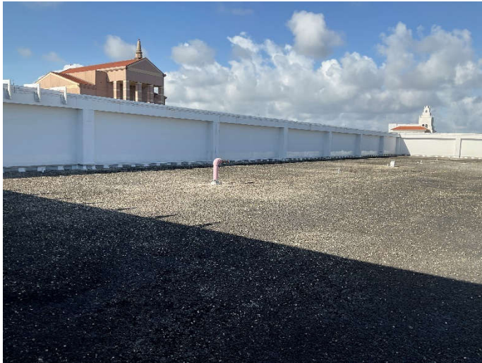
Photo # 35. Parapet wall along the perimeter of roof.
