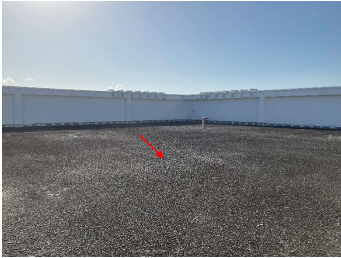
Photo # 31. Existing gravel Built-Up-Roof (BUR) system.
