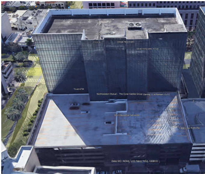
Photo # 3. North elevation.
