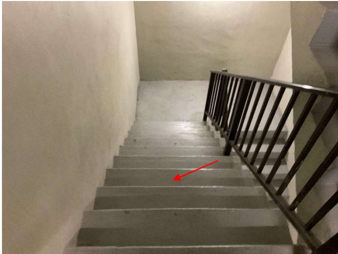
Photo # 41. Reinforced concrete stairs.
