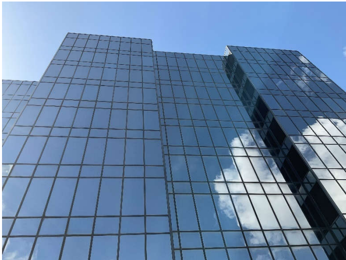
Photo # 47. Overall view of curtain wall at building façade.
