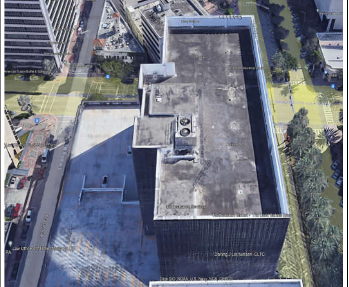
Photo # 4. West elevation.
