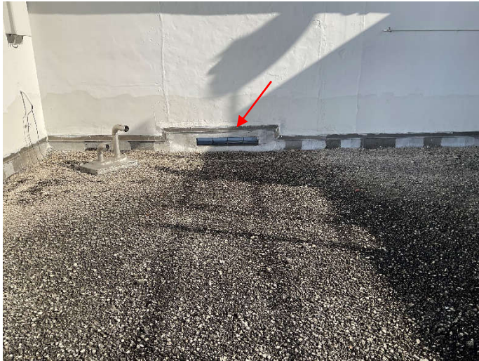
Photo # 37. Overflow scuppers at roof.
