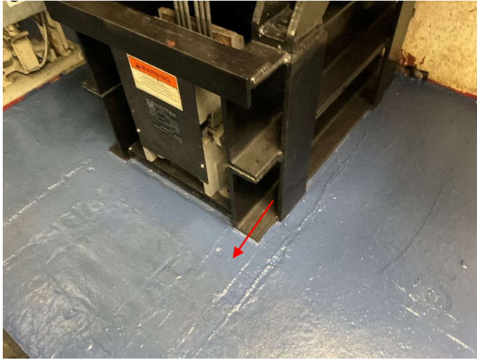
Photo # 45. Close-up view of elevator sheave beam.
