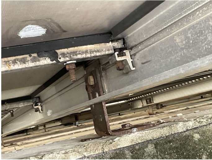
Photo # 49. Overall view of curtain wall anchors.
