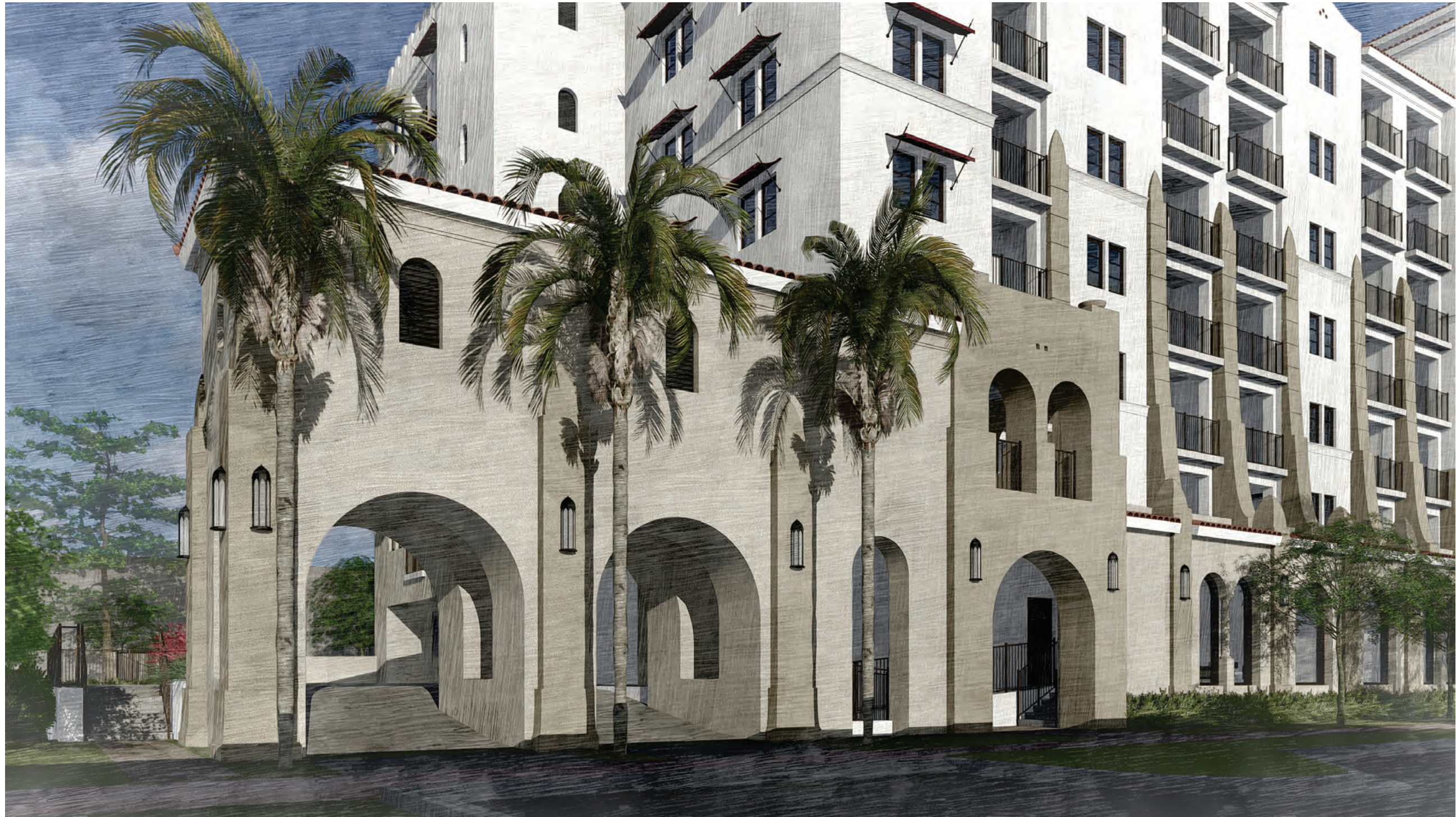
PARKING GARAGE ENTRANCE | NORTH VIEW
