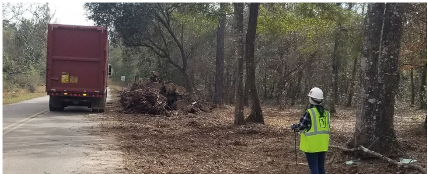
Figure 6. ROW Monitoring following Hurricane Sally, Baldwin County, Alabama
