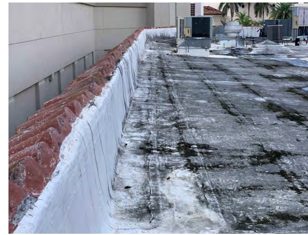
PHOTO 5 - EXISTING BARREL TILE ON COPING
