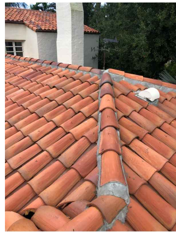
PHOTO 2 - ARTISAN BLEND CLAY ROOF TILES
