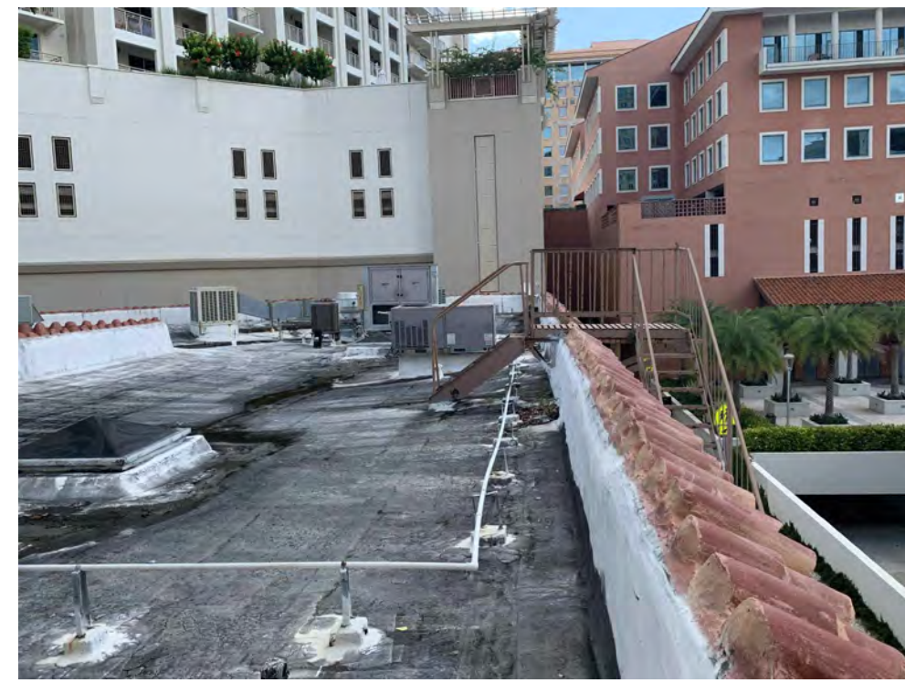
PHOTO 3 - EXISTING BARREL TILE ON COPING
