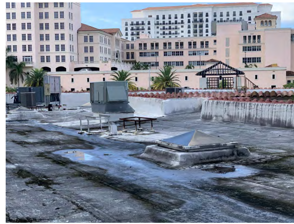
PHOTO 4 - EXISTING ROOF CONDITION
