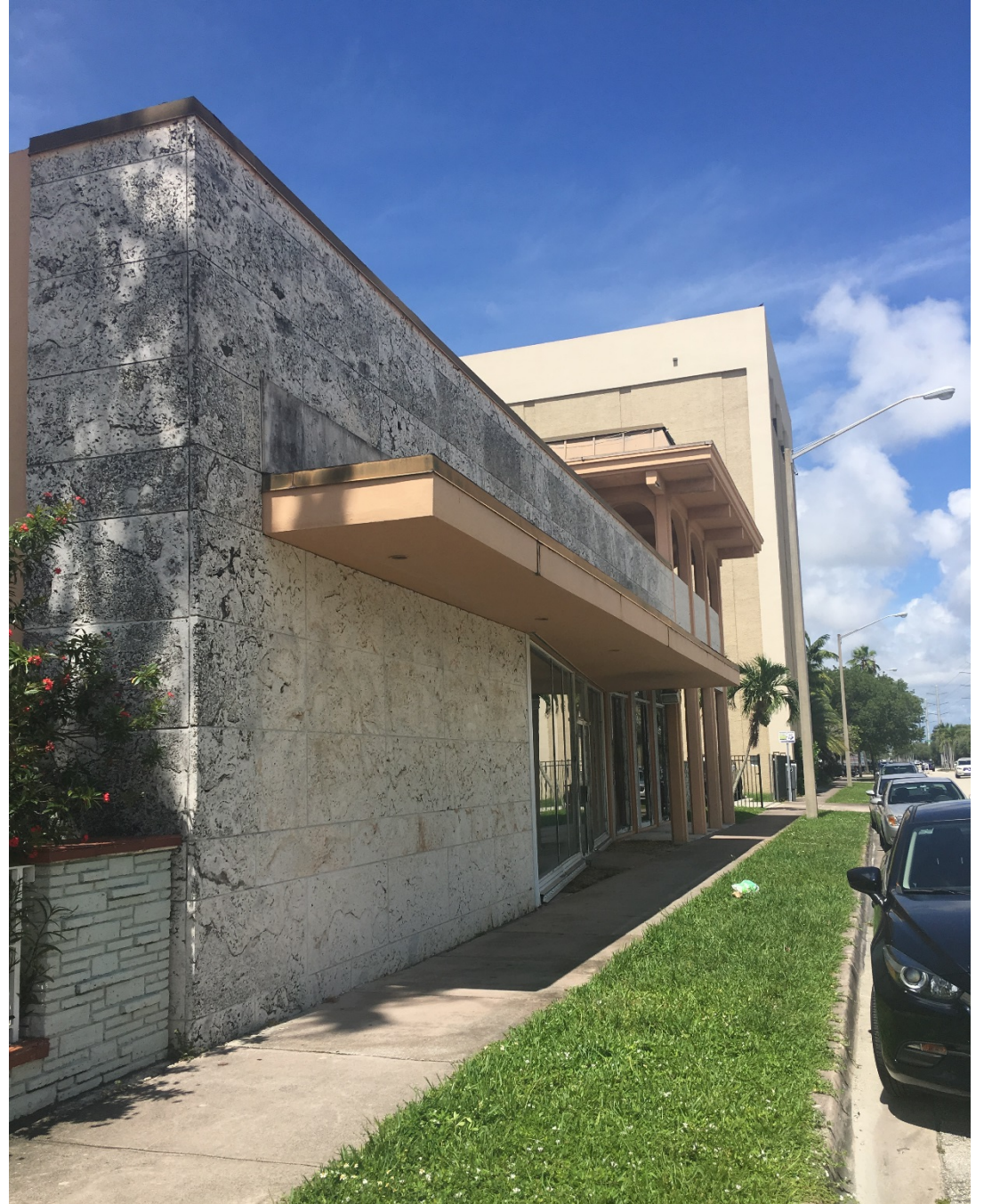
Neighboring Properties along Ponce de Leon facing north
