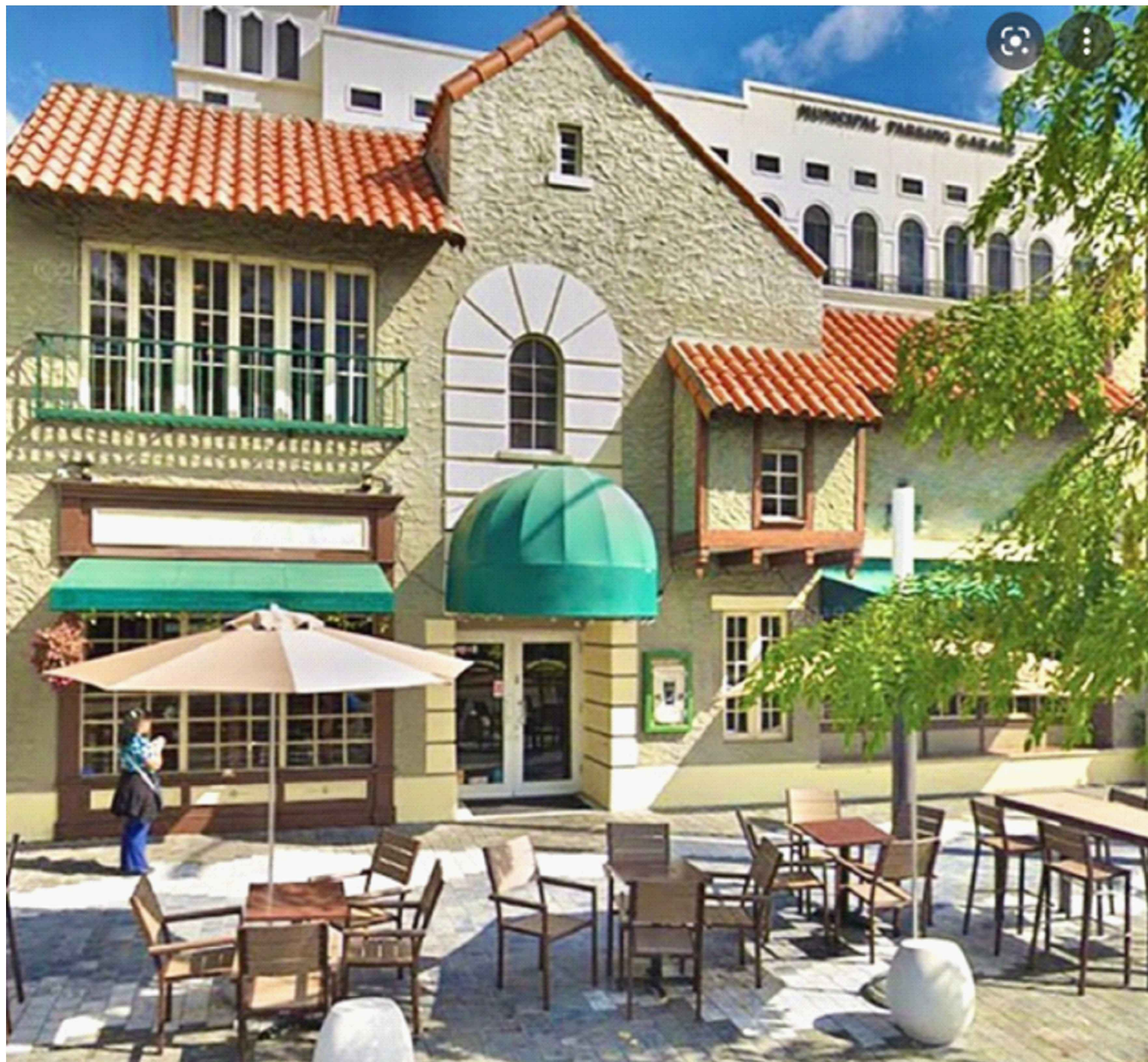
IMAGE - EXISTING FACADE
