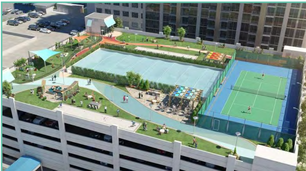
SkyHouse Uptown Parking Deck, Charlotte, NC (photo credit: Charlotte Observer)
