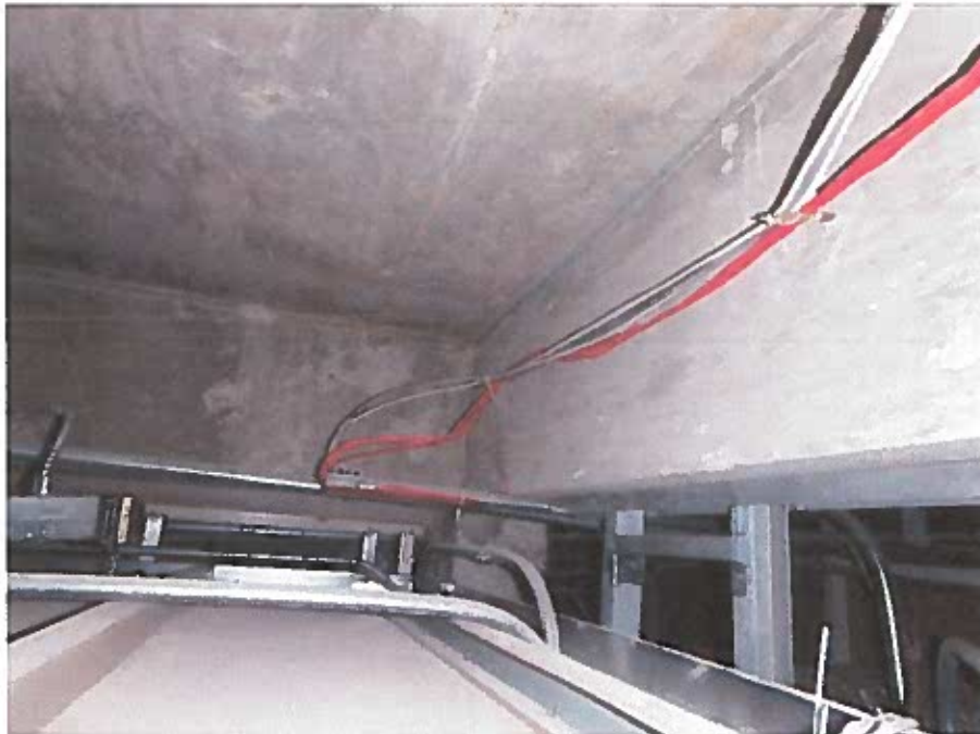
Overview of concrete slab area
