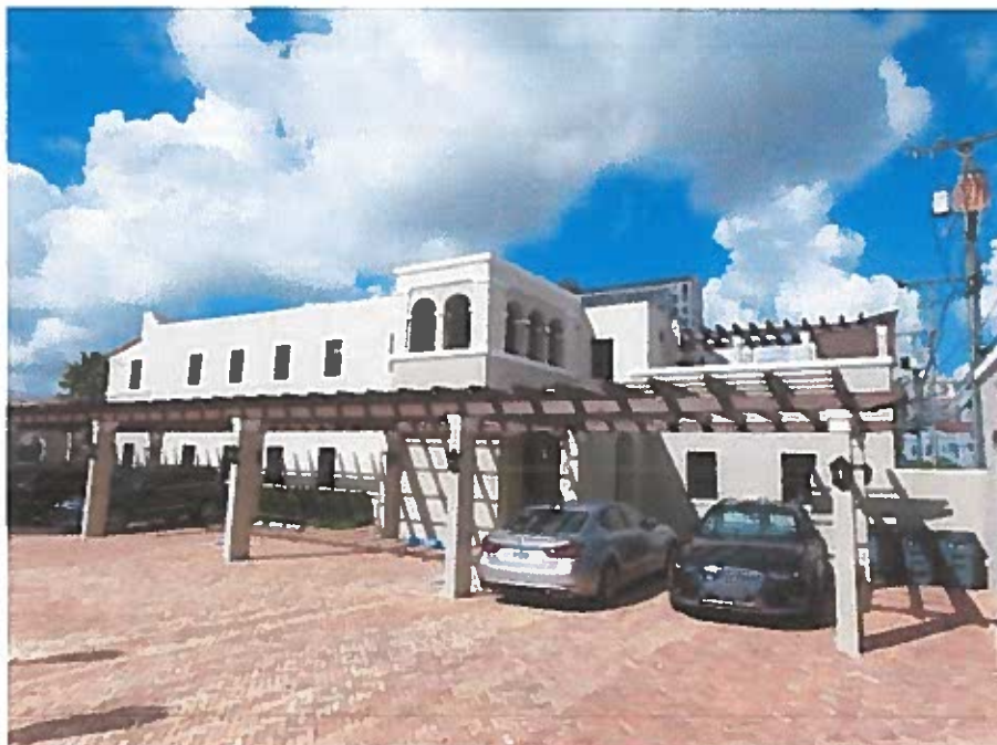
Right side of building
