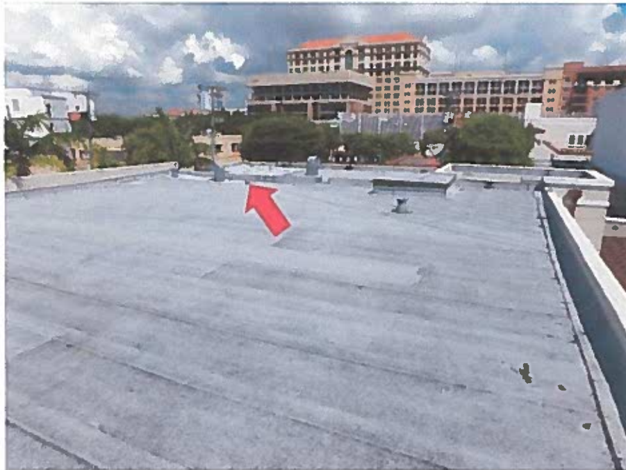
Overview of rooftop with single roof drain
