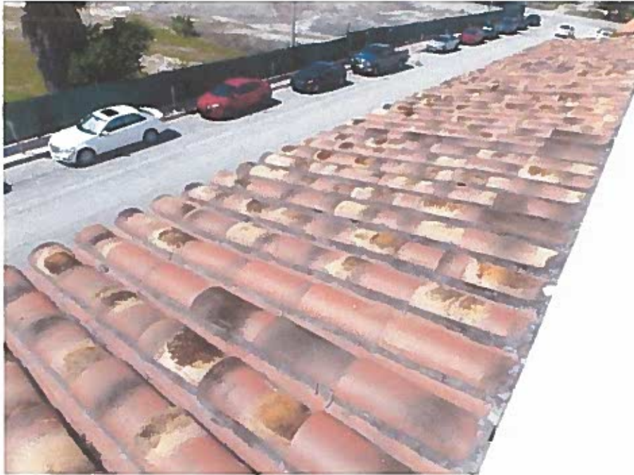
Overview of tile roof at front of building
