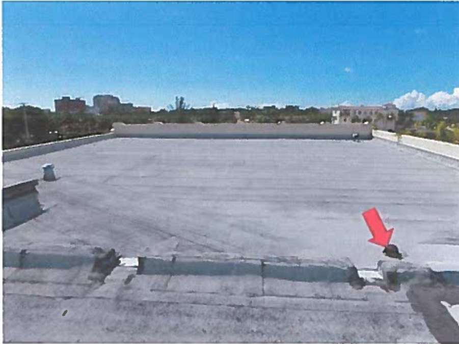
Overview of rooftop with single roof drain
