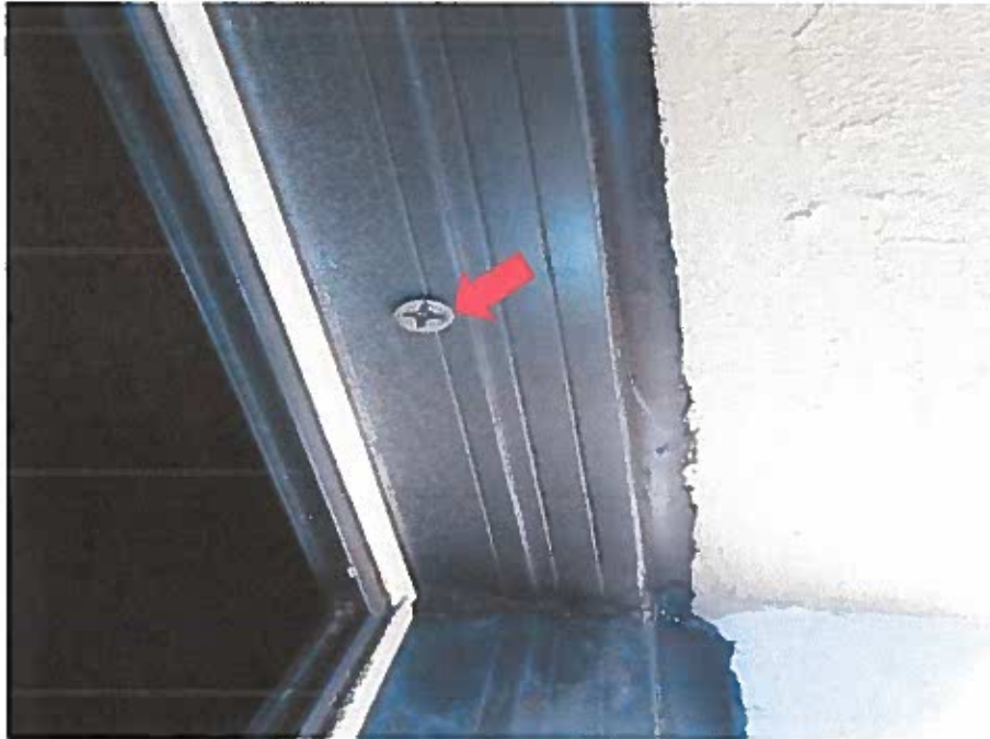
Screw fasteners at window jamb
