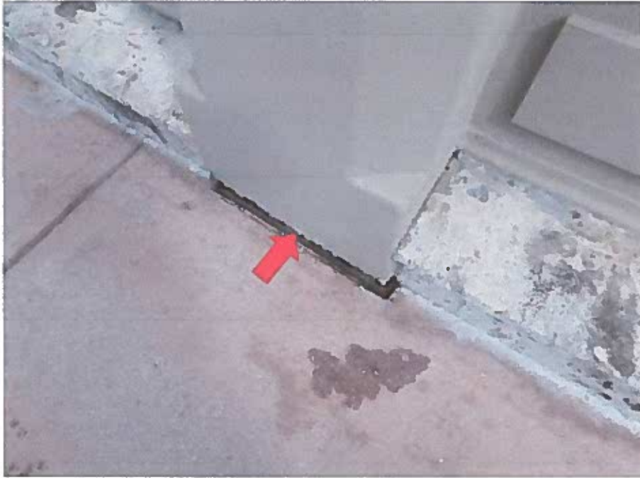
Expansion joint at sidewalk
