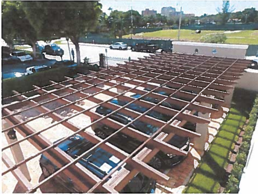
Overview of trellis at parking lot
