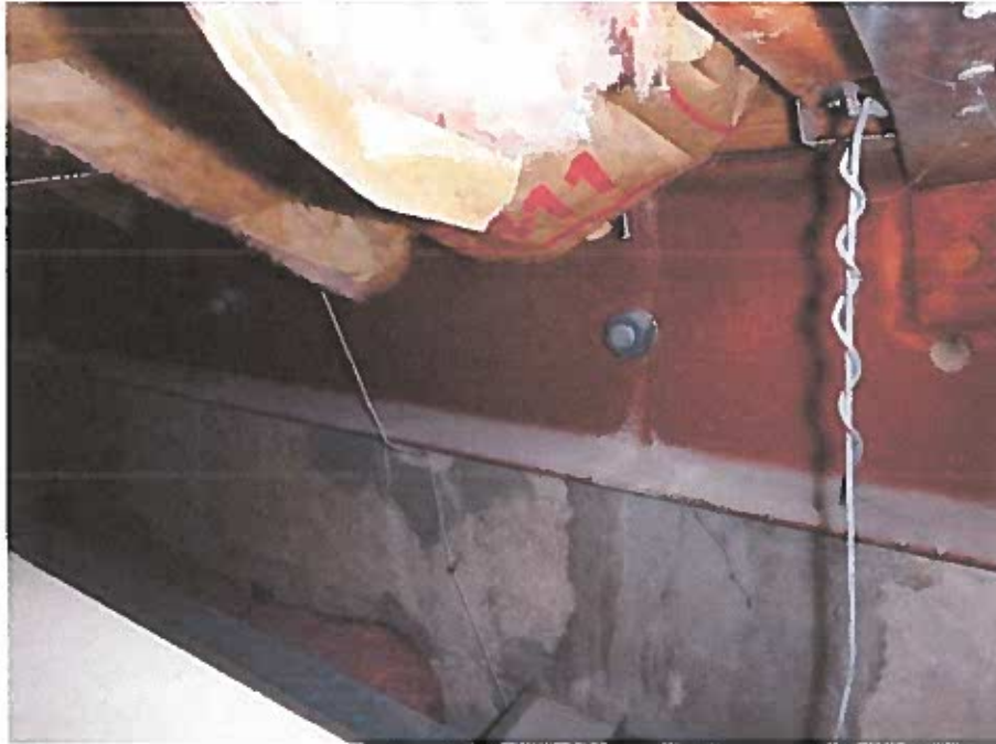
Overview of external steel reinforced concrete beam and tie-column
