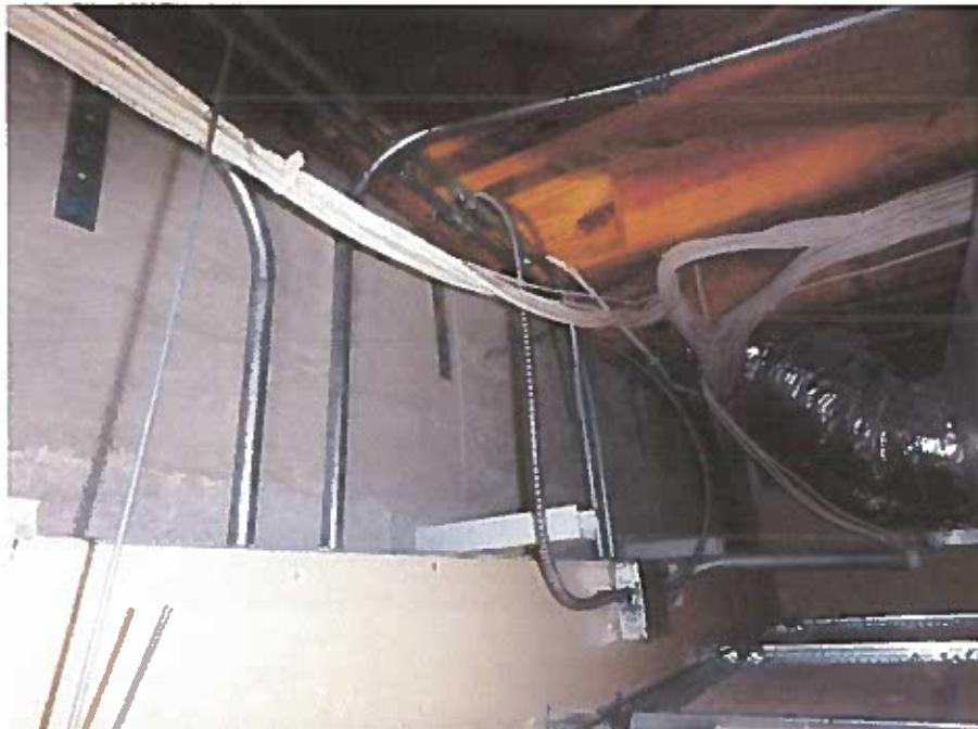
Overview of typical wood floor framing over concrete beam
