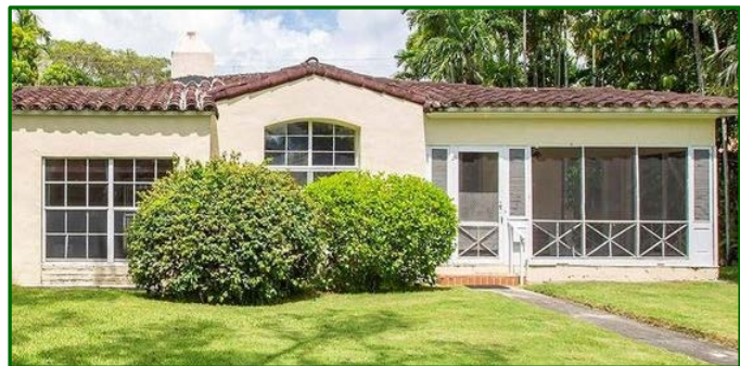
Figures 13: Garage Enclosure, 2020 Note: brick below infill windows; discernable original opening; floor level, step tile Courtesy of Realtor.com
