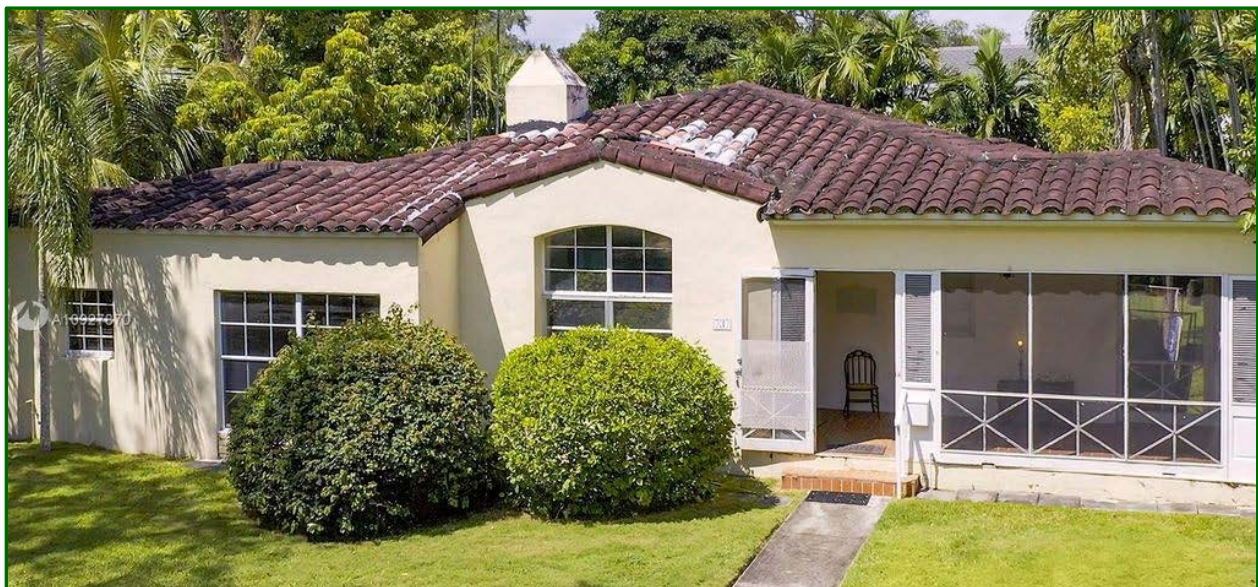
Figures 8: 737 Minorca Avenue Permit #5383, 1937 [top]; Historic Photo, c.1940 [center] Current Photo, 2020: [bottom] Courtesy of Realtor.com Note: Rendering shows flat tile roof; original installed roof was barrel tile
