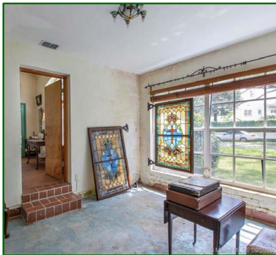
Figures 13: Garage Enclosure, 2020 Note: brick below infill windows; discernable original opening; floor level, step tile Courtesy of Realtor.com
