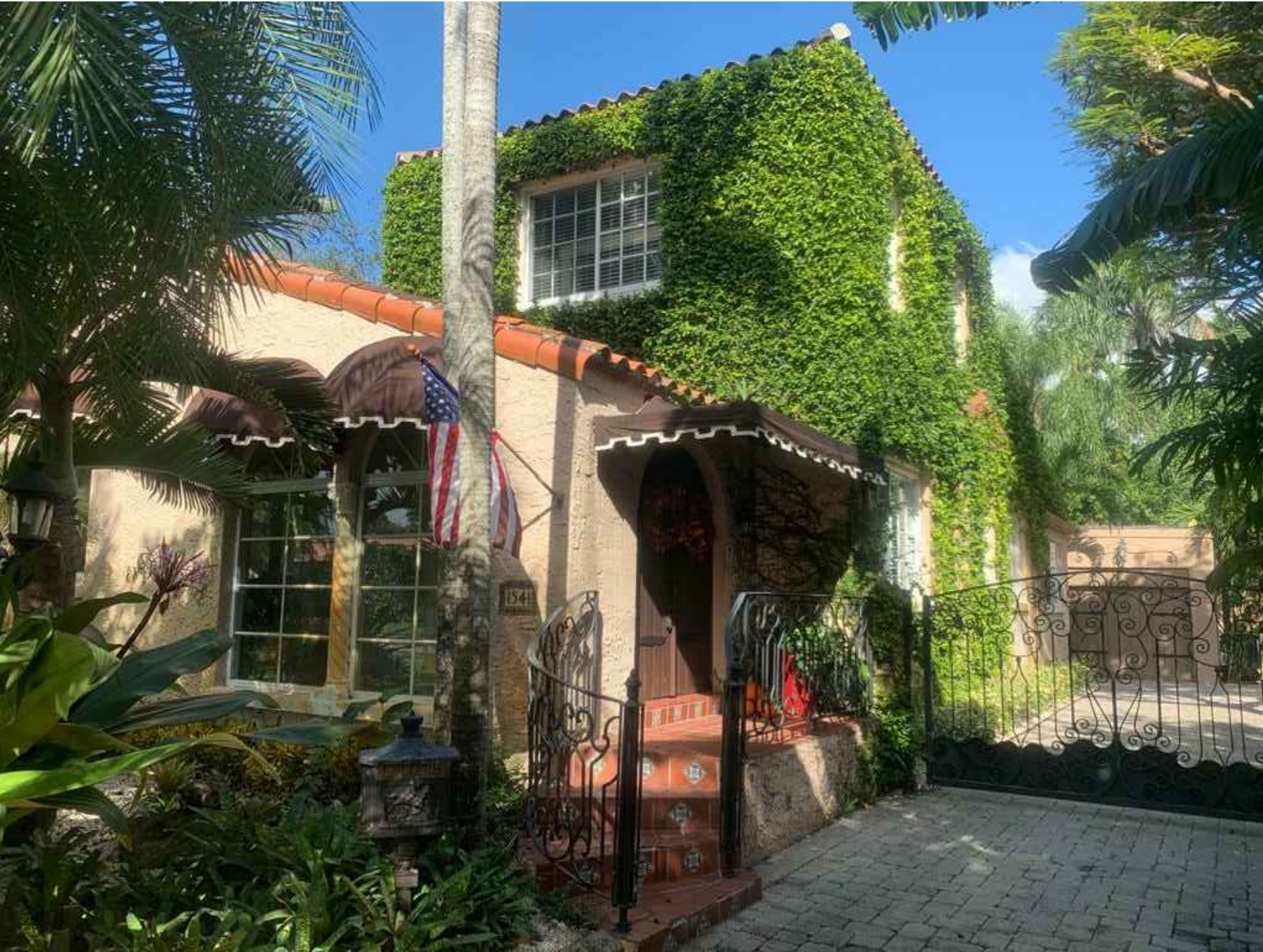
FRONT VIEW FROM DRIVEWAY.
