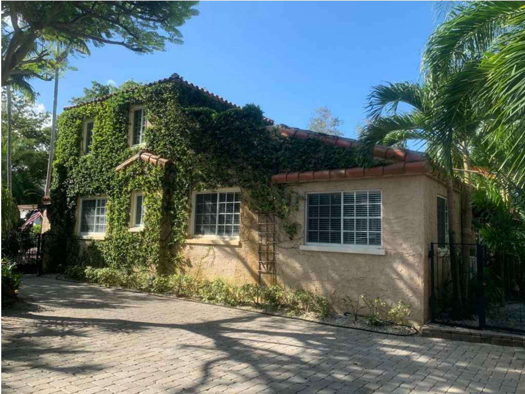
SIDE VIEW FROM NORTH-EAST CORNER
