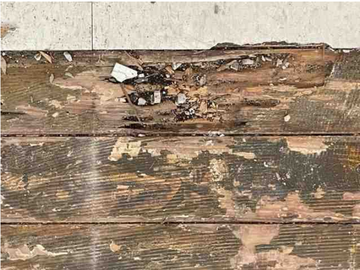
Termite Damage
