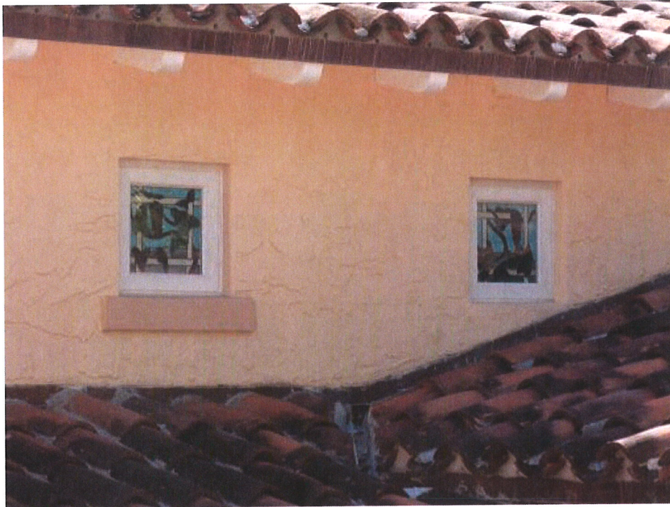
PHOTO #13—Second Level West Facing Window Detail
