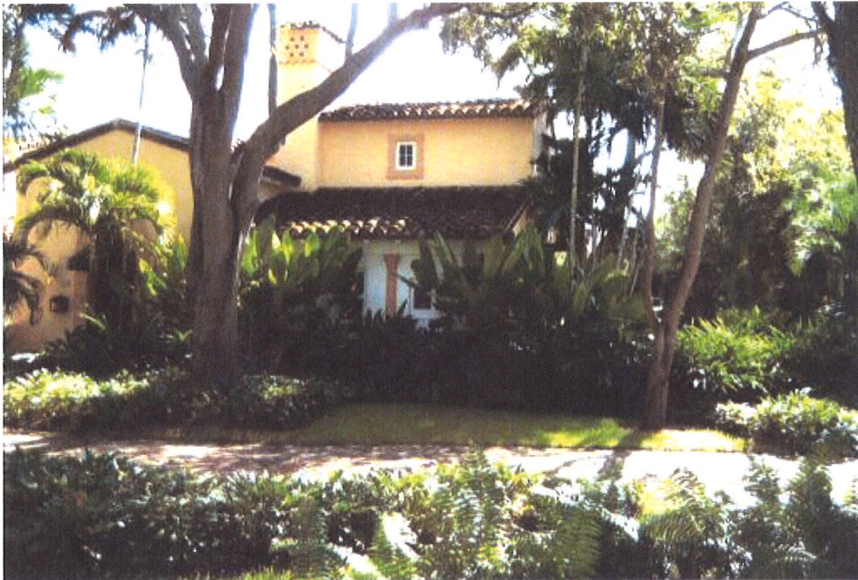
PHOTO #11—Southwest (Front Facade) Elevation
