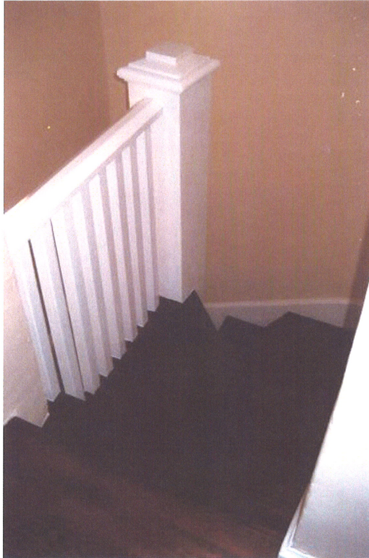
Restored Secondary Stairs
