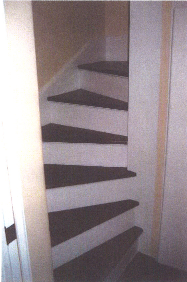
Restored Secondary Stairs
