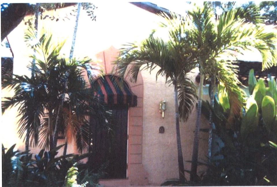
PHOTO #10—West (Front Facade) Entry Door Elevation
