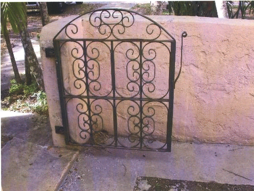
Typical Gate – Prior to Restoration
