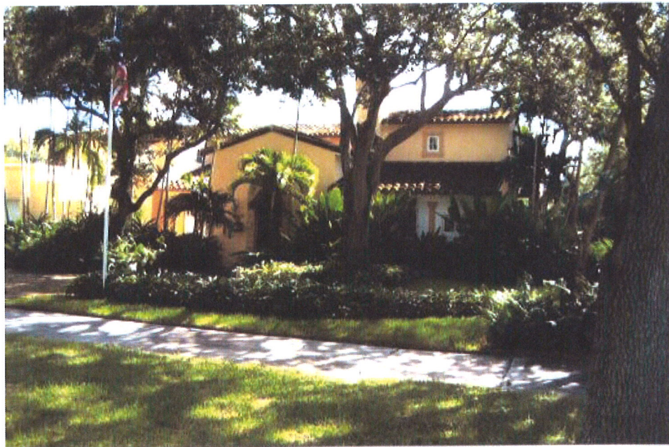
PHOTO #8—West (Front Facade) Elevation
