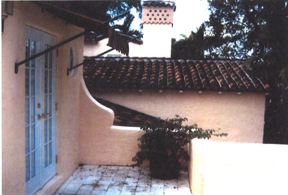
PHOTO #35 – Garage Roof Terrace
