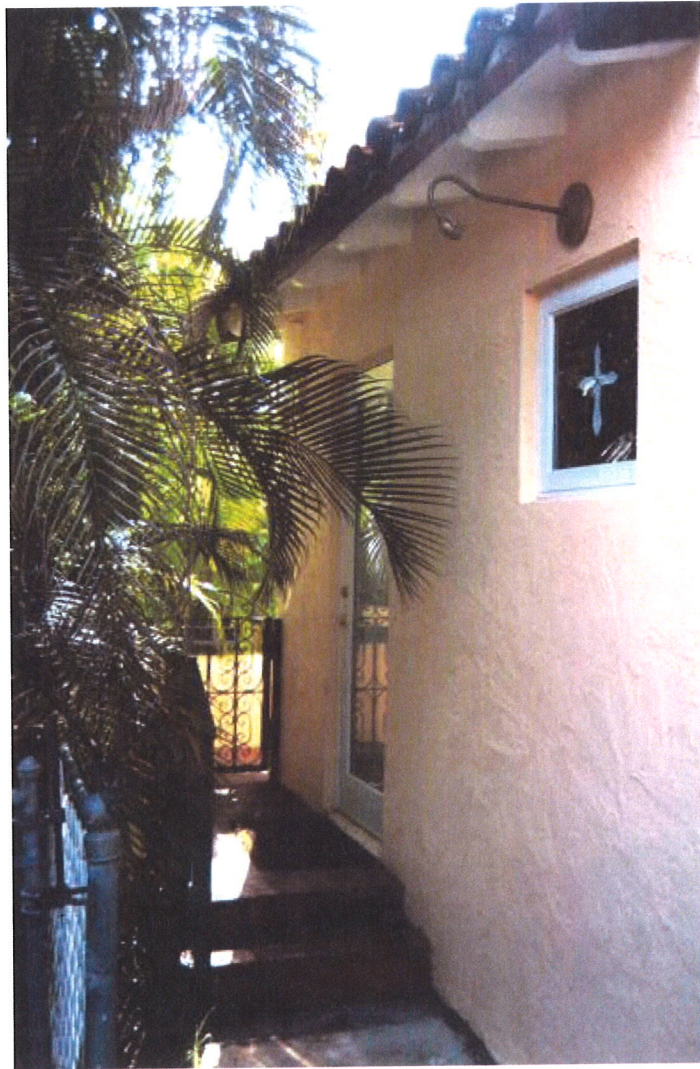
PHOTO #15—North Partial Interior Side Elevation
