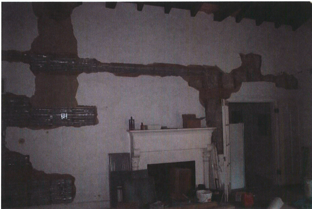
Typical Interior Plaster Repair – Living Room
