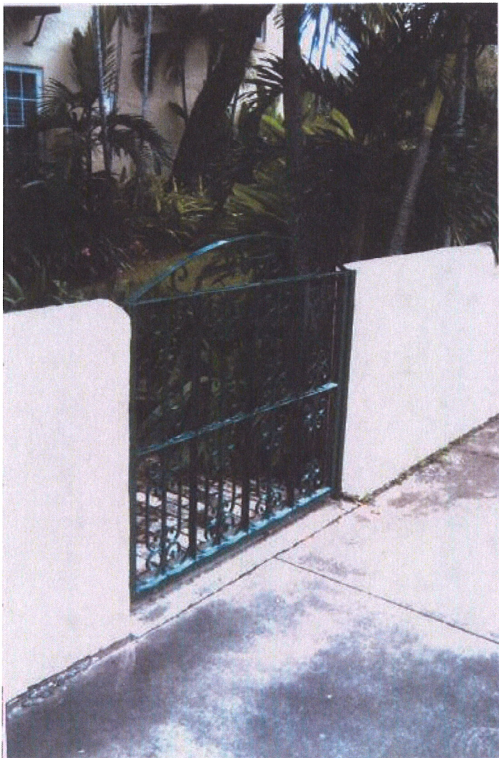
PHOTO #42 – Gates, Grillework, Restored Wall South Street Side Facing
