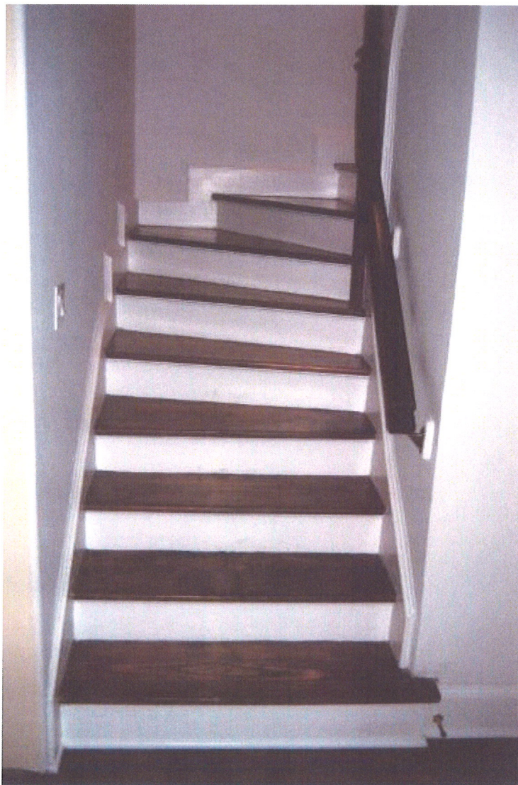
Restored Main Stairs
