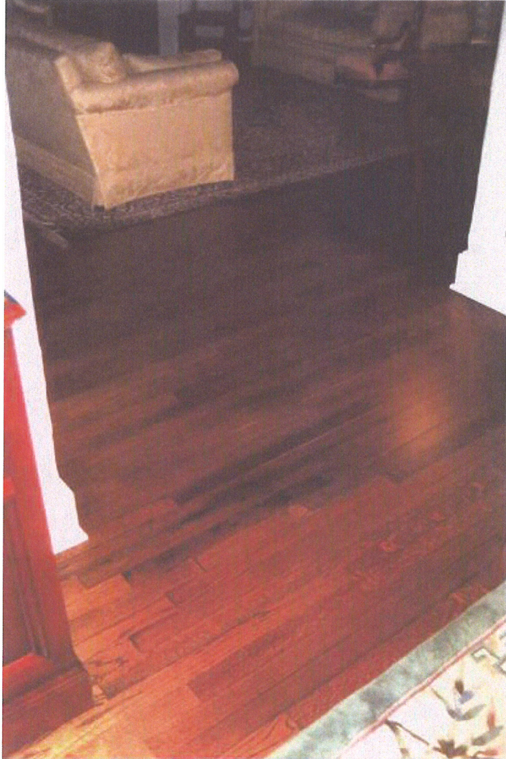
Restored & Reworked Flooring
