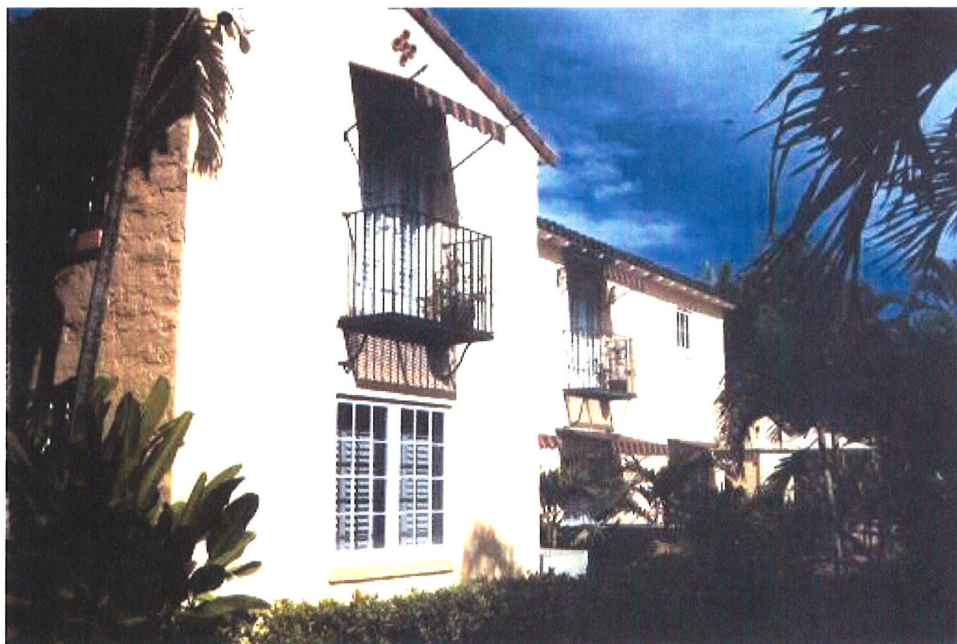
PHOTO #4—East (Rear Facade) Elevation Southeast Bedrooms
