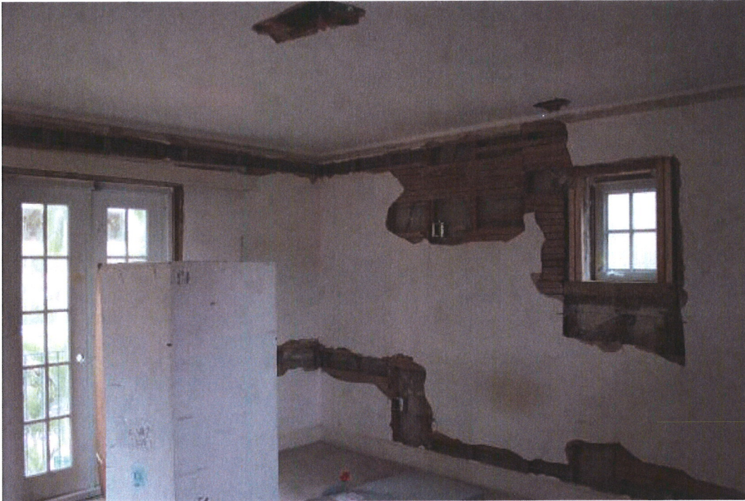
Typical Interior Plaster Repair Bedroom
