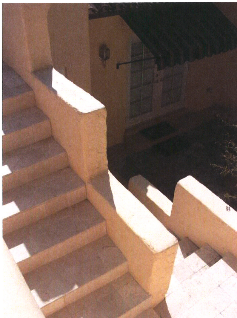
PHOTO #39 – Garage Roof Terrace Stair
