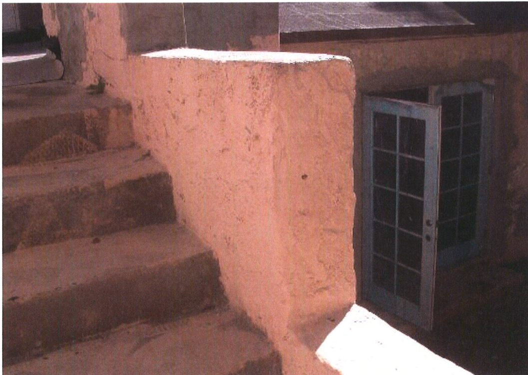
Garage Staircase to Patio – in Progress
