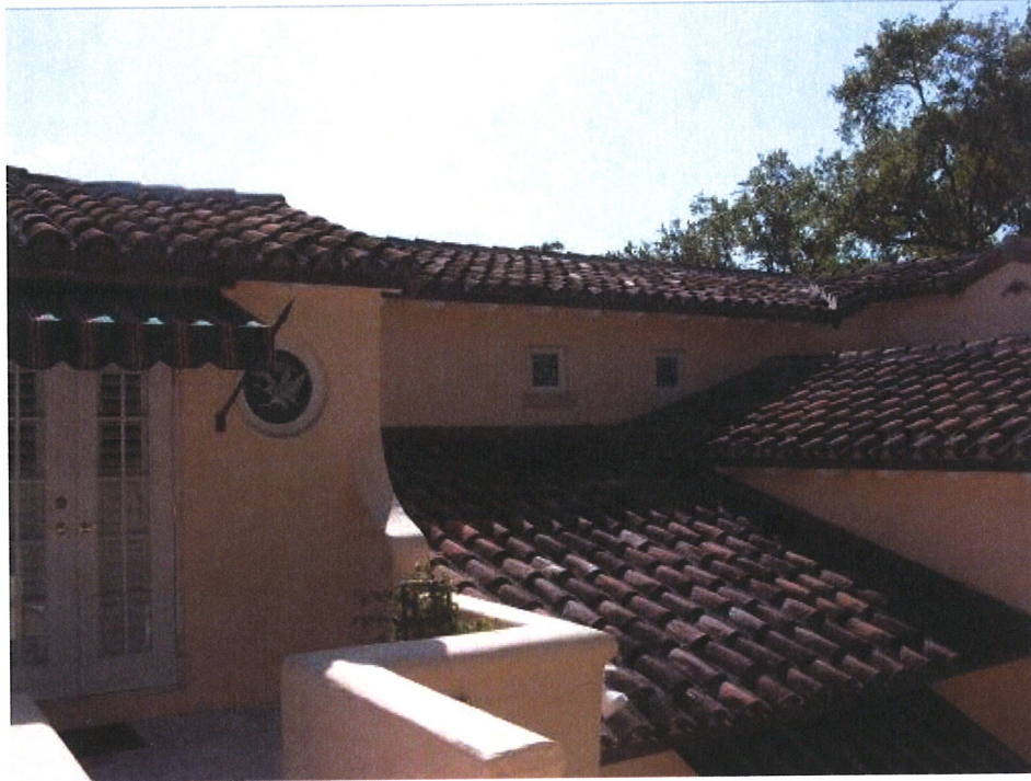
PHOTO #9—West (Front Facade) 2 nd floor Addition from Garage Roof Terrace
