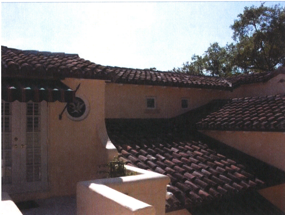
PHOTO #36 – Garage Roof Terrace
