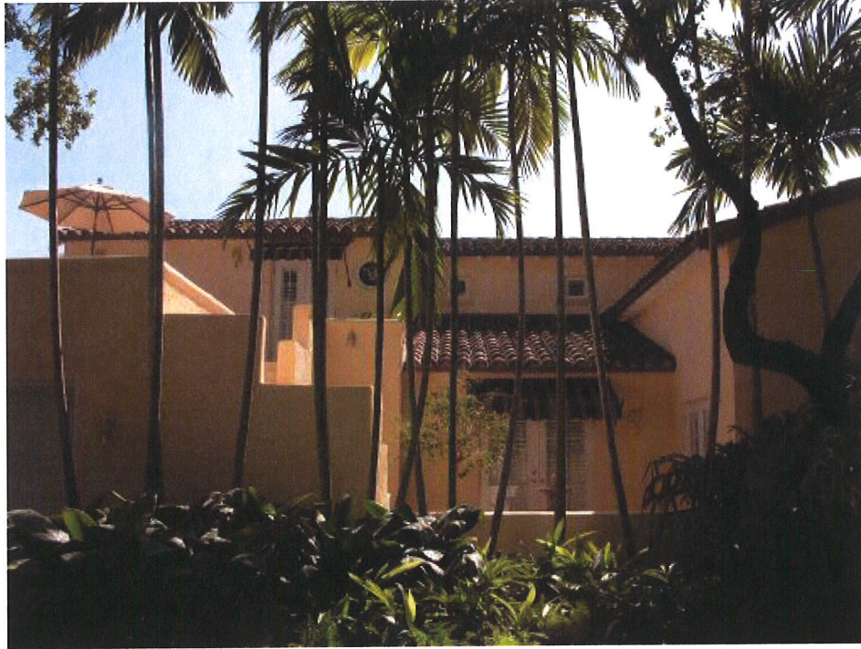
PHOTO #7—West (Front Facade) Elevation (Front Terrace)
