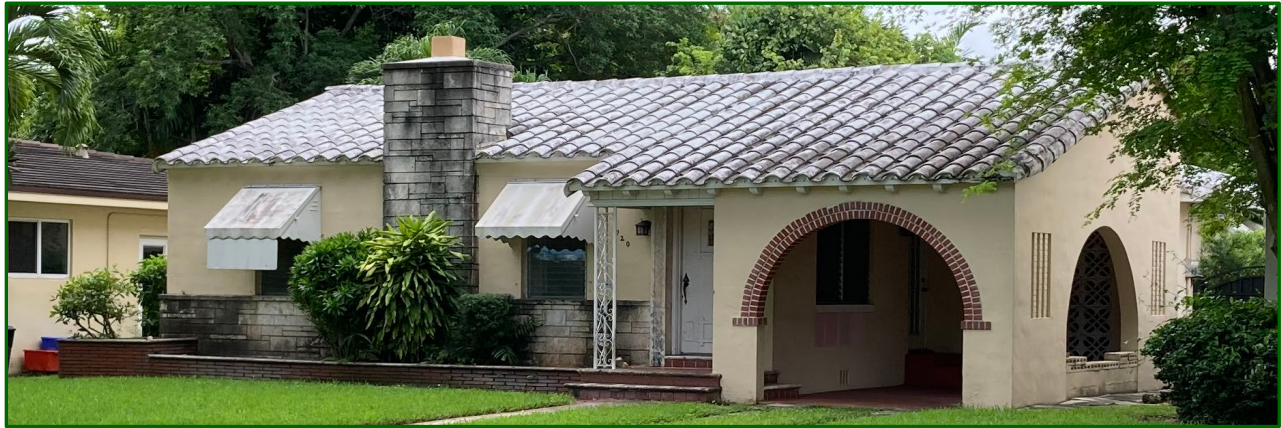
Figure 17: Front (North) Façade, 2024
