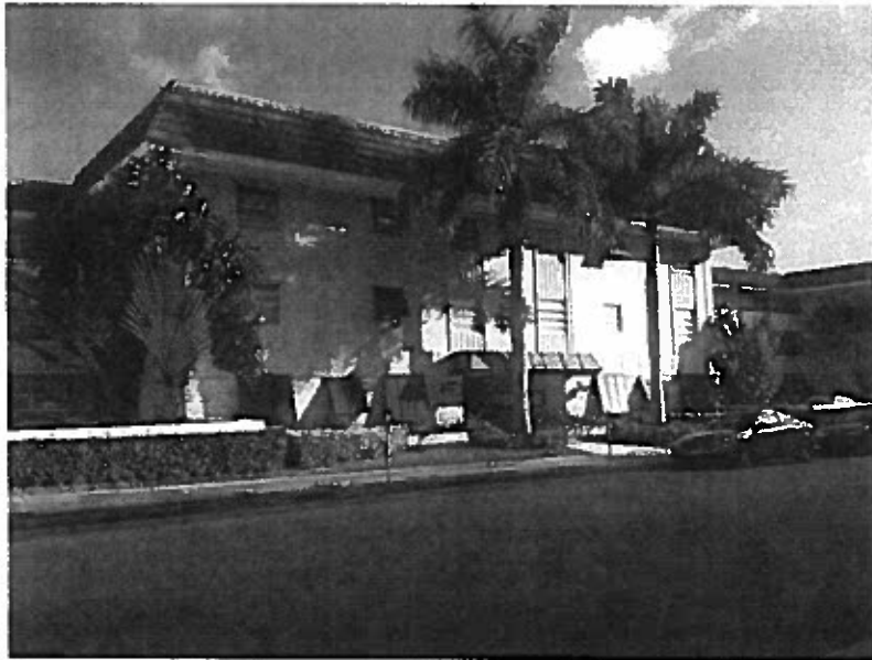
Photograph No. 2 (general building elevation)
