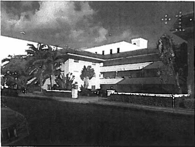
Photograph No. 1 (general building elevation)
