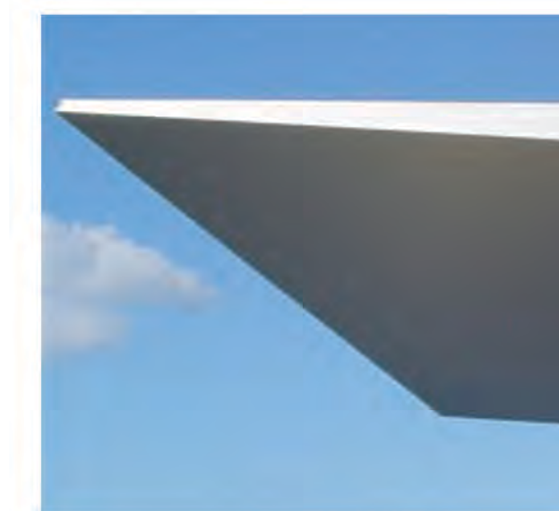
TAPERED CONCRETE OVERHANG
