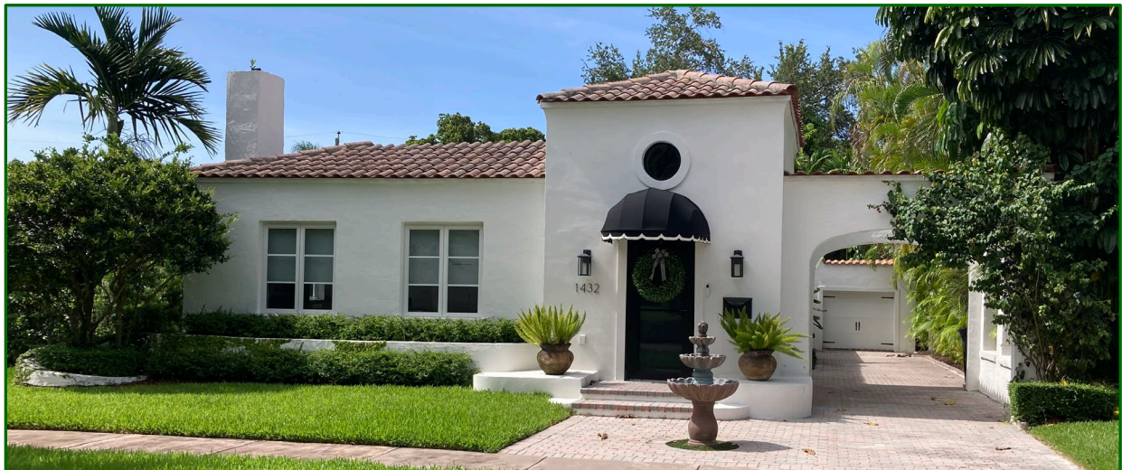
Figure 16: Front (North) Façade, 2024
