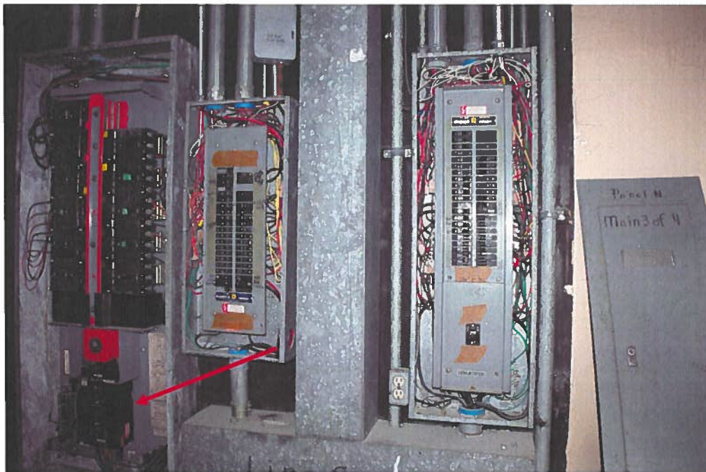
Figure 2: Regular Image of 400A DP Main 4 of 4
