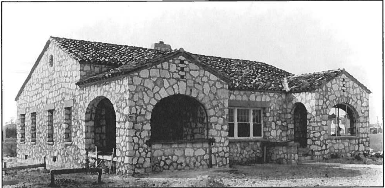
Figure 1: November 15, 1923 Fishbaugh photo, Under Construction
