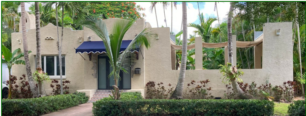
Figure 14: Front (South) Façade, 2025 1923 Original Home with 1993 Open-air Terrace
