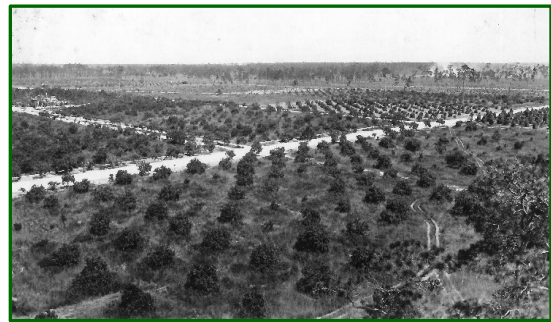
Figure 1: Streets in Coral Gables Under Construction, July 22, 1922
