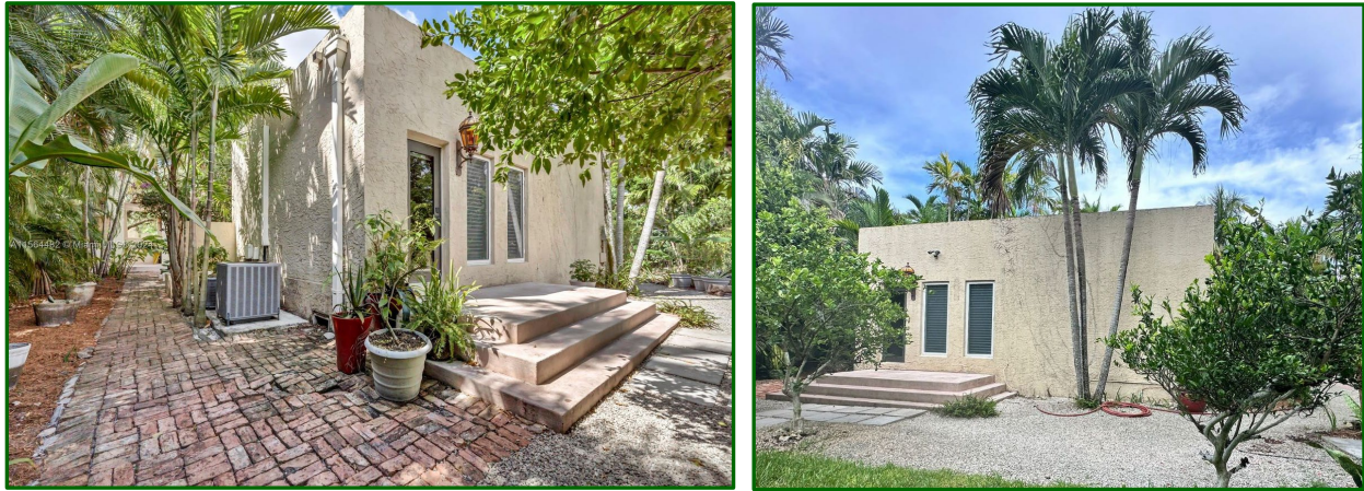
Figures 20: 1960 Rear Addition, 2024: Northeast Corner [left]; North Façade [right] Courtesy Realtor.com
