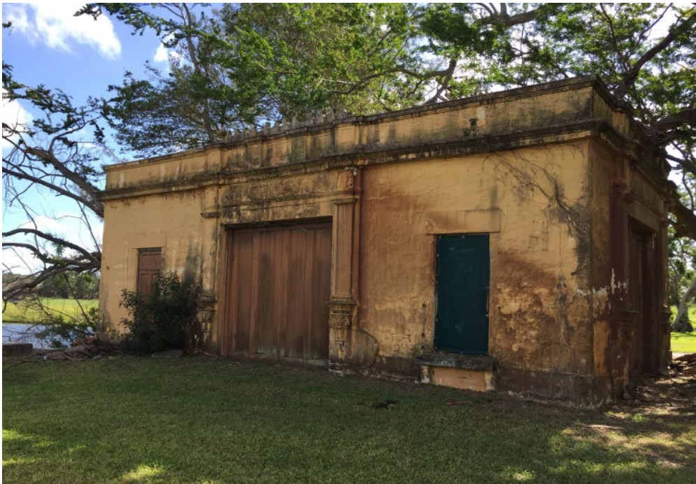
Gondola Building, December 2017
