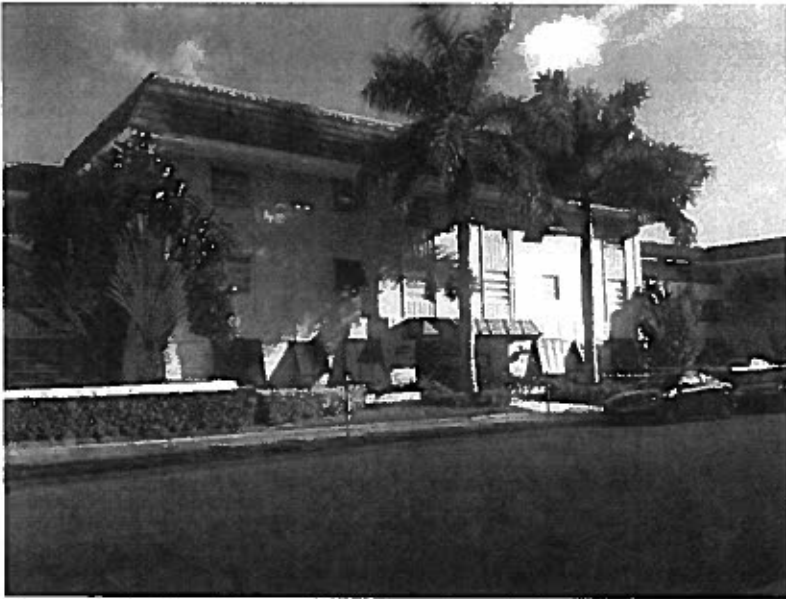
Photograph No. 2 (general building elevation)
