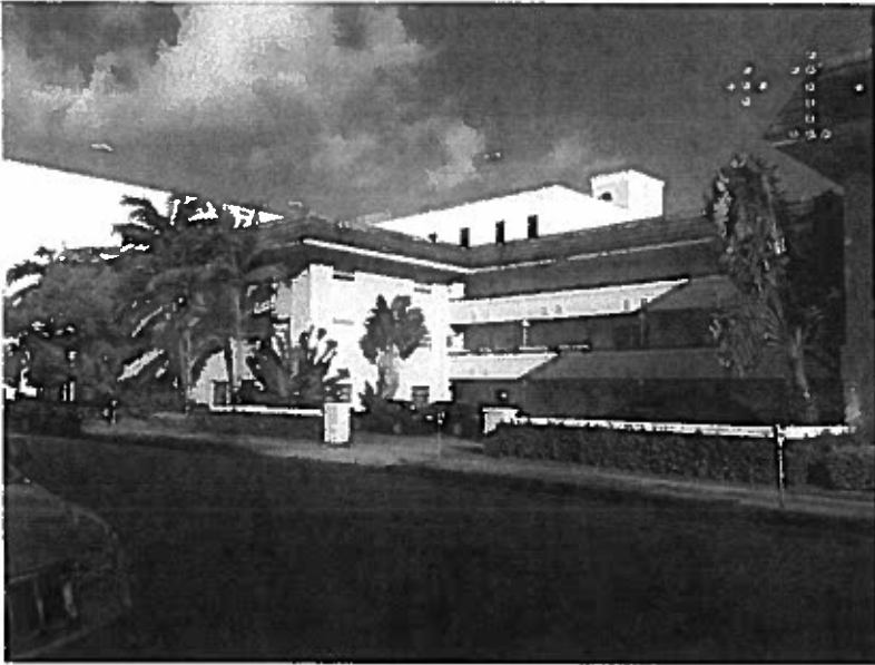
Photograph No. 1 (general building elevation)
