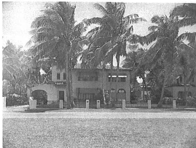
Fig. 1 1940s photograph of front facade
