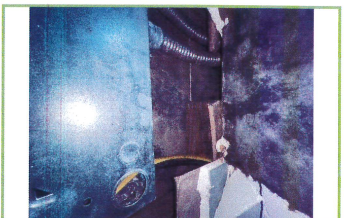
Photograph #6: Bathroom East Wall – Photo depicts wall access location and SVMG on backside of building material (bedroom wall).
