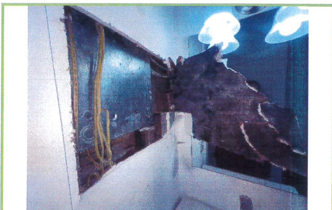
Photograph #5: Bathroom East Wall – Photo depicts wall access location and SVMG on backside of building material (bathroom wall).
