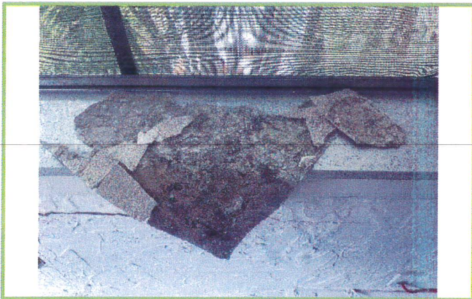
Photograph #3: Living Room West Perimeter Wall – Photo depicts backside of wall texture with SVMG.
