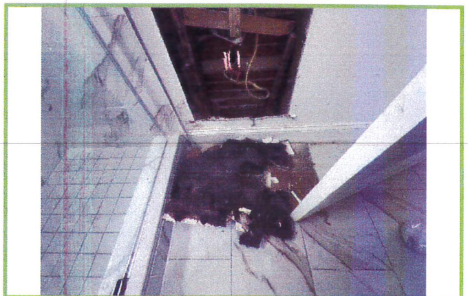
Photograph #4: Bathroom North Wall – Photo depicts wall access location.
