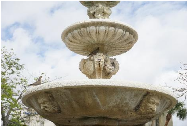
Figure 12. Undersides of lower marble and middle basin; soiling, discoloring, and mineral accretion (photo by EverGreene, February 2021).
