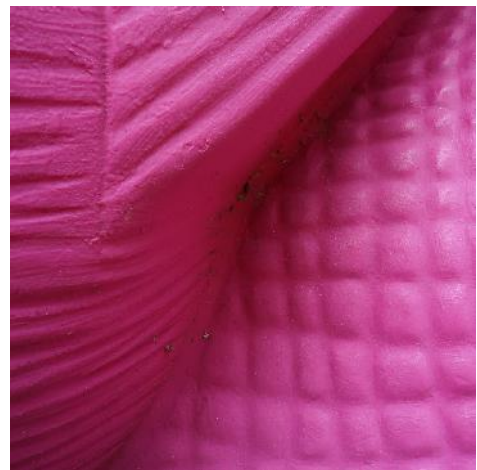
Figure 10. Soiling and debris collecting on underside of shell (photo by EverGreene, February 2021).
