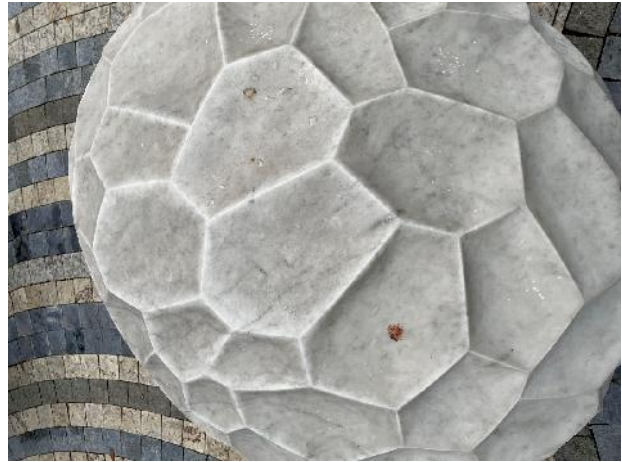
Figure 8. General soiling and guano, typical (photo by EverGreene, February 2021).
