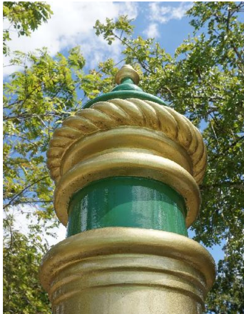
Figure 1. Capital of Triad of Venice with soiling on underside surfaces (photo by EverGreene, February 2021).
