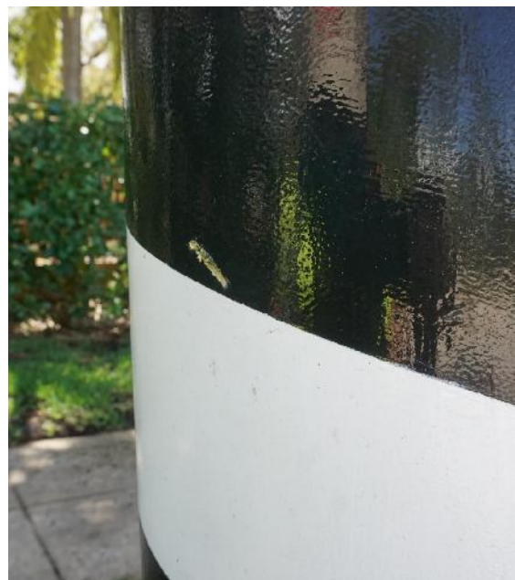
Figure 2: Gouge on the shaft of Pop Venice (photo by EverGreene, February 2021).
