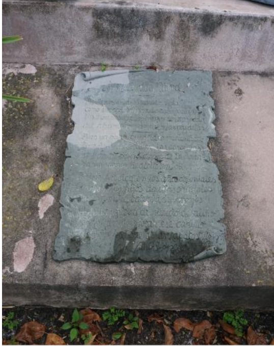
Figure 12. Concrete plaque (photo by EverGreene, February 2021).
