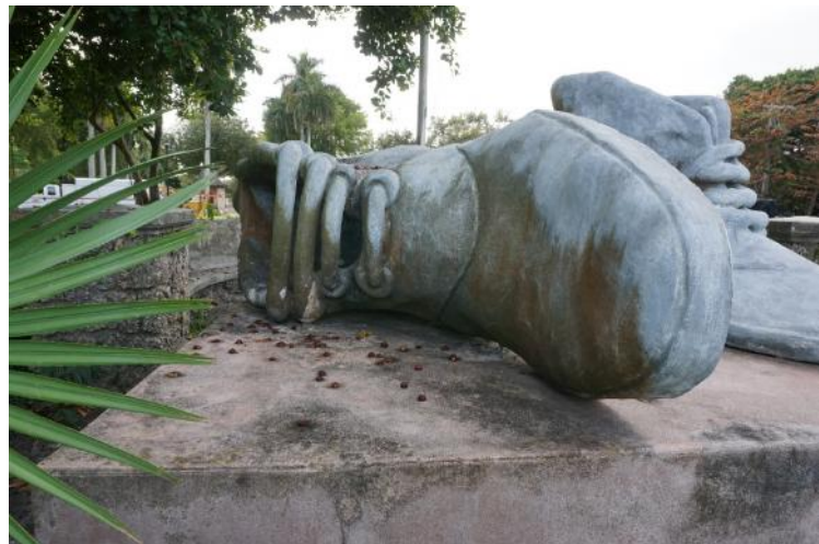
Figure 7. View of north shoe, biological growth and debris (photo by EverGreene, February 2021).
