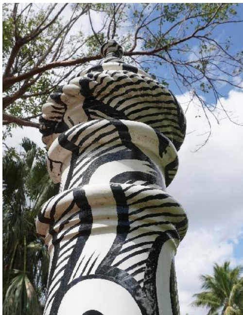
Figure 1. Soiling on undersides of the capital (photo by EverGreene, February 2021).
