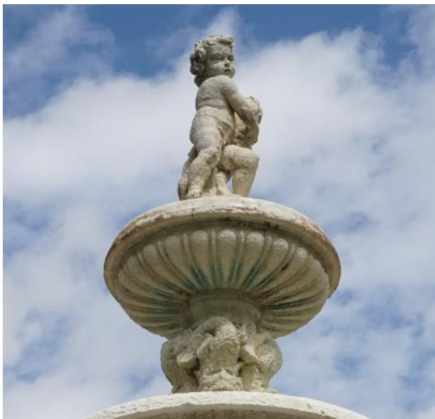
Figure 14. Copper staining on underside of top basin; cracks along entire edge of top basin; soiling and biological growth (photo by EverGreene, February 2021).
