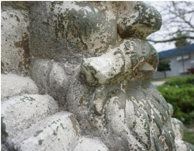
Figure 3. Previous repair on mustache (photo by EverGreene, February 2021).
