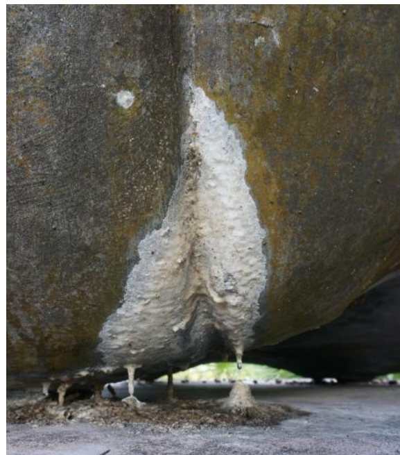
Figure 3. Extensive mineral accretions, typical stalactites and stalagmites forming on bottom of sculpture (photo by EverGreene, February 2020).
