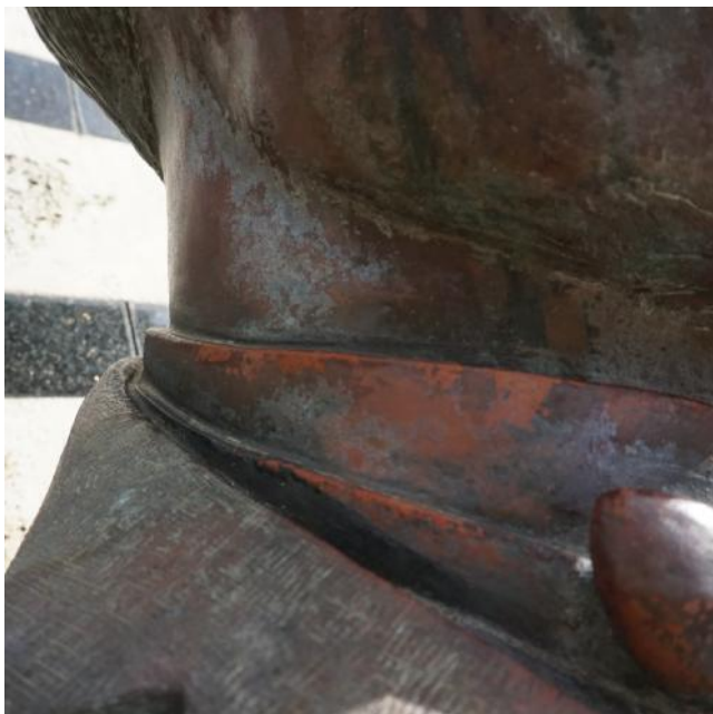
Figure 3. Coating failure and loss of patina, proper right side bust (photo by EverGreene, February 2021).
