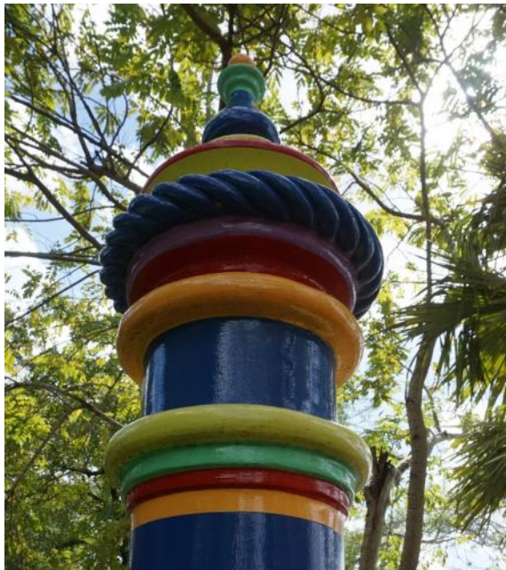
Figure 1. Soiling on underside of capital (photo by EverGreene, February 2021).
