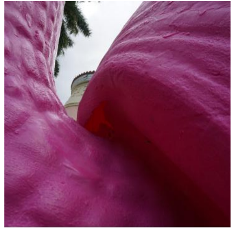
Figure 8. Large break on underside of the shell (photo by EverGreene, February 2021).
