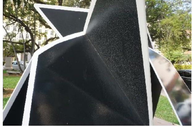
Figure 4. Soiling on surface that does not get washed with rain (photo by EverGreene, February 2021).
