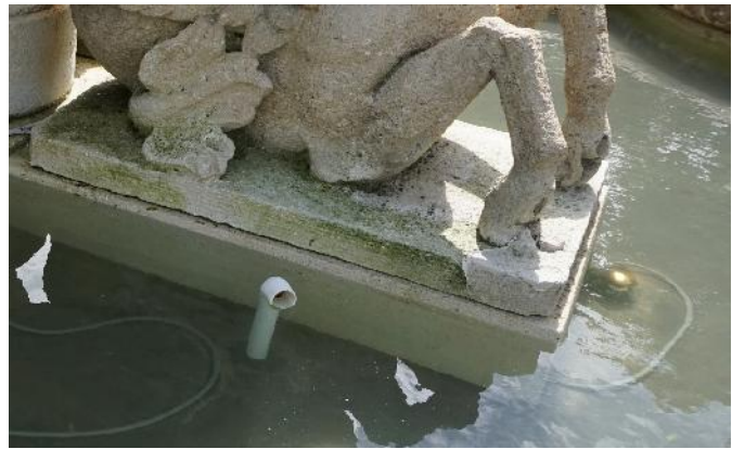
Figure 11. Previously repaired spall on west Pegasus; biological growth (photo by EverGreene, February 2021).
