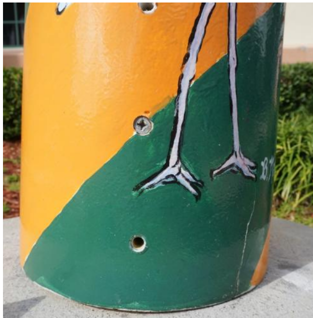
Figure 5. Missing fasteners (photo by EverGreene, February 2021).
