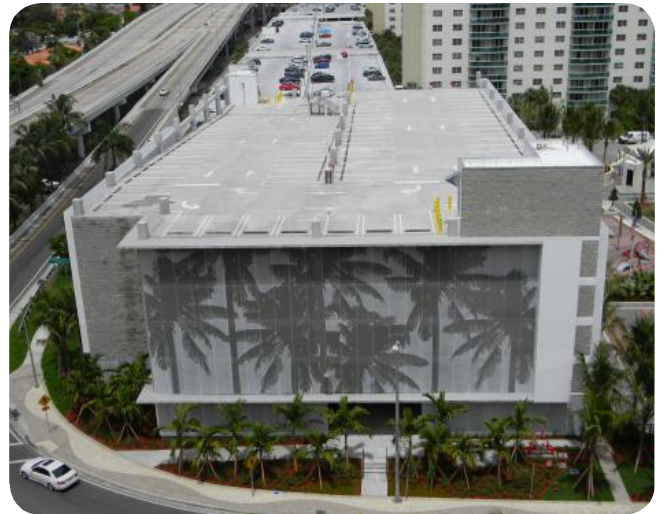
Heritage Park and Parking Garage, Sunny Isles Beach, FL
