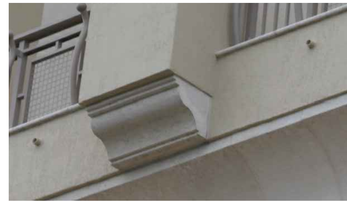
8 PRECAST CONCRETE BRACKETS GABLES PONCE
