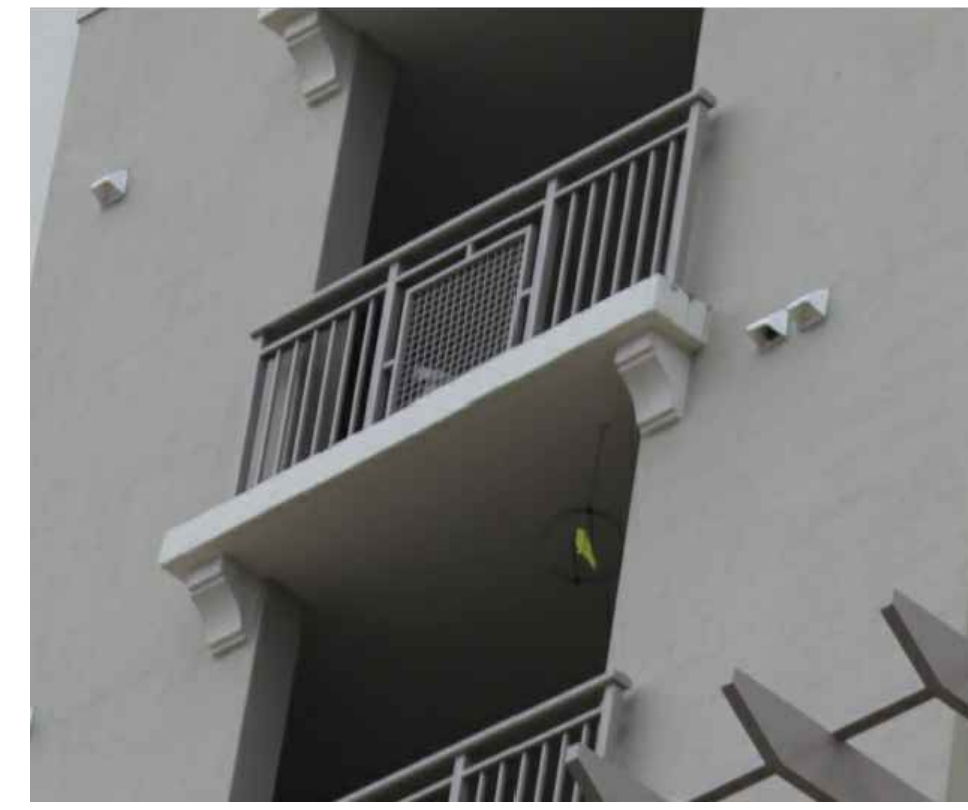
6 42" HIGH A.F.F. SAFEGUARD W/ BALCONIES GABLES PONCE
