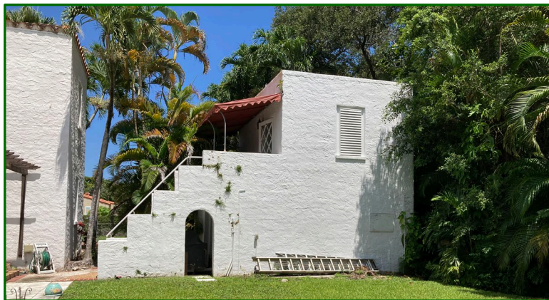
Figures 21: 1925 Garage Building Top: East Façade: 1962 Historic Photo [left]; 2023 [right] Center: North Façade, 2023 Bottom: West Façade, 2023
