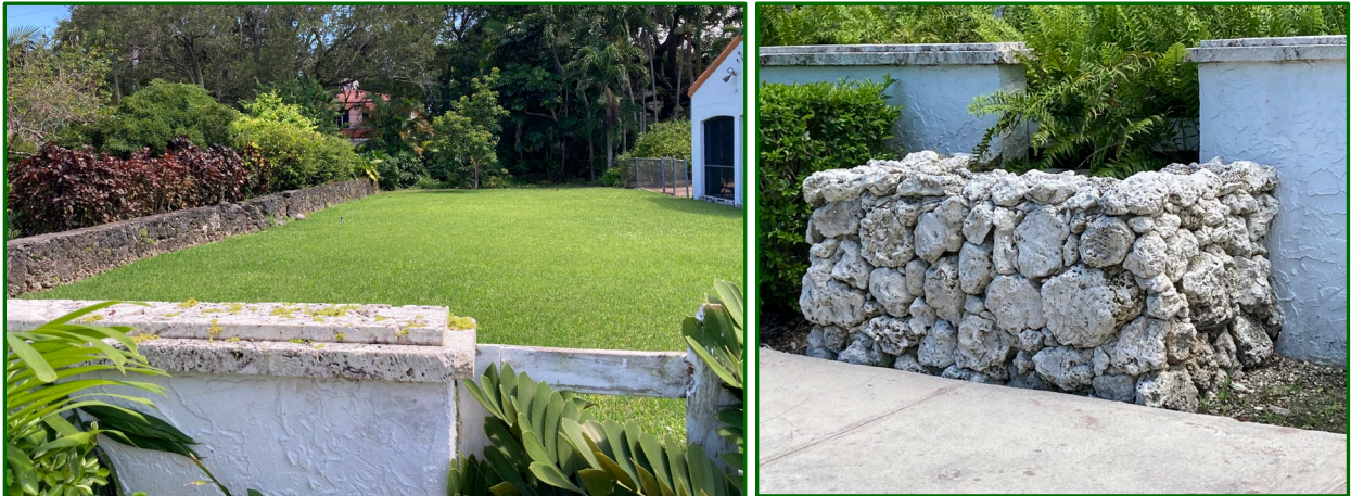
Figure 11: Perimeter Walls, 2023: East Wall [left]; Coral Rock Planter (typ.) [right]
