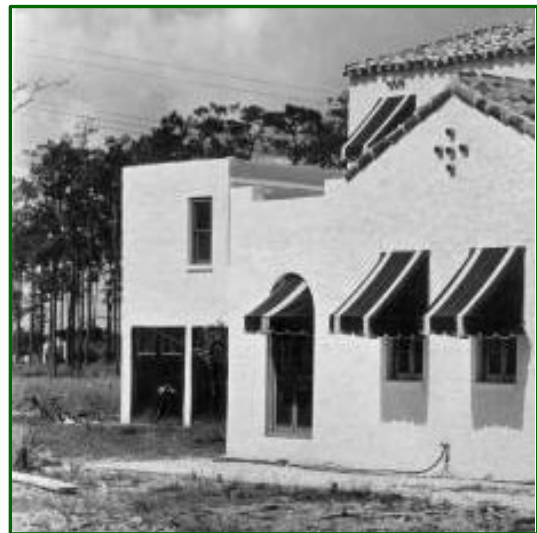
Figure 20: 1925 Garage Building Partial View East Façade with Vehicular Opening, August 1926
