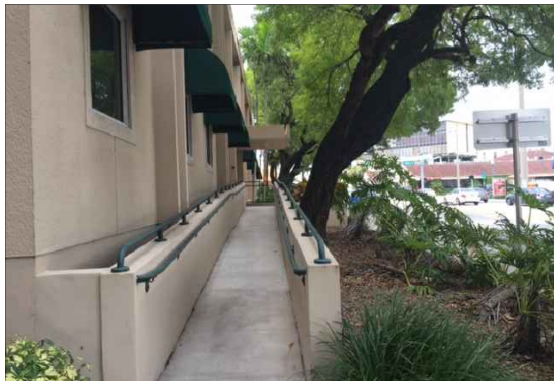
ANNEX BUILDING - EXISTING ADA RAMP
