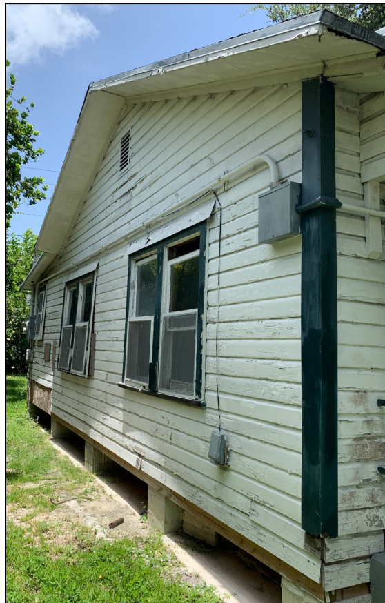
Figure 5: East Elevation Current Photo, July 2026
