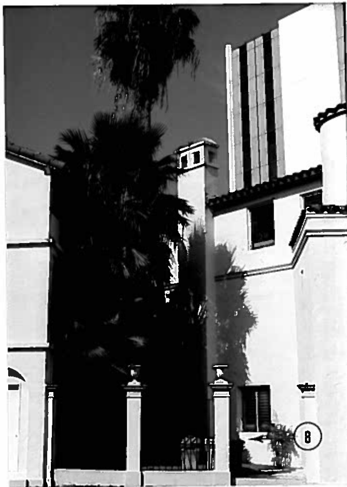
DETAIL, COURT AREA
