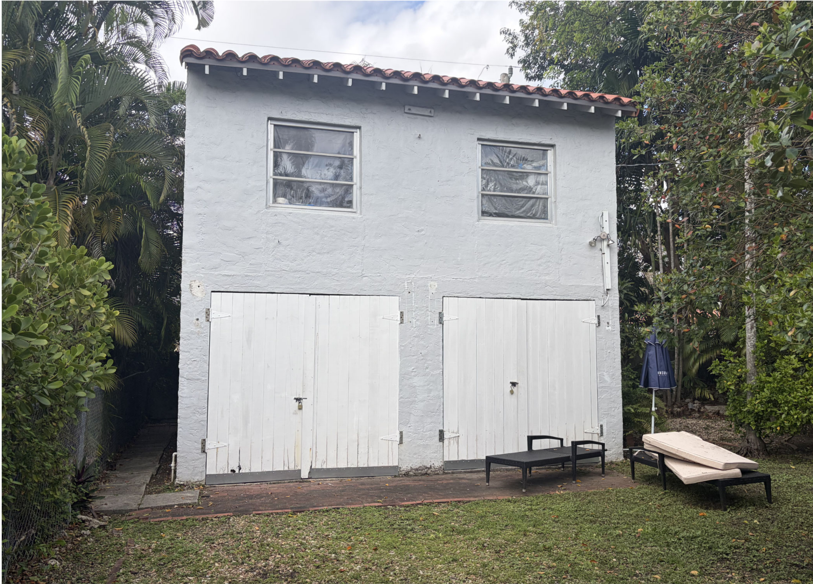
Existing carriage house
