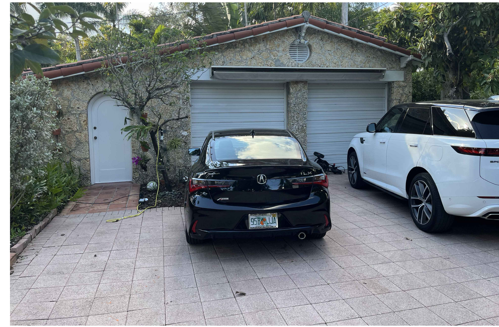
EXISTING GARAGE VIEW
