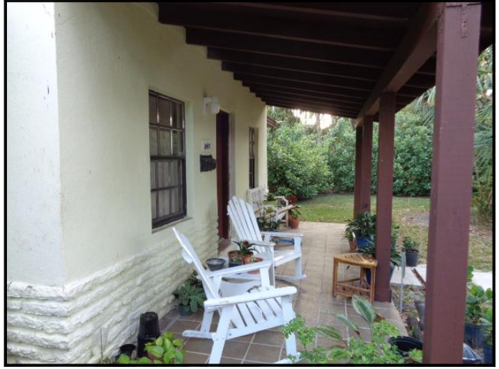
Covered Entry Porch
