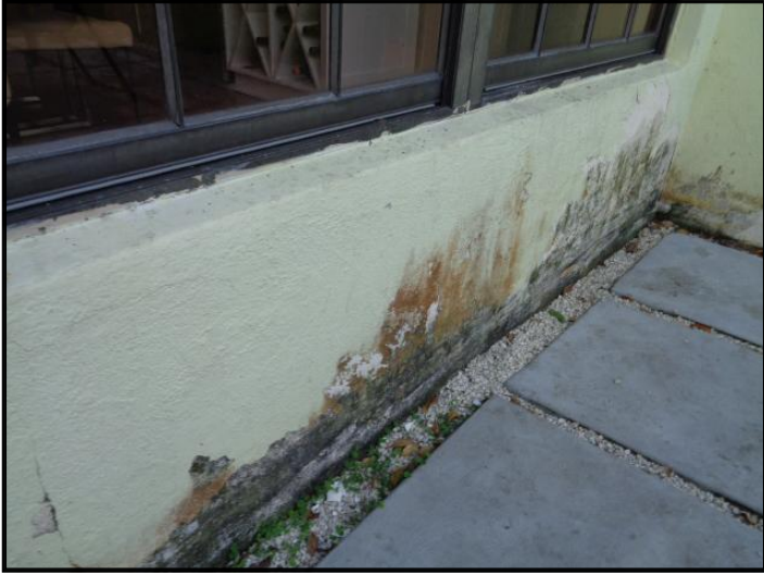
Exterior Wall Paint
