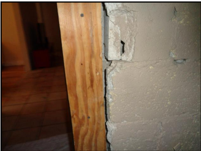
Gap Between Jamb and Wall
