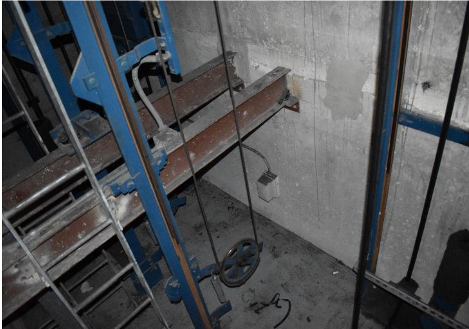
View of the elevator pit
