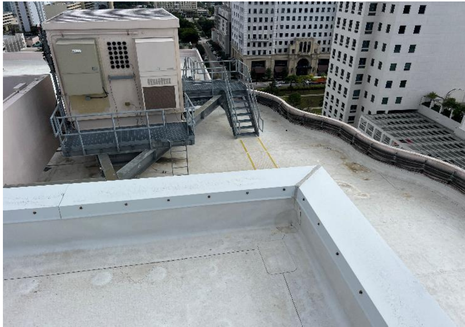
Overall view of the roof from the upper roof. Looking towards southeast.
