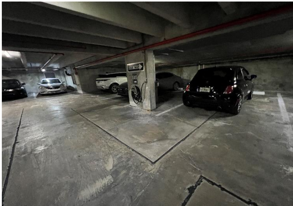
Typical view of the basement level, isolation joints between the SOG and top of spread and combined footings
