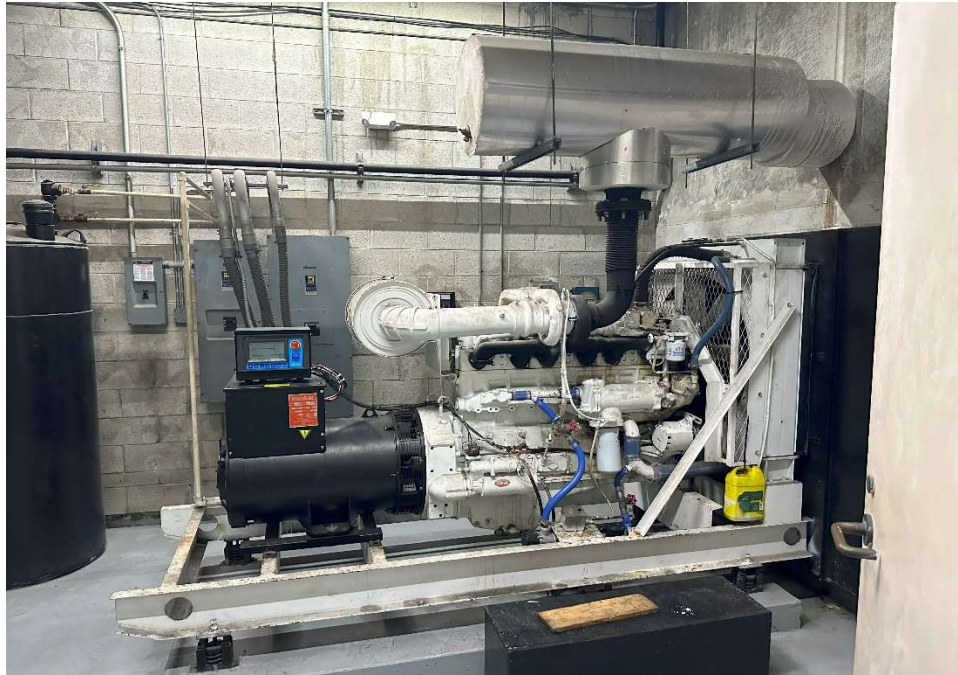
Generator Room Layout – 250KW Generator
