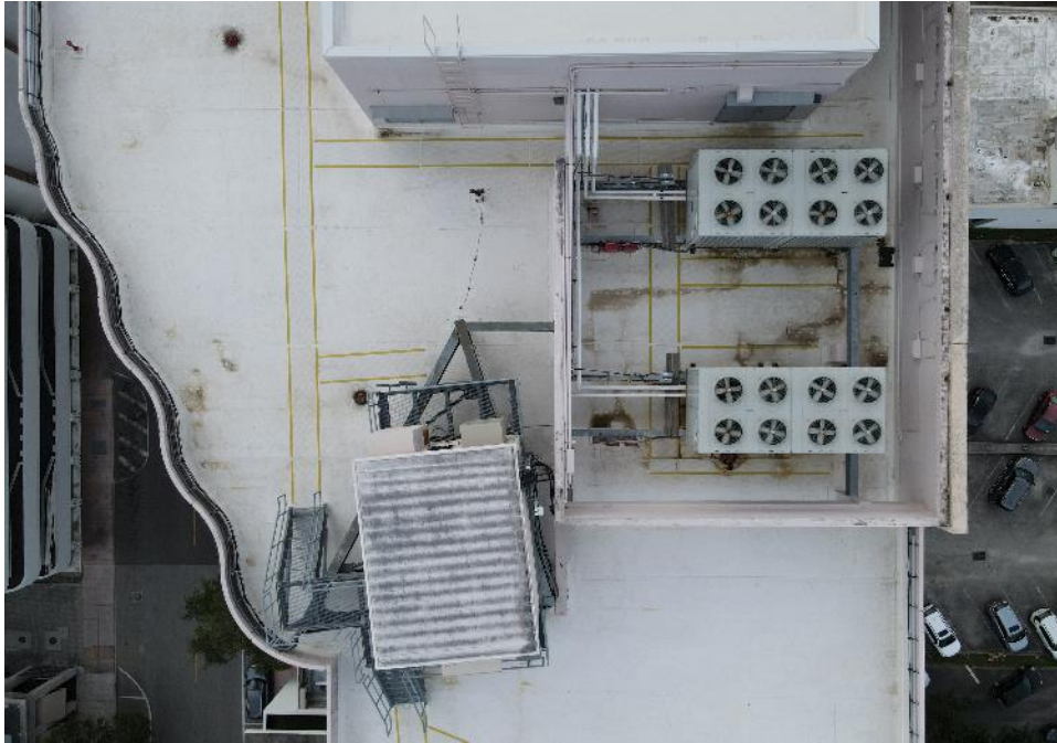
Close-up view of the roof
