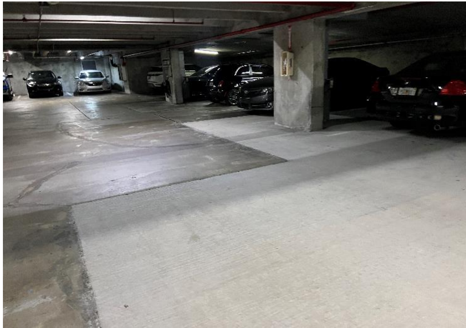
View of previous SOG repair at the basement level
