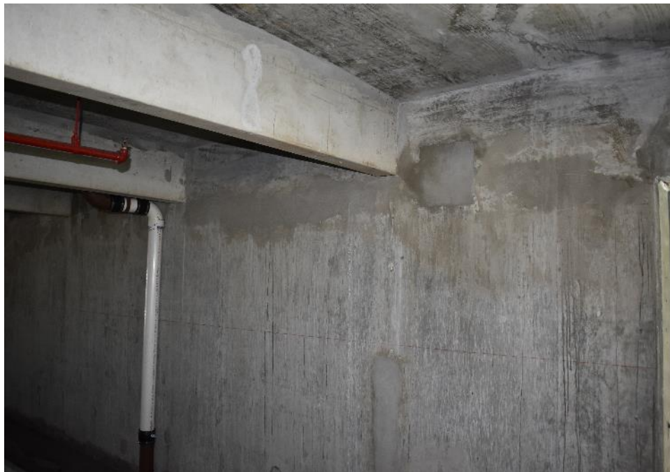
Typical repairs at the garage level
