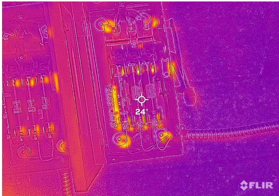
Item 33: Air Comp Disconnect at 24.0 Degrees Celsius (zero delta)
