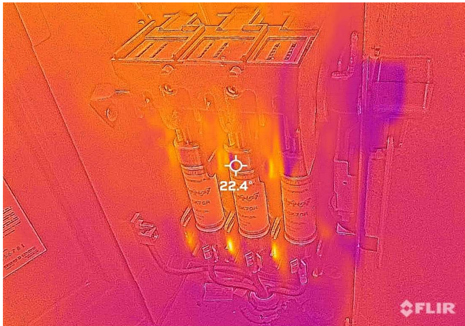
Item 69: Disconnect at 22.4 Degrees Celsius (zero delta)
