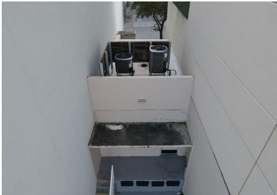
Small low-slope roof at the east elevation
