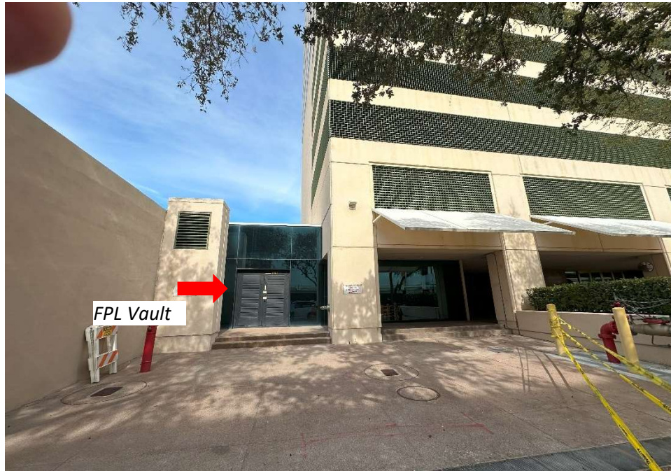
FPL Service: 3 Phase 277/480V, 4 Wire
