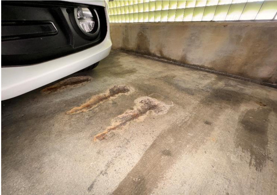
Typical spalling and exposed rebar at garage 3 rd level
