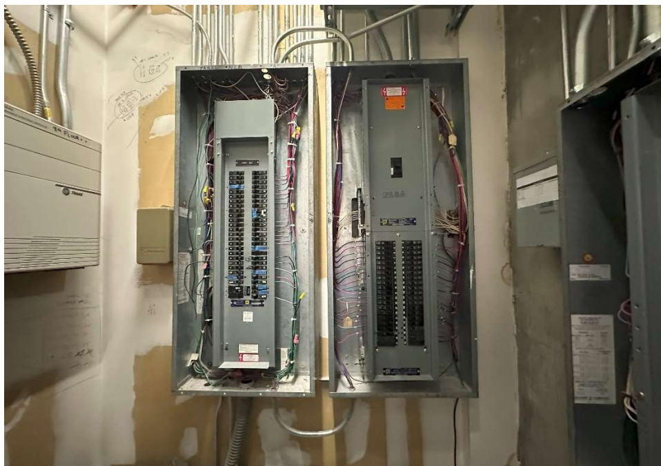
Panels NL8 and NL8A Opened -
