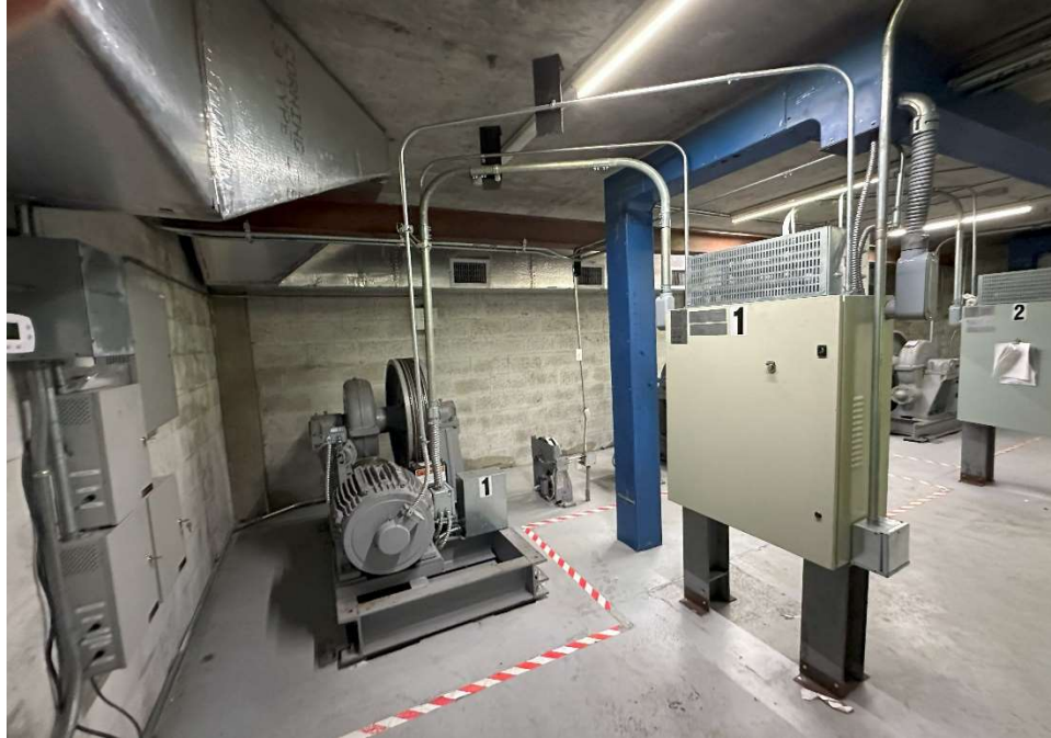
Elevator Machine Room – Elevators 1,2 & 3 – Upper Roof -
