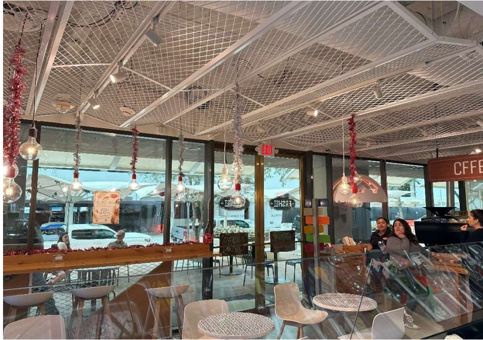
Restaurant Emergency/Exit Lights –
