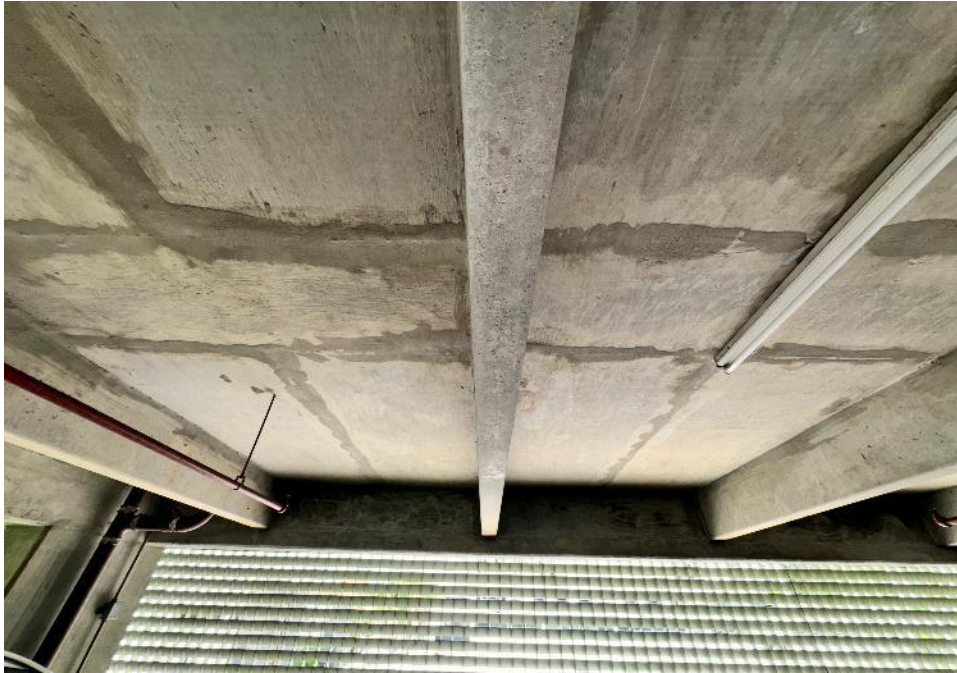
Typical overhead repairs at the garage levels
