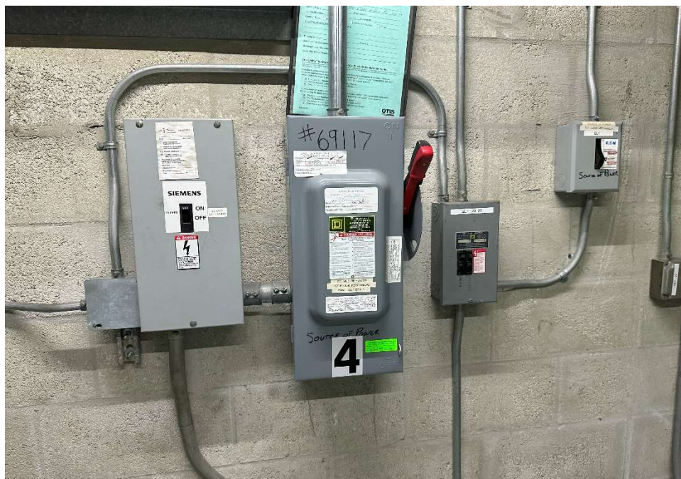
Elevator 4 Disconnects -
