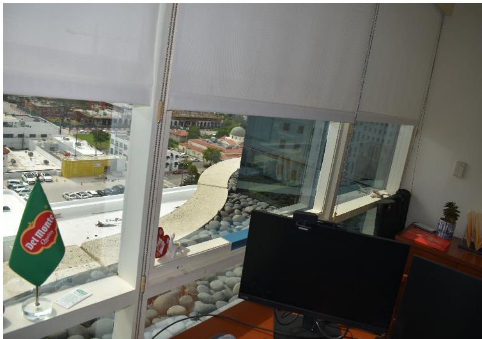
View of the interior side of the windows
