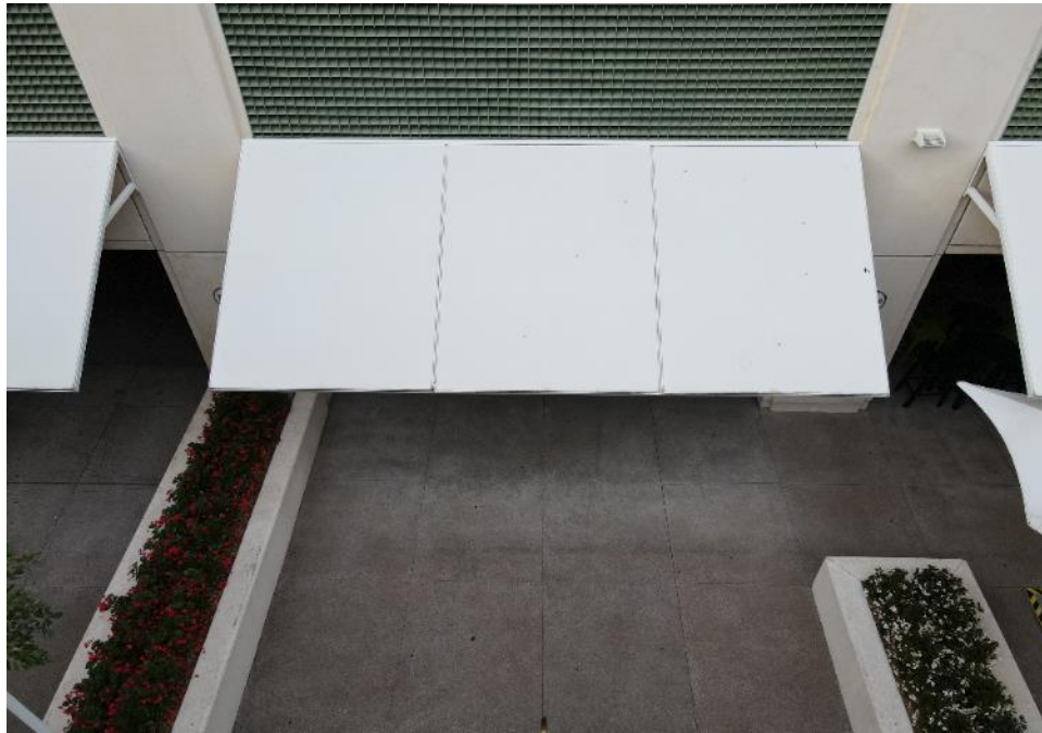
Typical awnings at the south elevation
