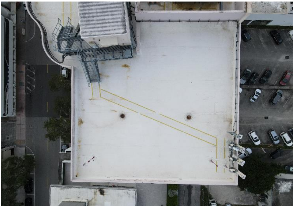
Close-up view of the roof at the east side
