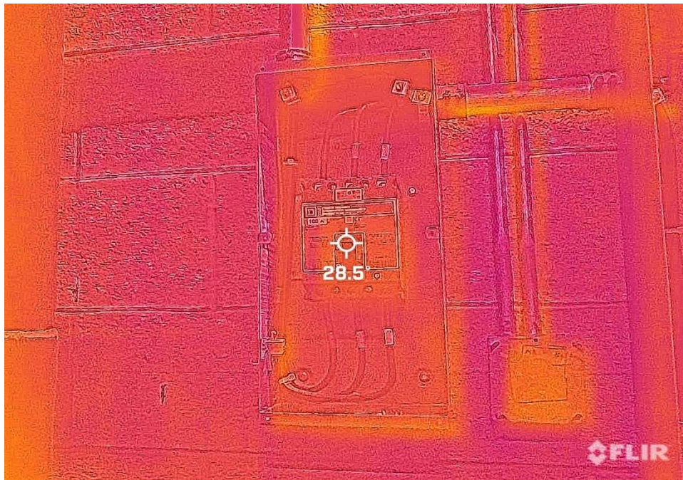
Item 18: Elev Disconnect at 28.5 Degrees Celsius (delta 3.5C)
