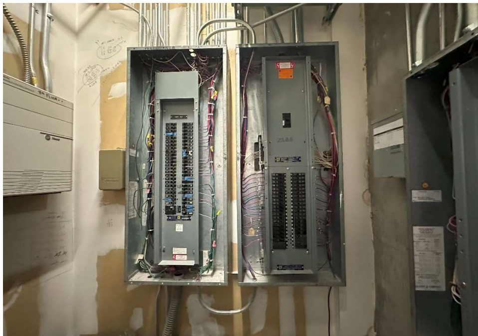
Panels NL8 and NL8A Opened -
