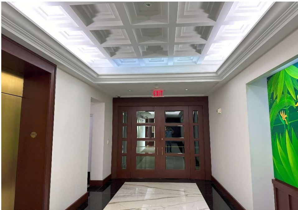
Means of Egress Lighting – Exit Lighting -
