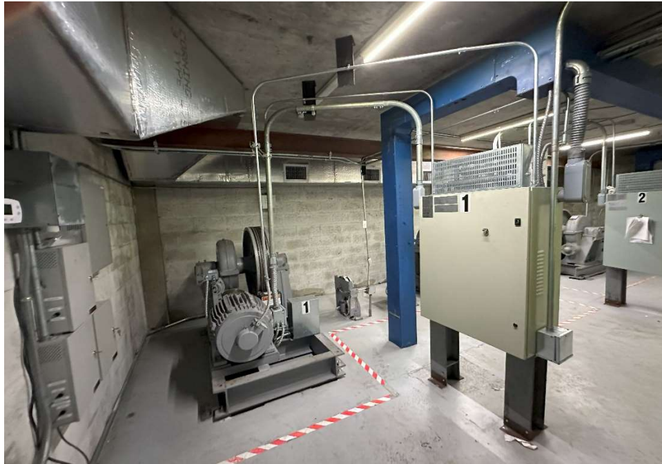
Elevator Machine Room – Elevators 1,2 & 3 – Upper Roof -
