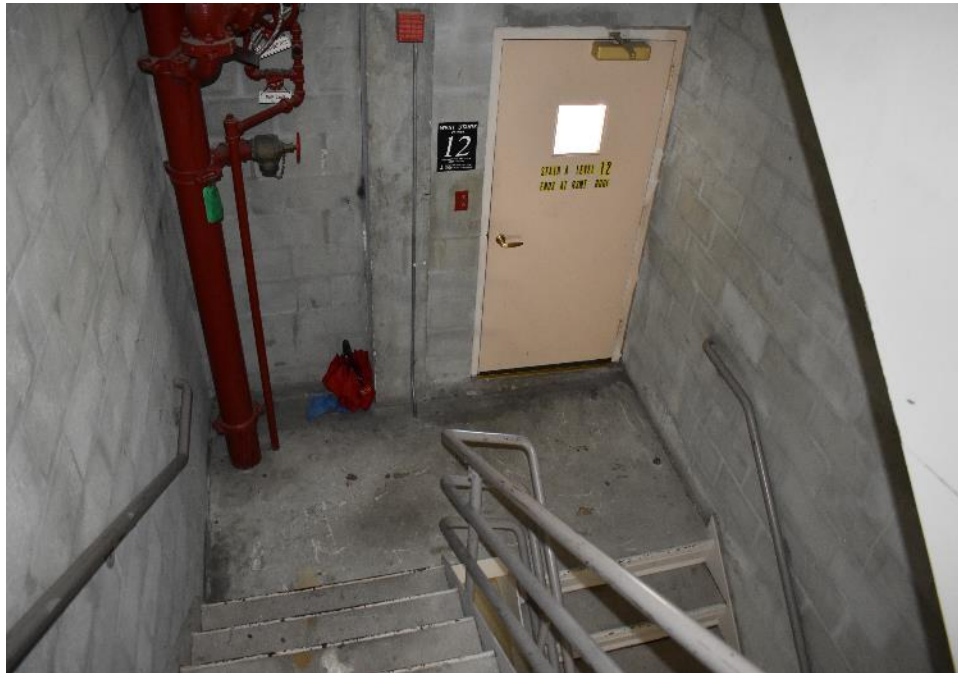
Typical view of the stairwell
