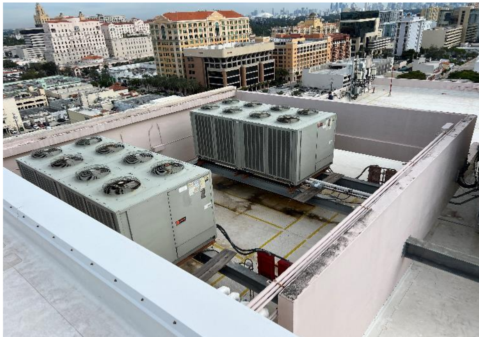
Overall view of the roof from the upper roof. Looking towards northeast.
