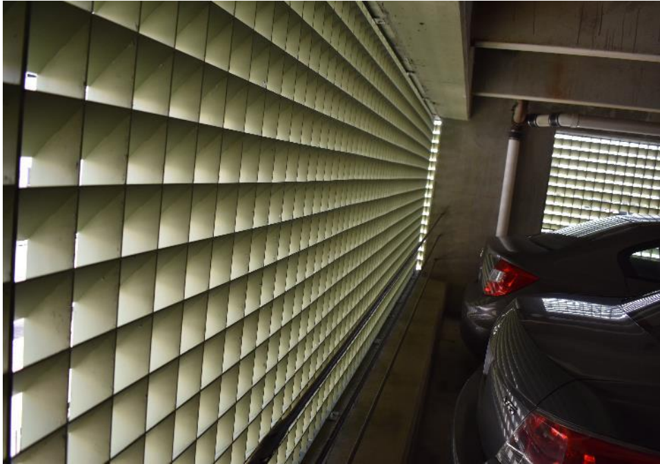
Typical louvers at the garage level
