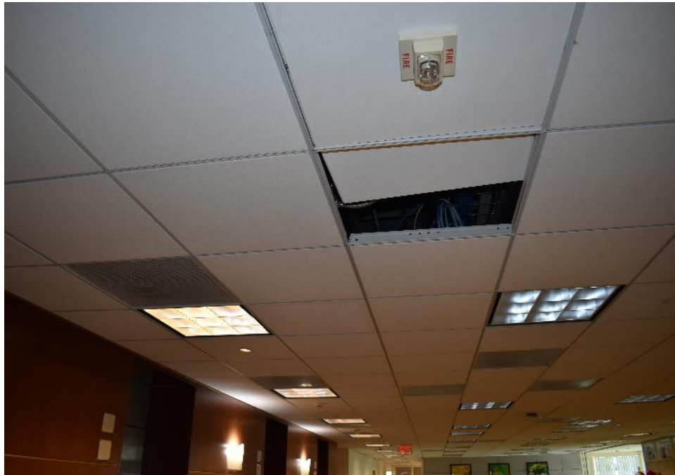
Typical acoustical tile ceiling at the office levels
