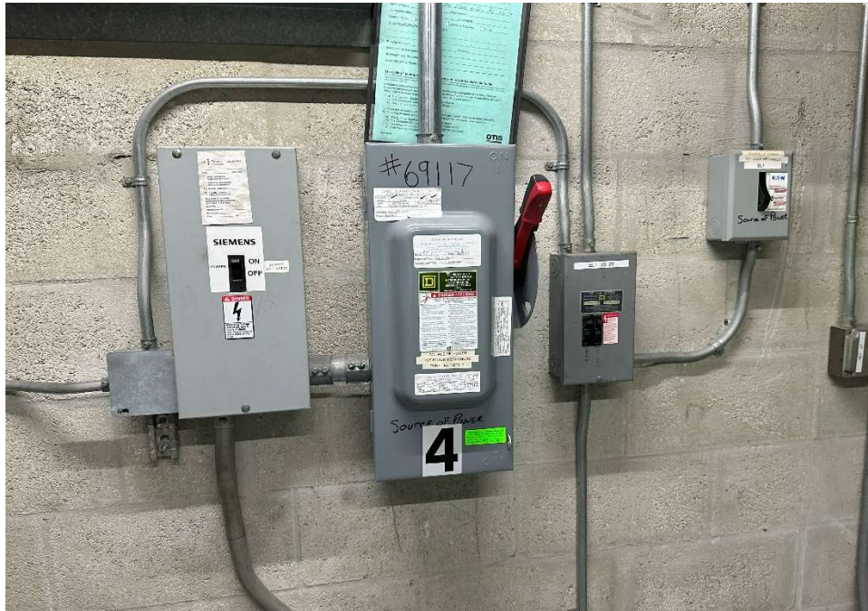
Elevator 4 Disconnects -
