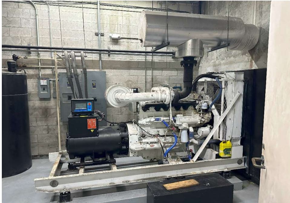
Generator Room Layout – 250KW Generator
