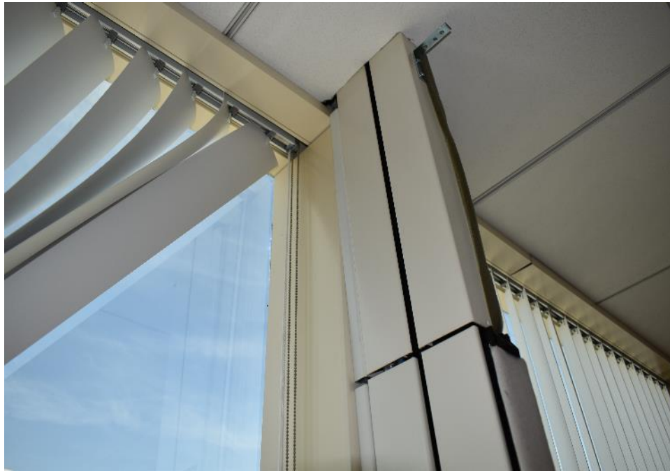
Typical partition to window frame
