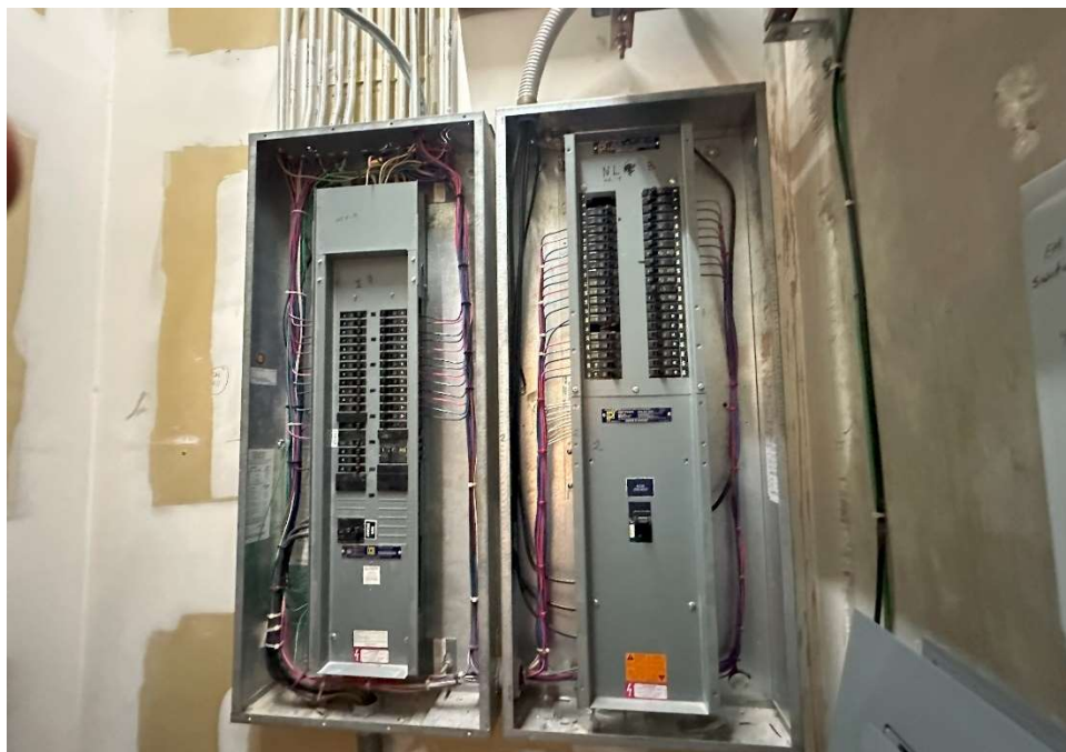
Panels NL9A and NL9B Opened -
