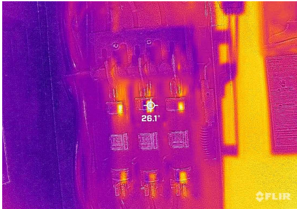
Item 23: Elev Disconnect 2 at 26.1 Degrees Celsius (delta 4.1C)
