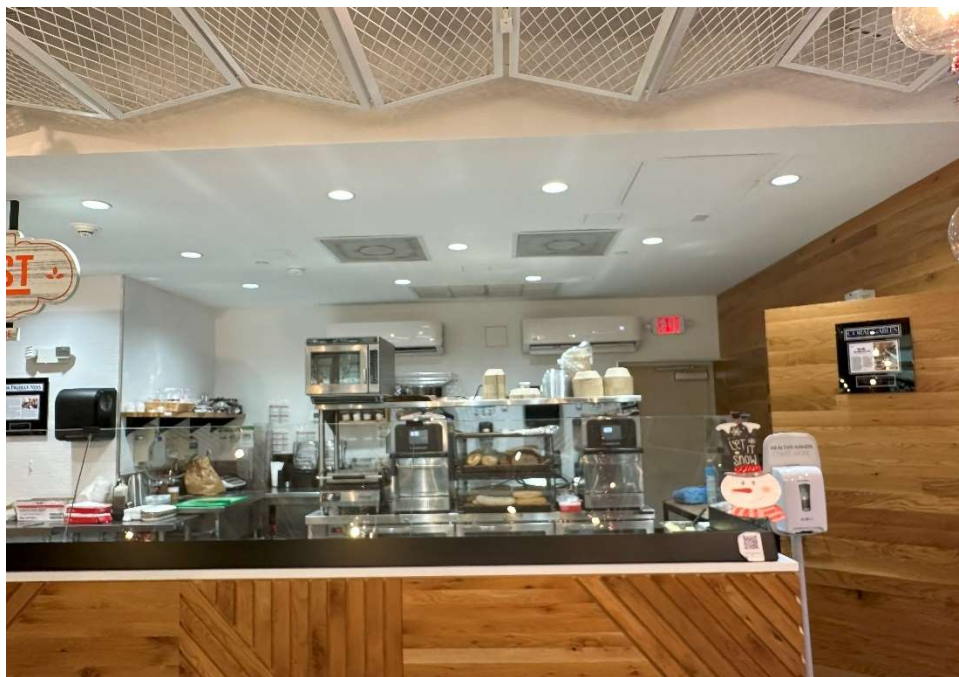
Restaurant Emergency/Exit Lights -
