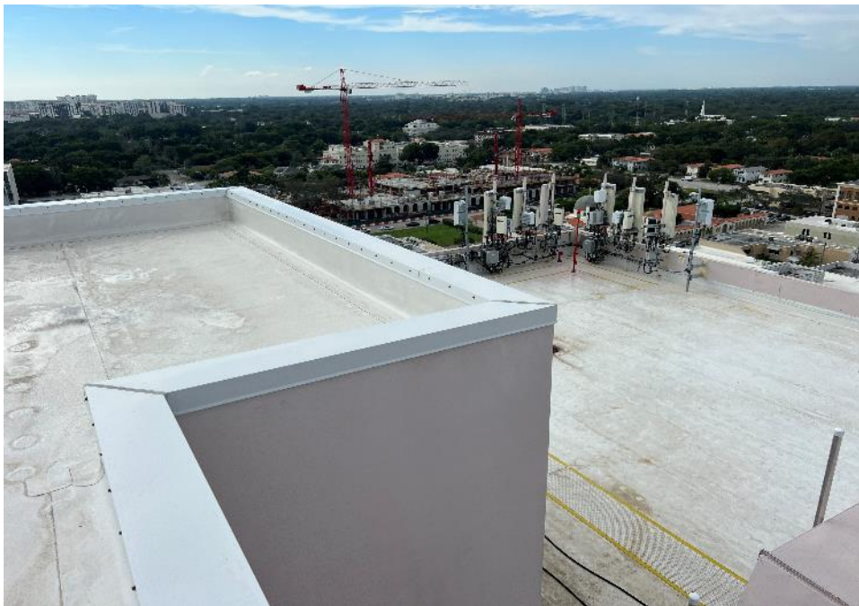
Overall view of the roof from the upper roof. Looking towards southwest.
