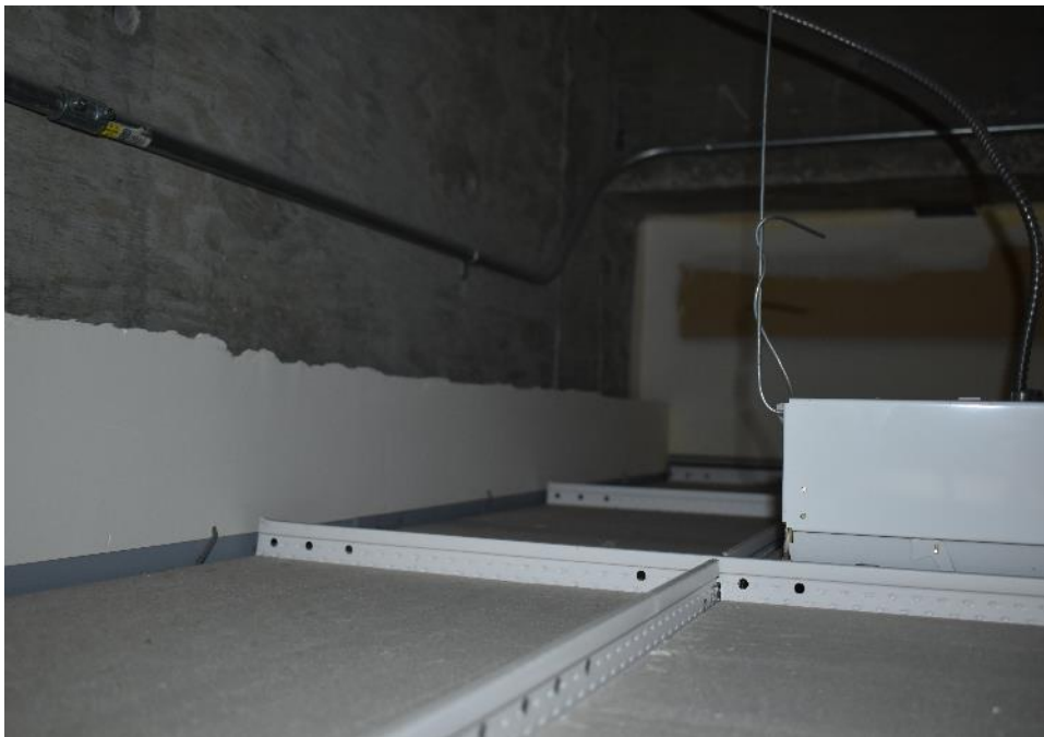
View of the structure above the acoustical tile ceiling
