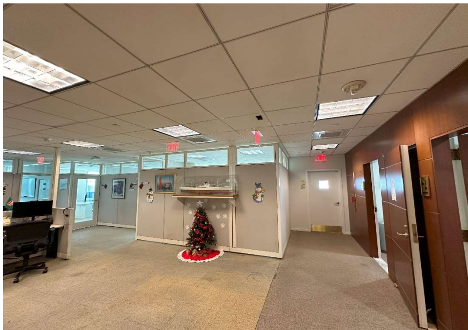
Means of Egress Lighting – Exit Lighting -
