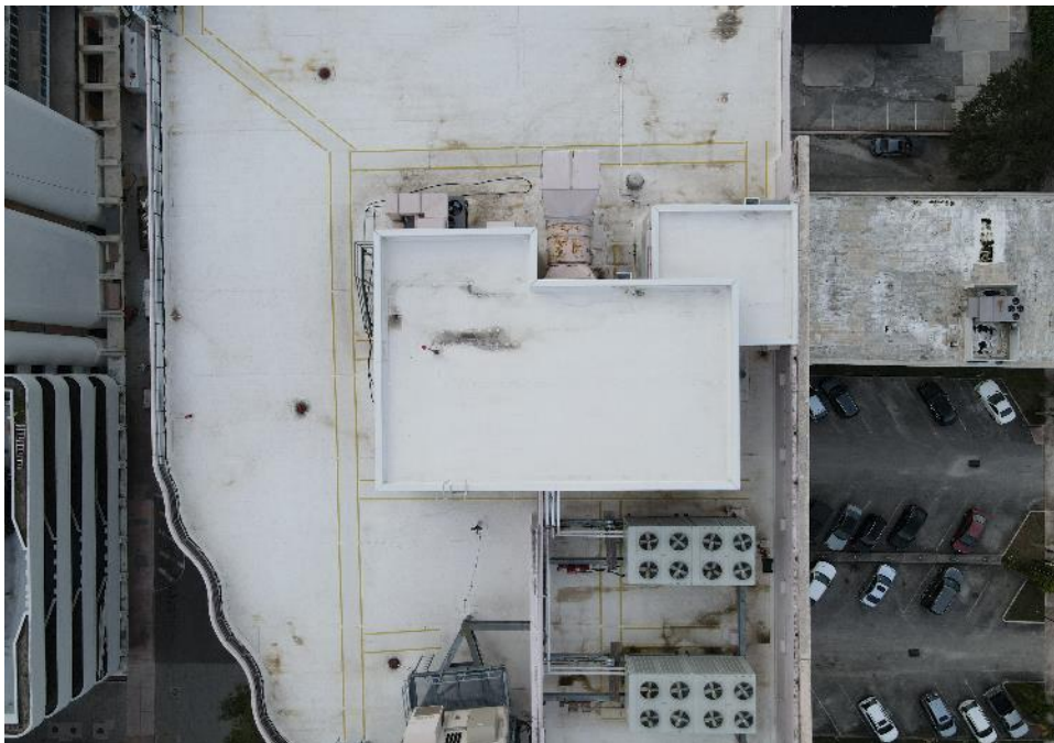
Aerial view of the roof
