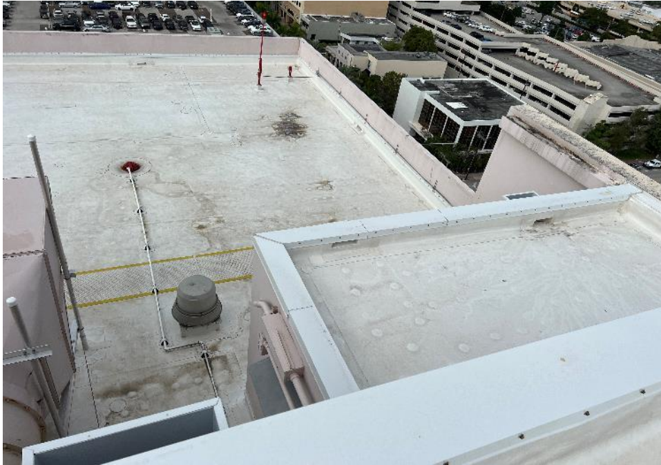
Overall view of the roof from the upper roof. Looking towards northwest.
