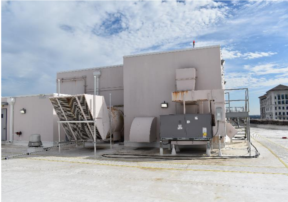
Roof equipment rooms and upper roof
