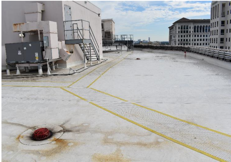
Overall view of the roof and drains
