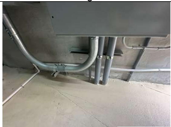
11. Service conduit/raceways
