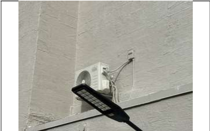
27. Wiring to mechanical equipment
