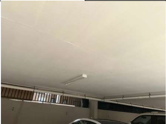
19. Building egress illumination
