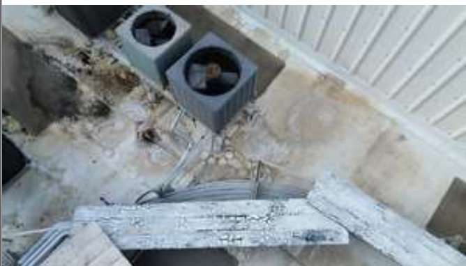
27. Wiring to mechanical equipment
