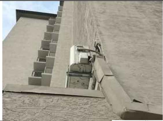
27. Wiring to mechanical equipment
