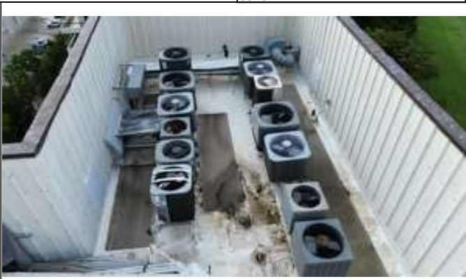
27. Wiring to mechanical equipment
