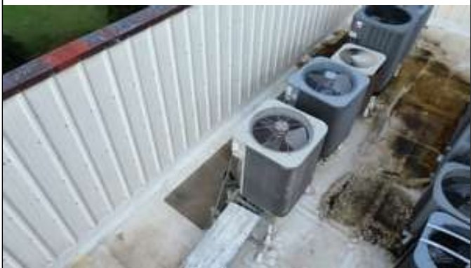
27. Wiring to mechanical equipment
