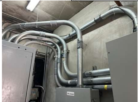
11. Service conduit/raceways
