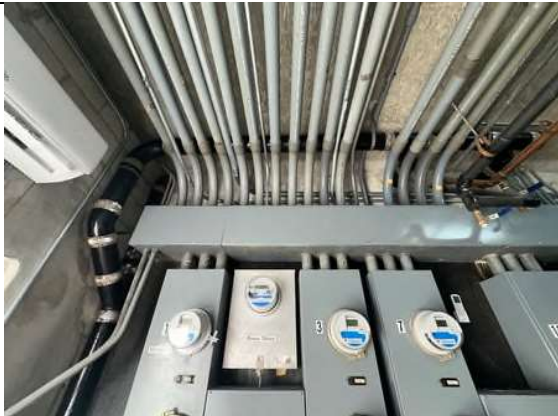
11. Service conduit/raceways
