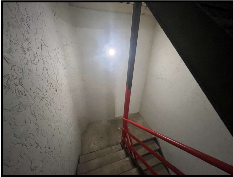
Photograph #174 The stairway landing properly illuminated.
