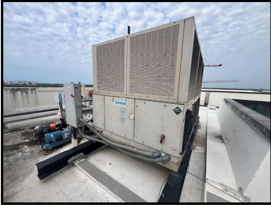
Photograph #155 AC Roof Area properly installed and good standing.
