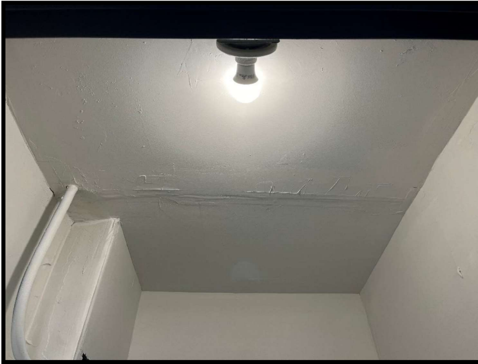
Photograph #110 Electrical room properly lit.
