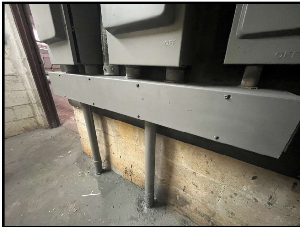
Photograph #72 Gutter in good condition.
