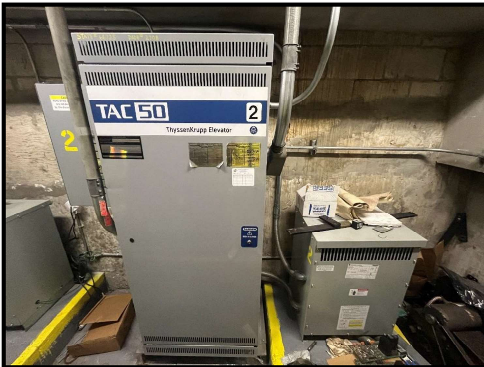
Photograph #44 Elevator Machine 2 properly identified. The label shall be of sufficient durability to withstand the environment involved and shall not be handwritten. NEC 210.5 C (1) (b). In the 2020 NEC, Section 705.10, Section 11.12.2.1.5 in NFPA 1.
