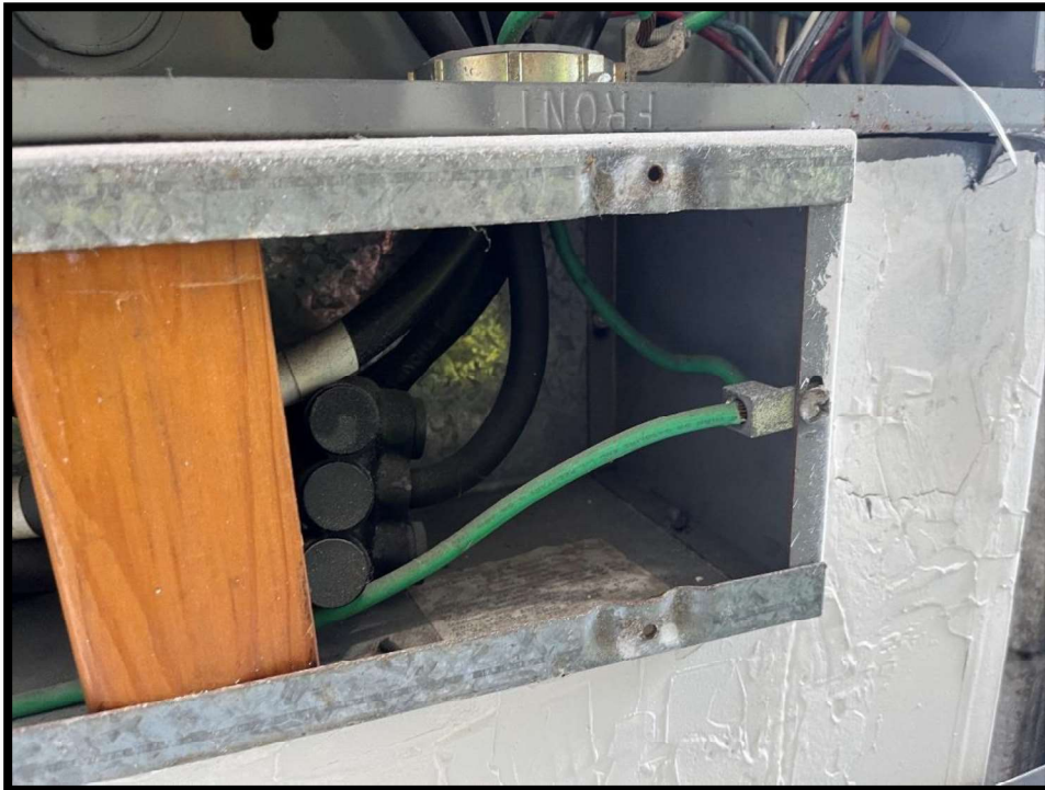
Photograph #96 The ground of the Gutter is properly installed.
