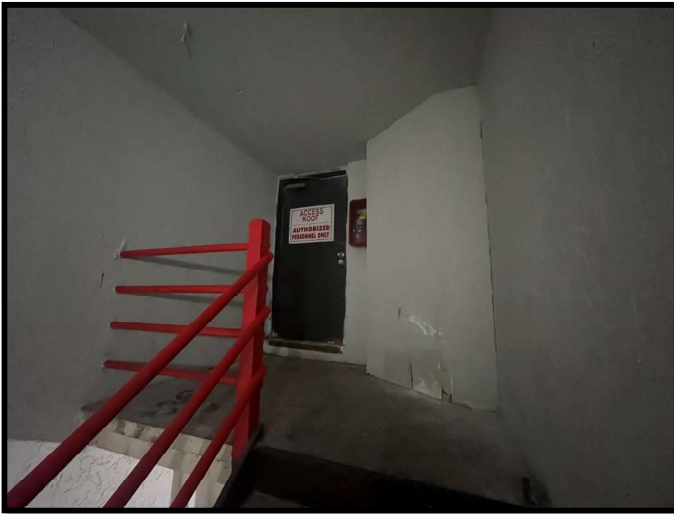
Photograph #164 The stairway landing properly illuminated.
