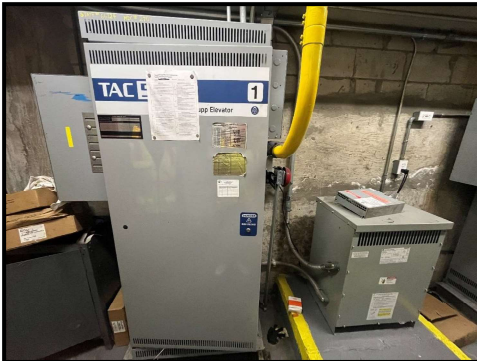
Photograph #40 Elevator Machine 1 properly identified.
