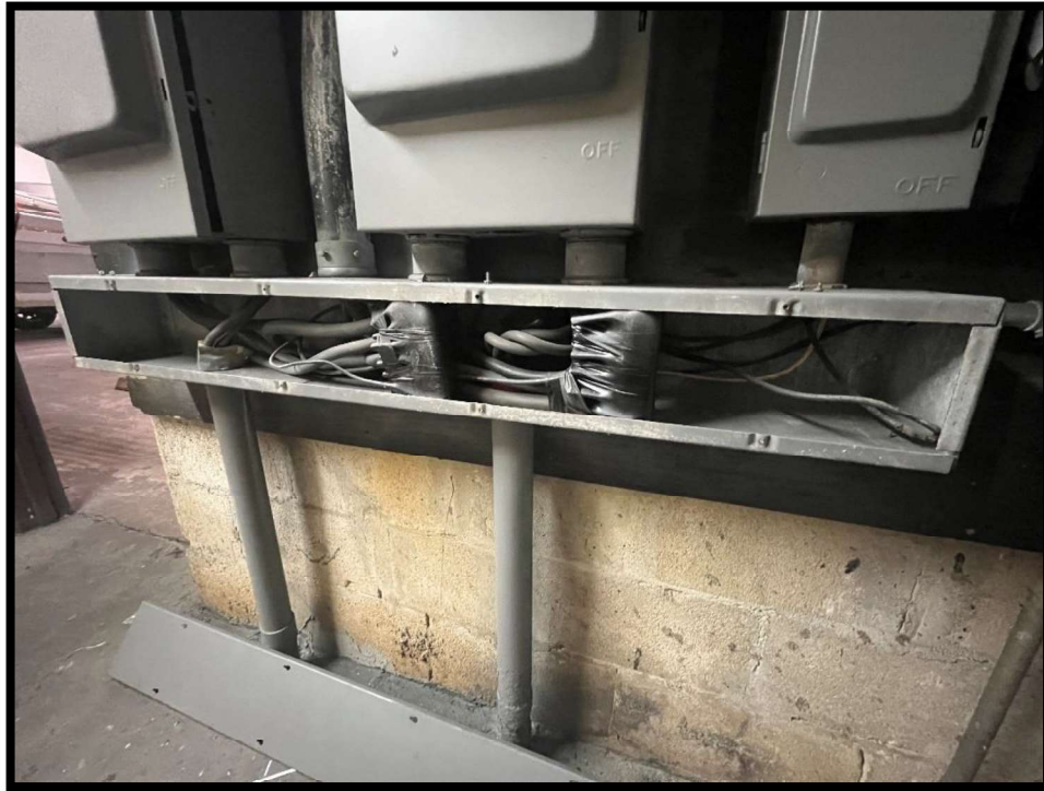
Photograph #73 Gutter properly installed and good standing.
