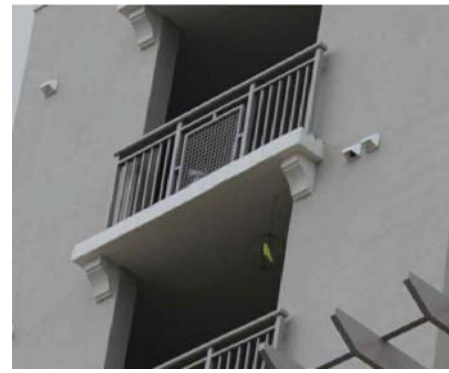
6 42" HIGH A.F.F. SAFEGUARD W/ BALCONIES GABLES PONCE
